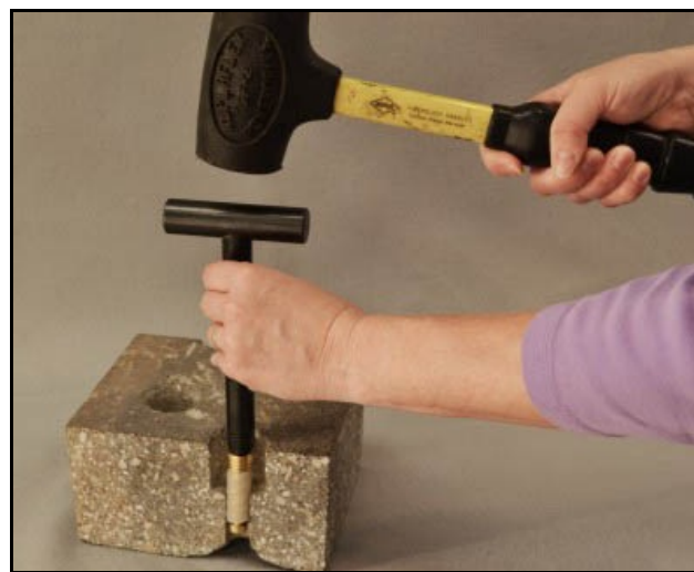
Figure 2. Flush-Mount Installation Process.
