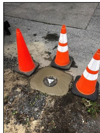
Photo of RW-5 curb box replacement following pouring of concrete.
