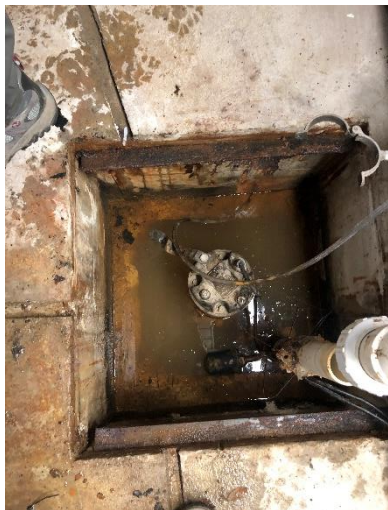
Photo looking down into sump and operating pump float mechanism during April 2021 inspection.
