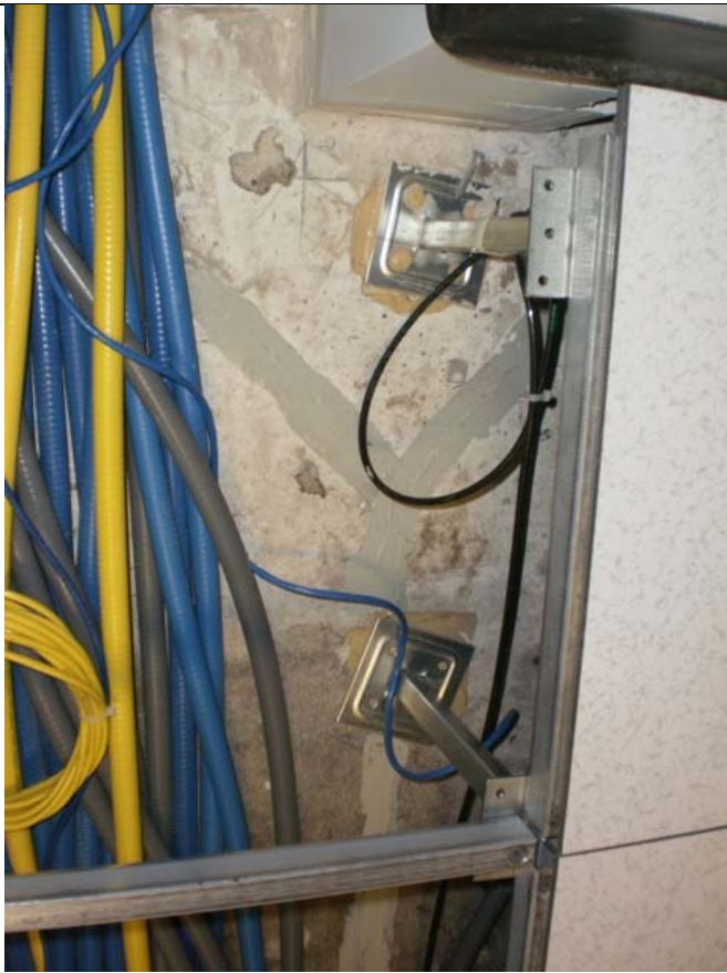
After sealing, expansion joints in the concrete floor slab below the raised floor in the VoltDelta server space.
