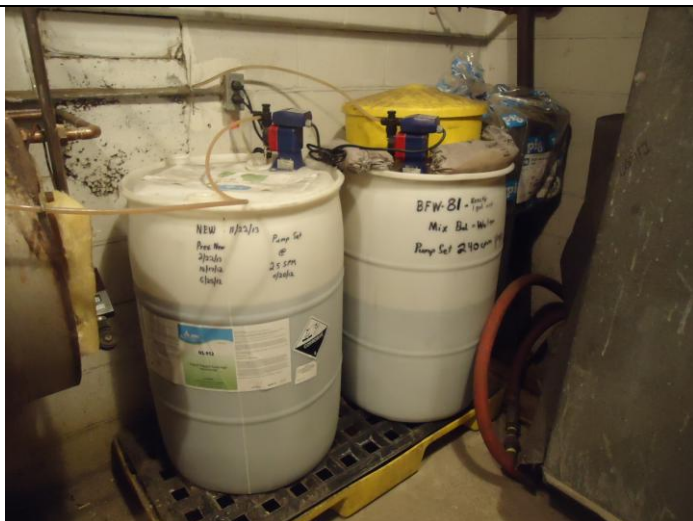
Liquid oxygen scavenger in Building 1
