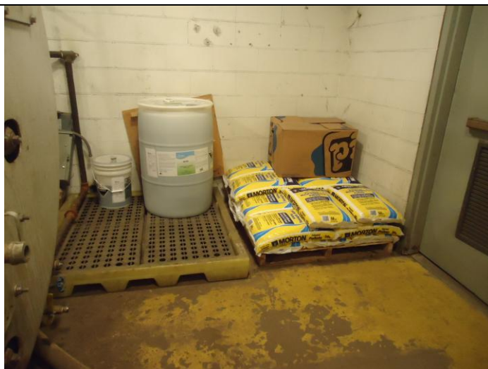
Liquid oxygen scavenger and salt in Building 1
