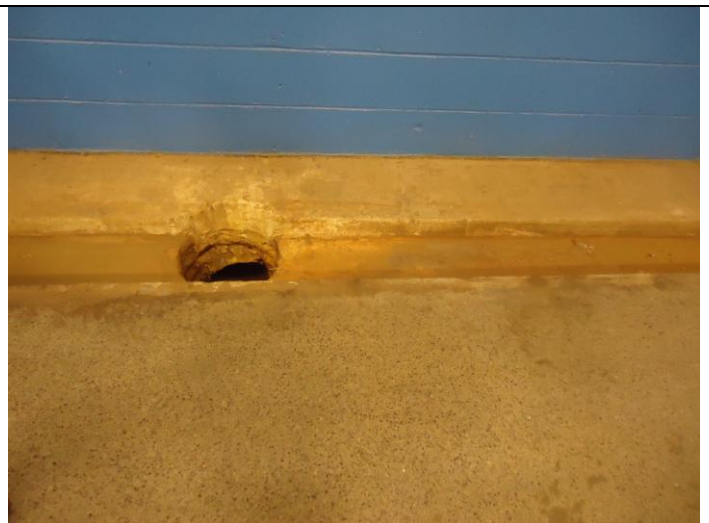
Plugged trench drain in Building 1
