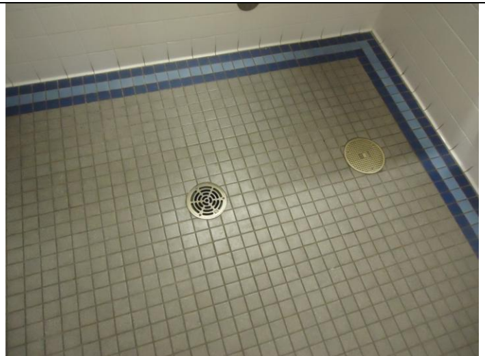
Floor Drain in Bathroom in Building 1
