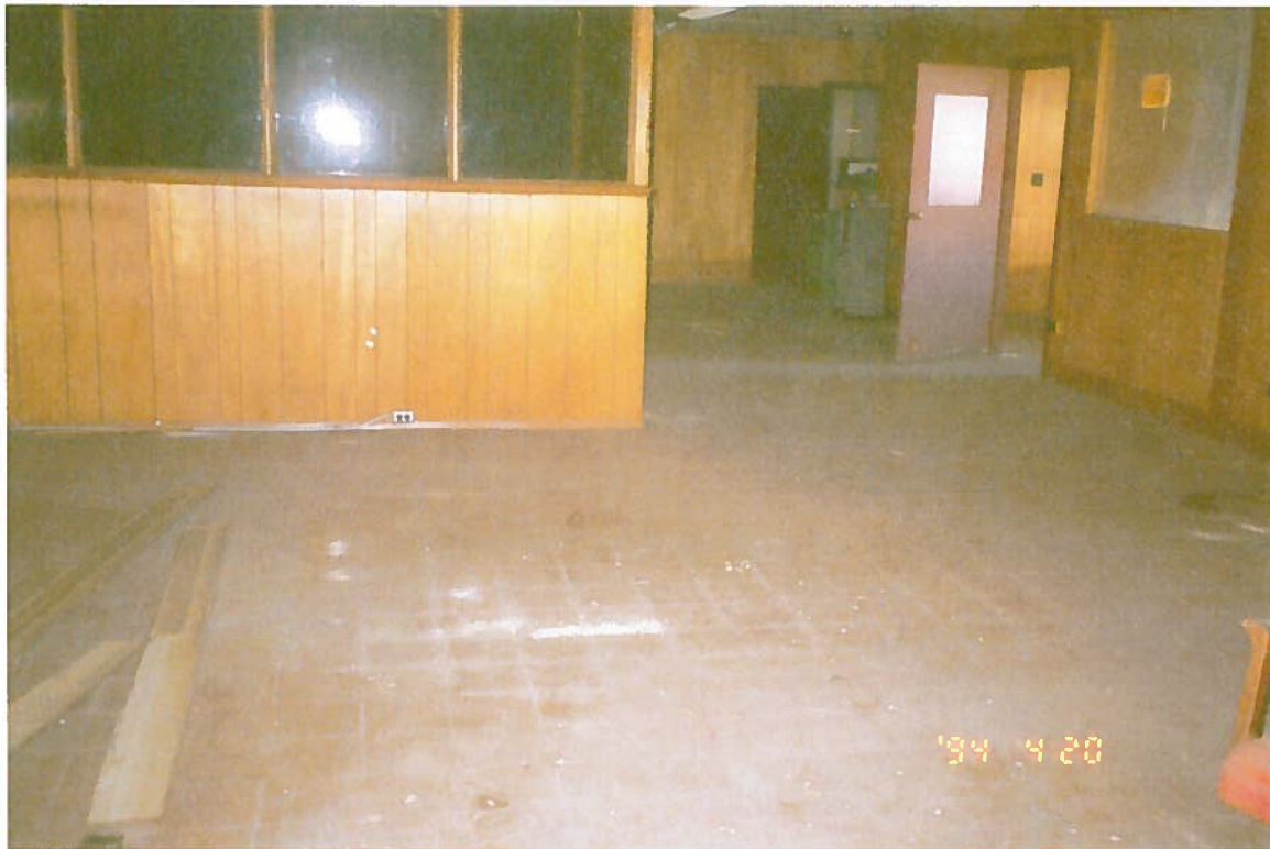
Photo No. 19. Second Floor 9 X 9 Floor Tile.
