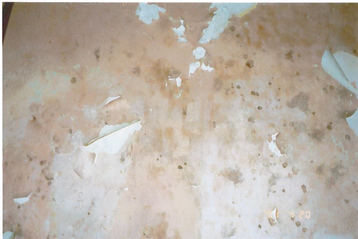
Photo No. 17. Stairway (Peeling Paint).
