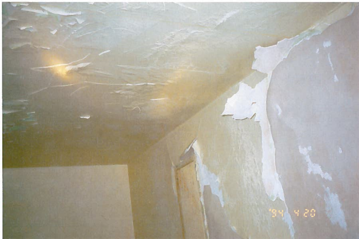
Photo No. 16. Second Floor Bathroom (Peeling Paint).
