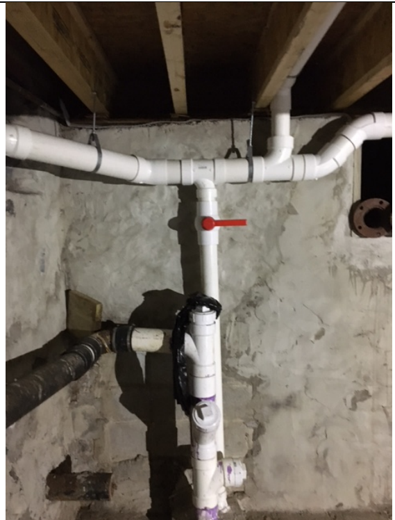
SSDS riser and valve from basement area intake pipe.
