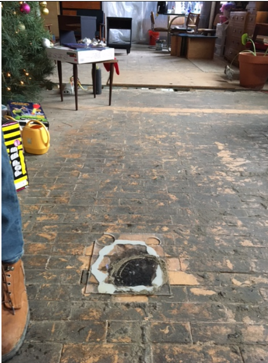
Test extraction hole, north side of Building E through brick floor slab.
