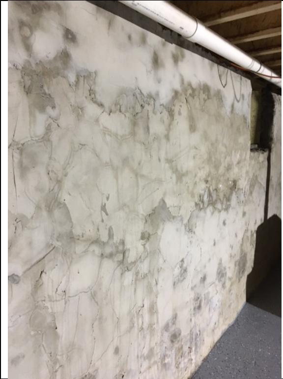
Basement wall, west side. Newly pointed.
