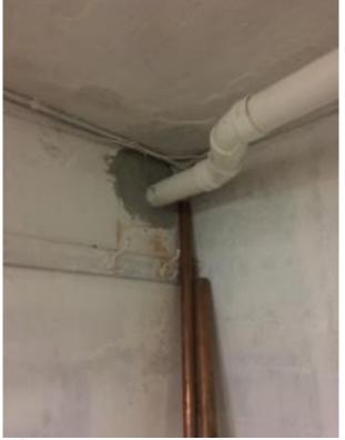
**DP-03** – Horizontal depressurization point extending below the western portion of the Site building where no basement is present.
