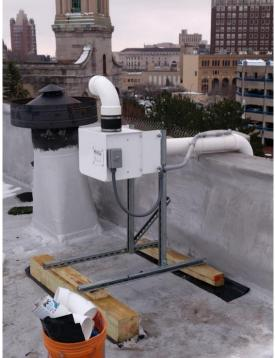
Festa Radon Technologies Company FRT Force fan, located on the roof of the Site building.
