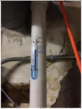
U-tube manometer on one of the depressurization points.
