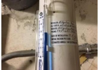
U-tube manometer and label on one of the depressurization points
