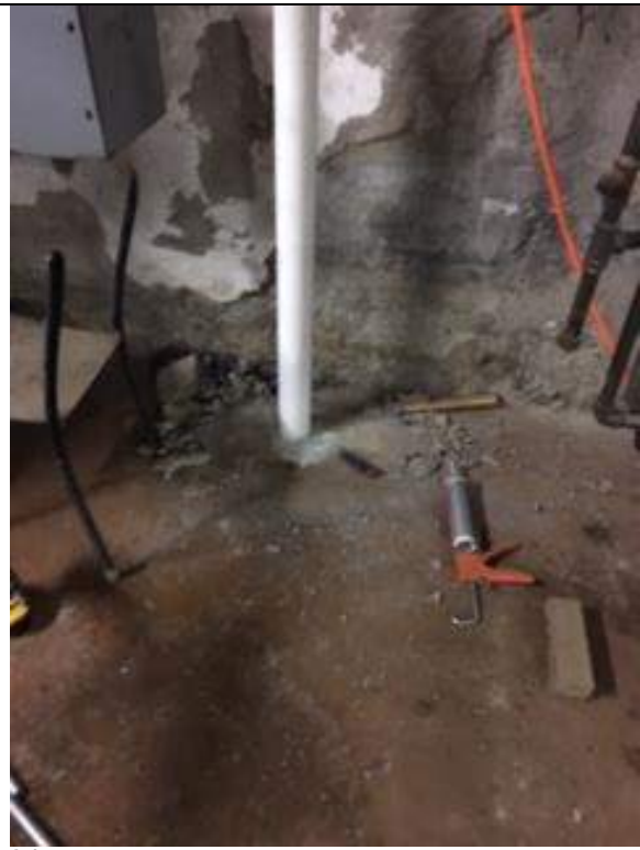
DP-01 - Vertical depressurization point during installation.
