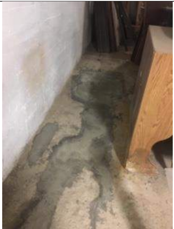
Sealing of floor cracks in building basement.
