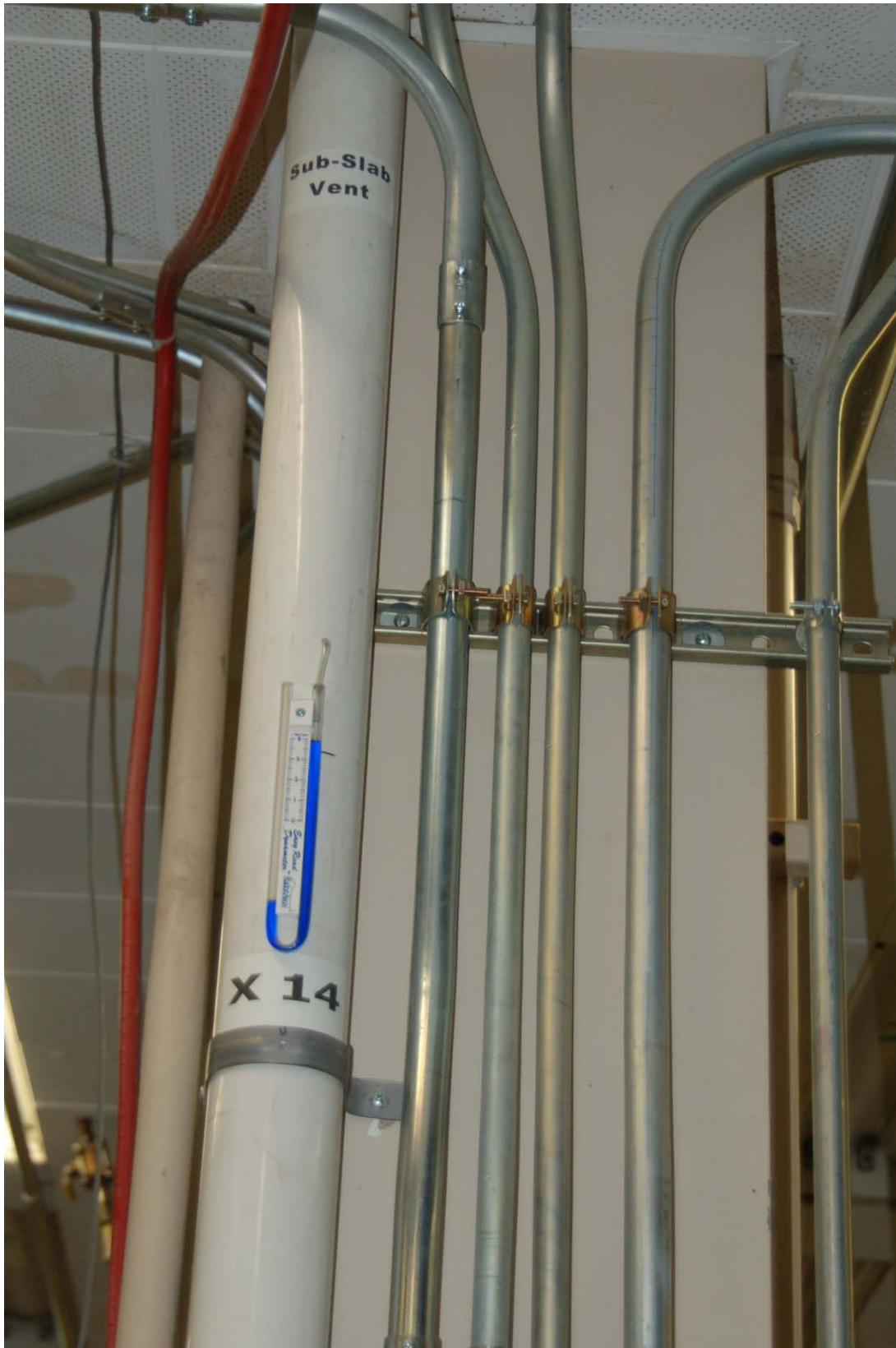
FIGURE 13. Typical Vent Pipe Labeling.
