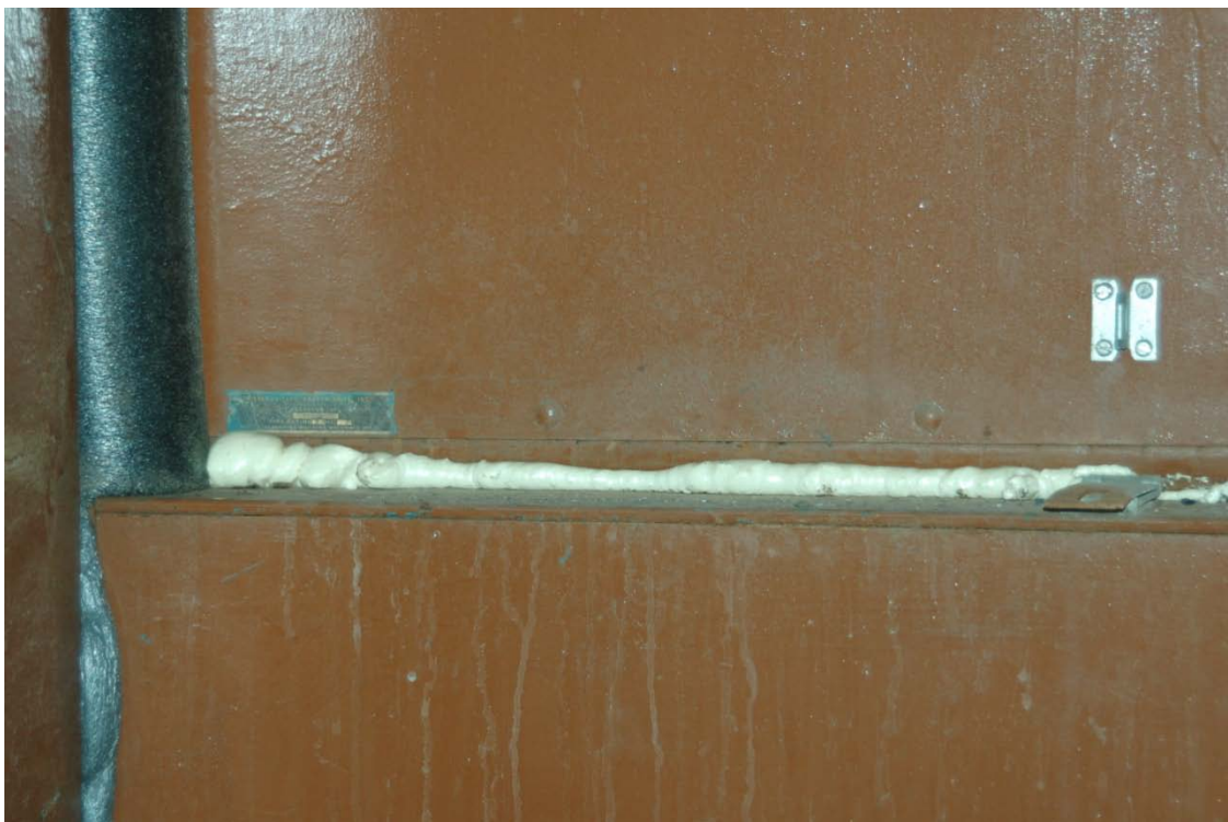
FIGURE 4. Typical Sealing of Creases and Tiny Spaces with Caulk.
