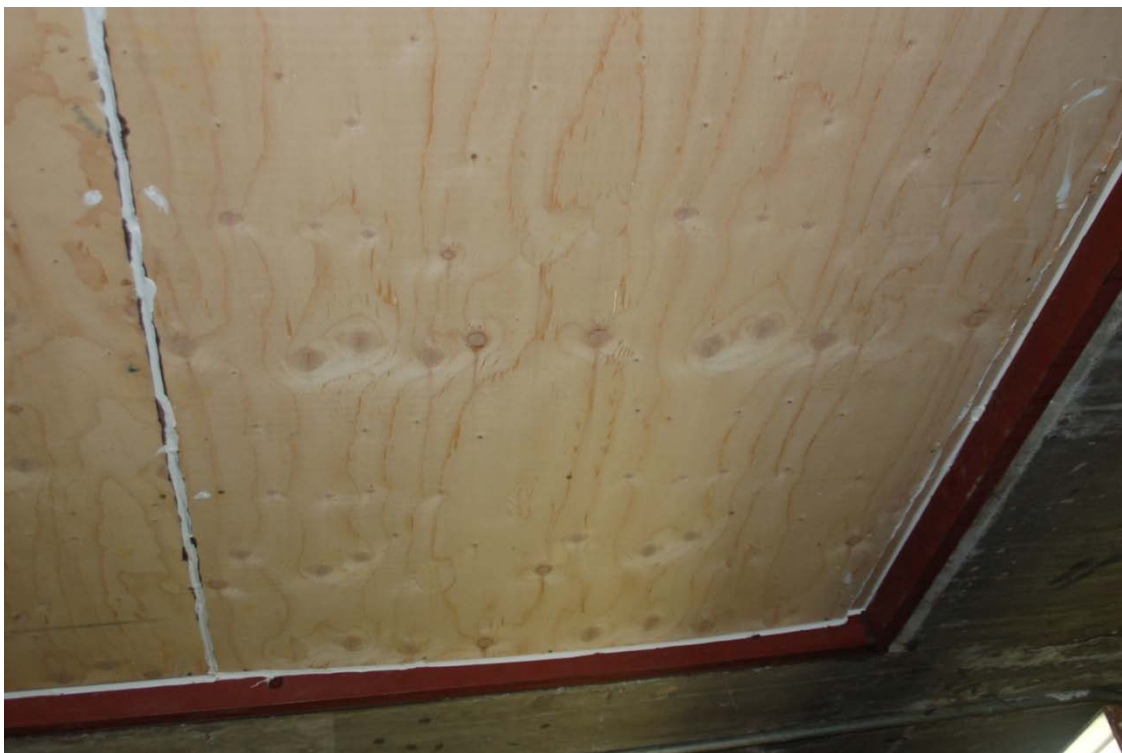
FIGURE 5. Typical Sealing of Large Openings.
