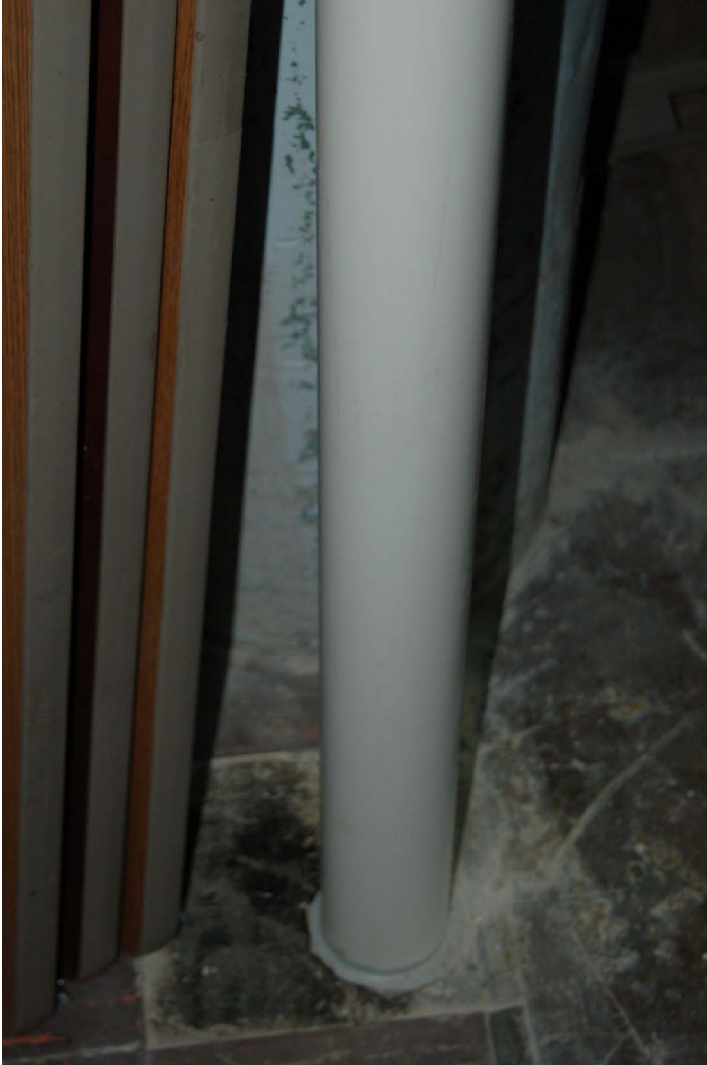
FIGURE 8. Typical Floor Penetration Sealed With Caulk.
