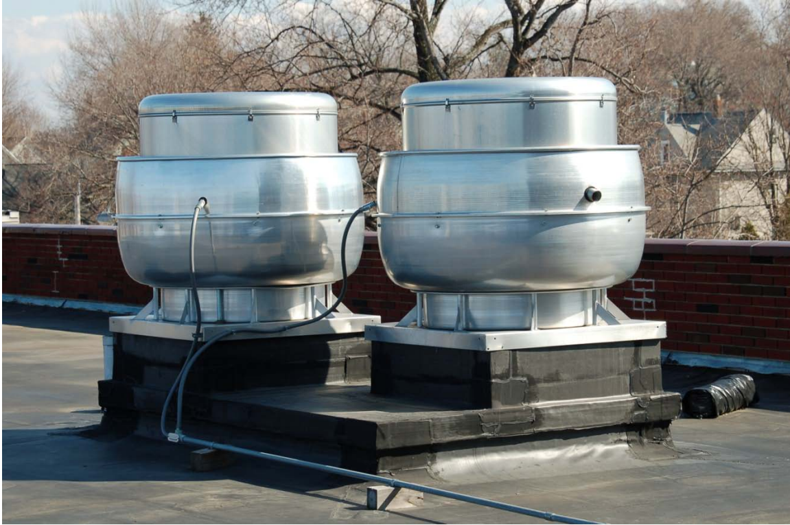
FIGURE 10. Exhaust Fans Installed on Building 10 Roof.
