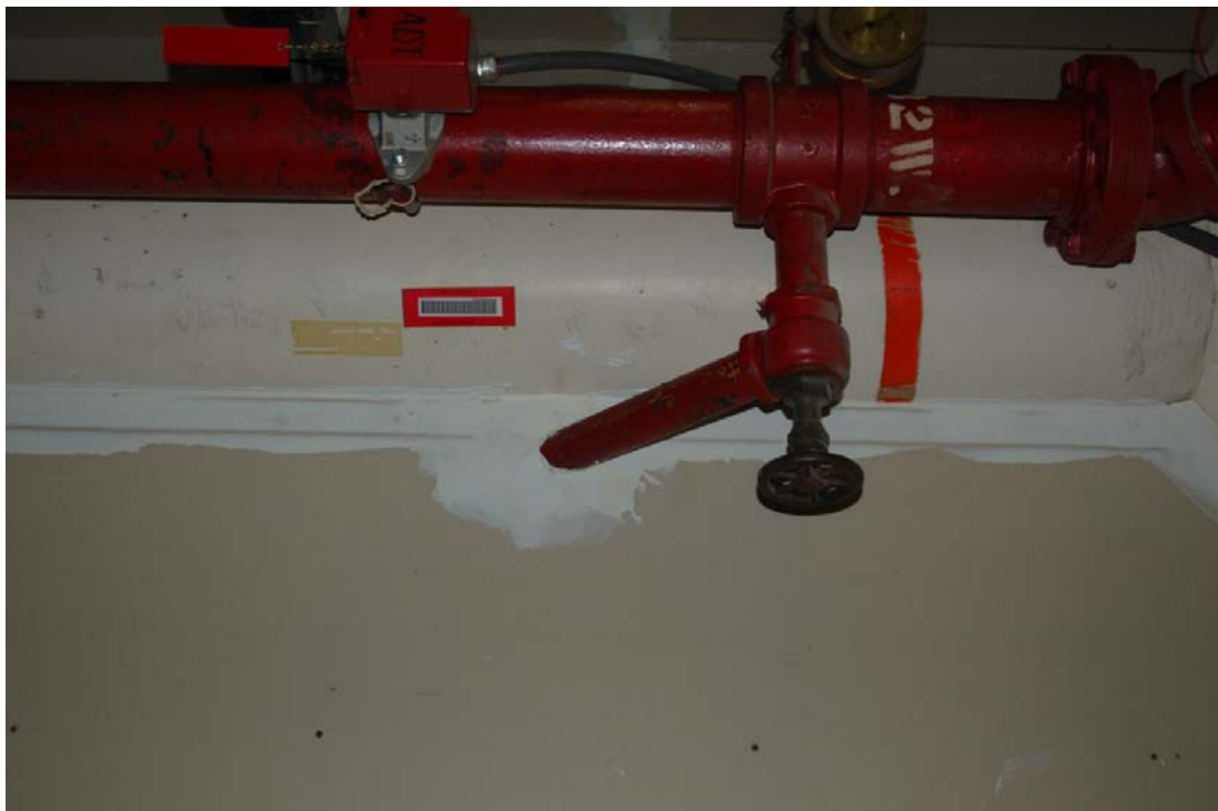
FIGURE 7. Potential Sources of Leaking Air Sealed With Caulk.
