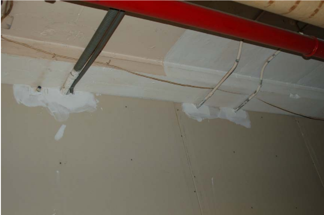
FIGURE 6. Areas Around Utilities Sealed with Caulk.
