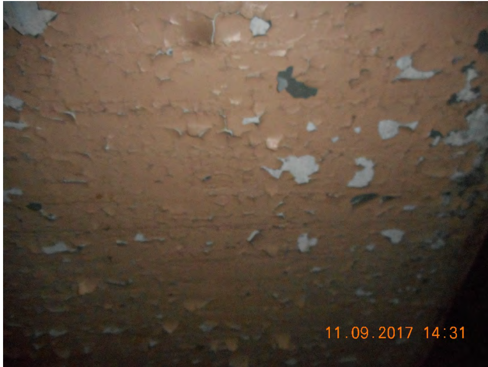
Interior – Painted Surface
