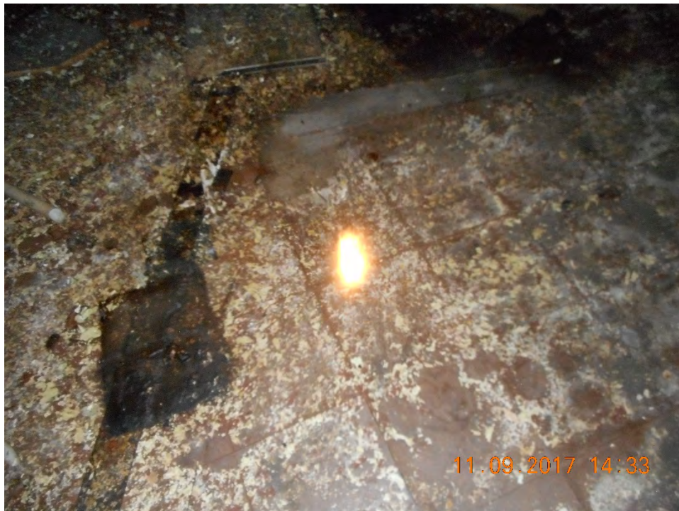
Interior – Second Floor Tile
