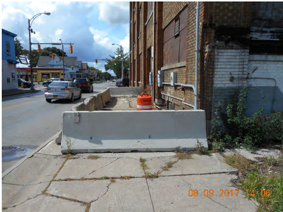
Exterior View South Side Along Avenue D
