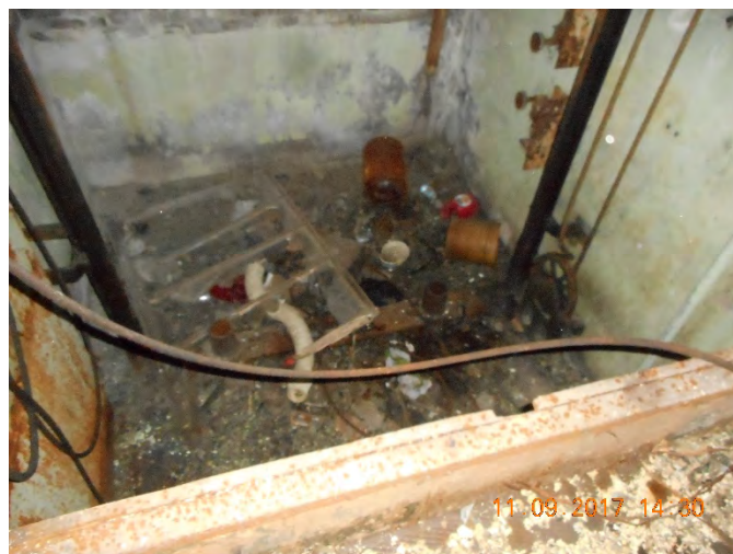
Interior – First Floor Elevator Pit
