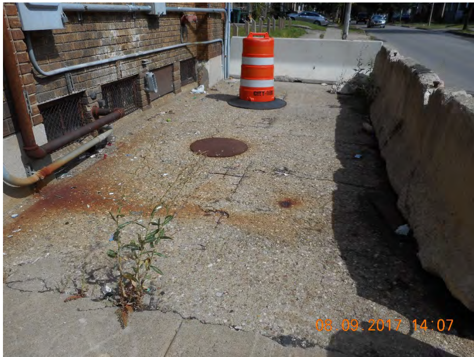
Avenue D Sidewalk Over Vault
