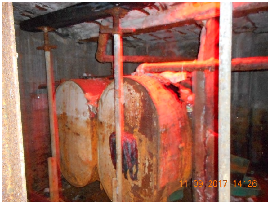
Basement – Vault Beneath Sidewalk
