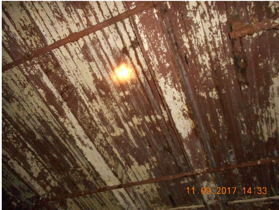
Interior – Second Floor Ceiling
