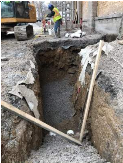
February 5, 2020 – View of sewer lateral excavation looking east with some stone backfill and bedding
