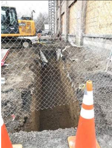
February 4, 2020 – View of sewer lateral excavation looking east.
