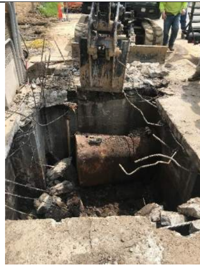
May 22, 2019 – View of AST tank vault with top removed. View looking east.
