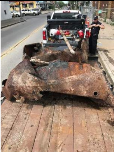
May 22, 2019 – View of corroded 275-gallon ASTs being loaded onto trailer looking west.
