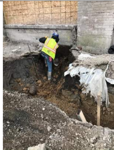
February 5, 2020 – Sewer lateral excavation towards east and excavated south towards building. View looking SE
