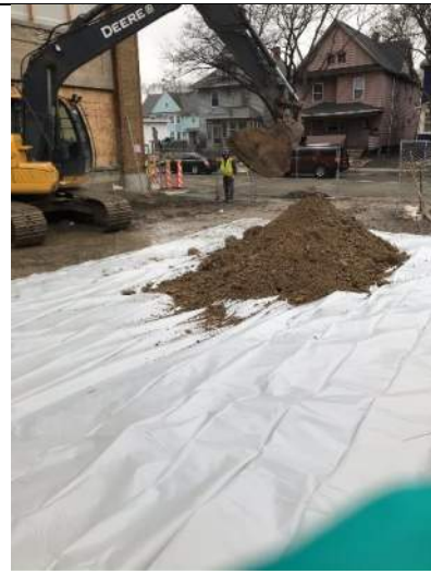
February 4, 2020 – On-site excavation and staging of soil removal for installation of sewer lateral. View looking SW.
