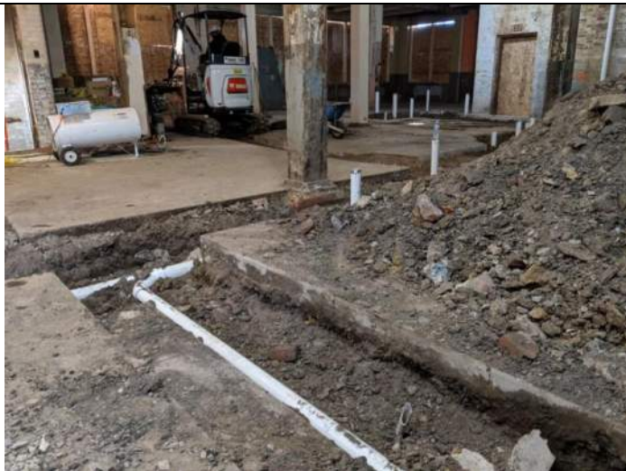
January 8, 2020 – View of trenches and plumbing installation looking southwest.
