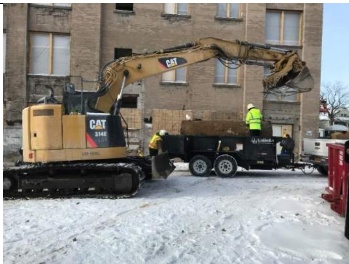
December 19, 2020 – 1,000 gallon UST removed from tank pit and loaded onto trailer. View looking west.
