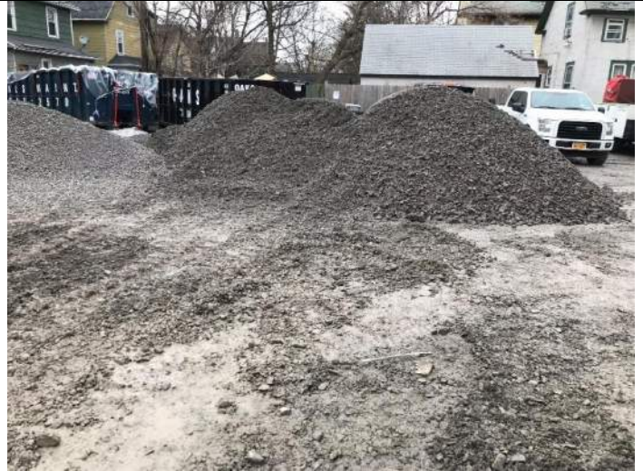
February 4, 2020 – View of imported stone stockpiles, looking east.
