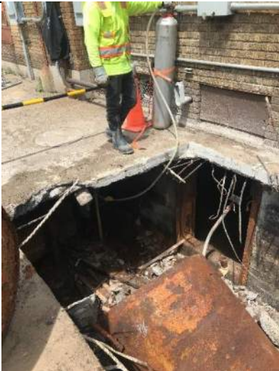
May 22, 2019 – View of AST removal and inerting AST using CO 2 . View looking northwest.
