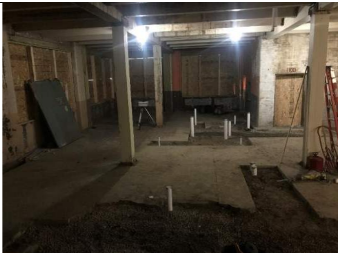
January 14, 2020 – Plumbing installation trenches backfilled view looking west
