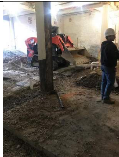
January 14, 2020 – Backfilling plumbing trenches view looking northeast.
