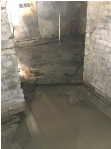
December 30 – Basement floor removed, water pooled in basement facing southwest.
