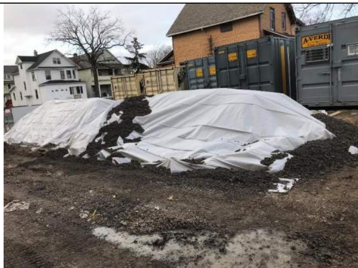
February 5, 2019 – View of soil staged on poly and covered with poly. Soil from sewer later excavation. View looking NW.
