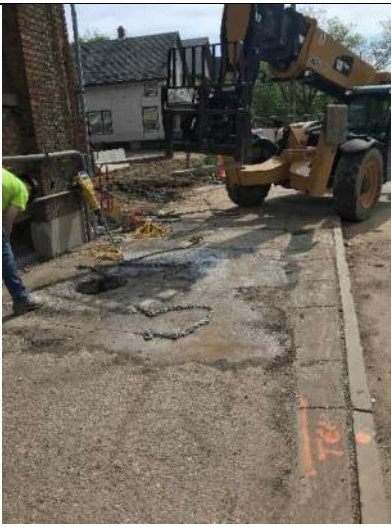
May 22, 2019 – View of AST tank vault prior to tank removal. View looking east.
