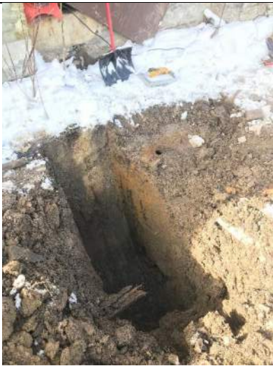
November 13, 2020 – Test pit excavation along site southern UST.
