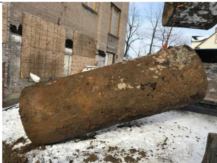
December 19, 2020 – Southern UST removed from excavation. Looking north northwest.
