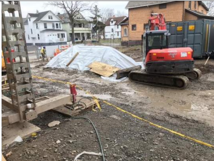
February 4, 2020 – View of soil removed as part of sewer lateral excavation stage on poly sheeting and covered in poly.
