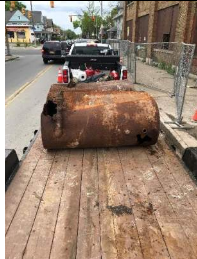
May 22, 2019 – View of second load of corroded 275-gallon ASTs being loaded onto trailer looking west.
