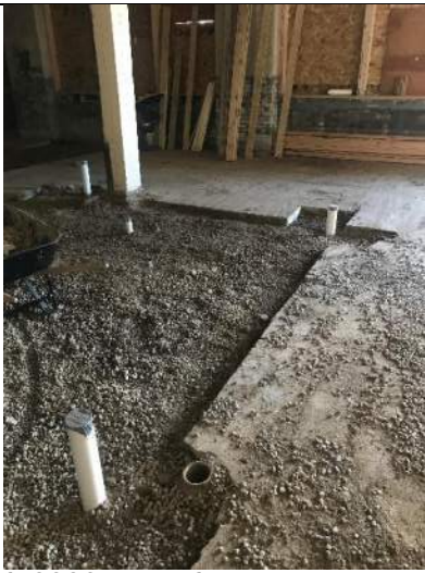
January 14, 2020 – Backfilled plumbing trenches view looking northwest.
