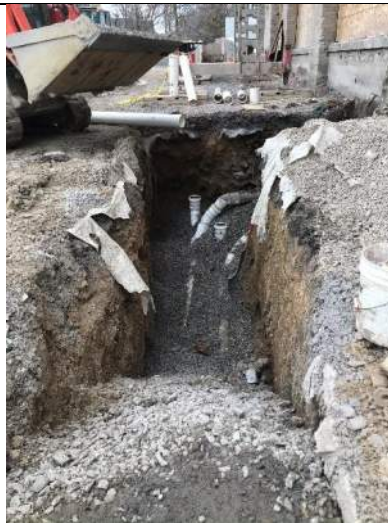
February 5, 2020 – View of installed sewer piping looking east.
