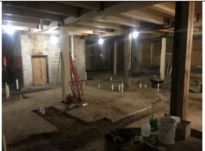
January 14, 2020 – Plumbing installation trenches backfilled view looking southwest.
