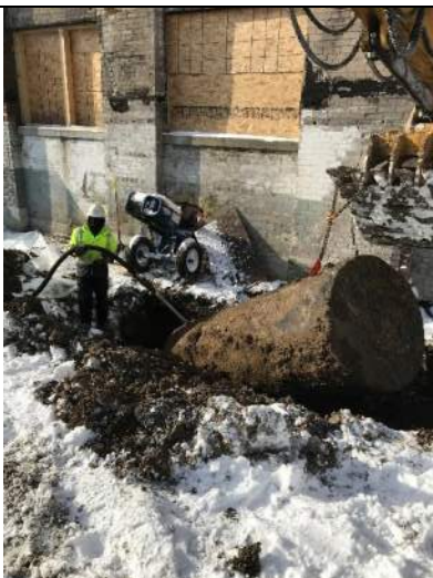
December 19, 2019 – 1,000 gallon UST removal immediately east of the Site building. View looking SW.
