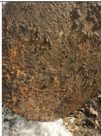
December 19, 2019 – View of south end of 1,000 gallon UST. Several small holes identified in tank.
