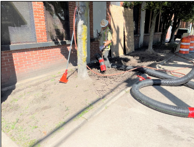
Photo No. 3 Vacuum Extraction of Surface Soils
