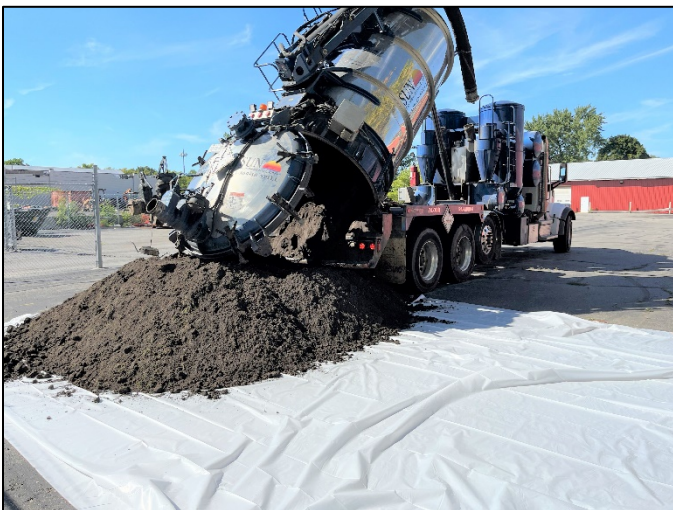
Photo No. 5 Stockpiling Topsoil Prior to Disposal
