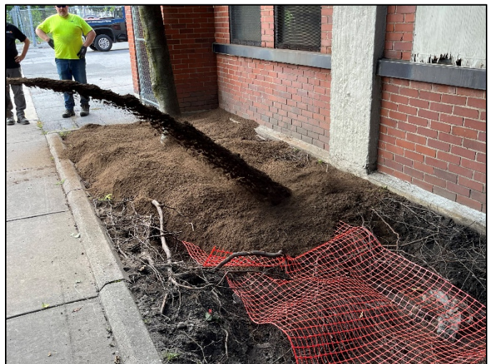
Photo No. 6 Placement of Imported Topsoil Over Demarcation Barrier
