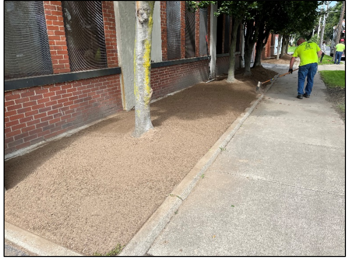
Photo No. 8 Raked and Graded Cover System
