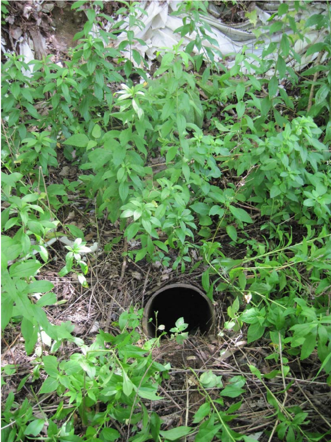
Description: Pipe J.
