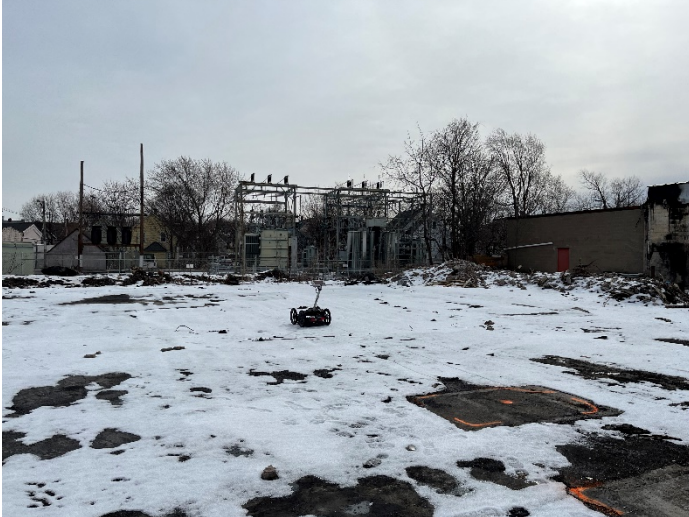
Photo No. 3 View of the site facing southeast
