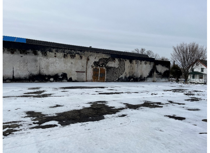
Photo No. 4 View of the site facing southwest
