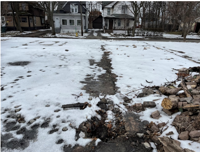
Photo No. 7 Suspected former floor drain
