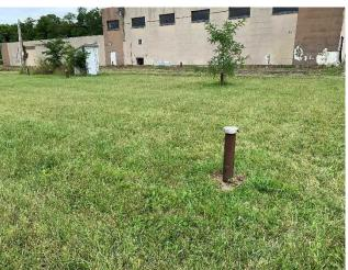
Photo No. 12 OW-3 missing lock
