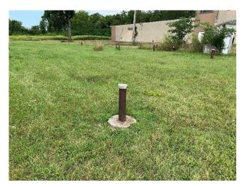
Photo No. 13 OW-2 missing lock
