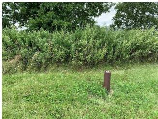
Photo No. 3 OW-5 missing cover & lock
