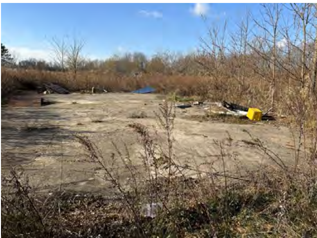
Photo No. 5 Concrete pad observed on the northern wooded area.
