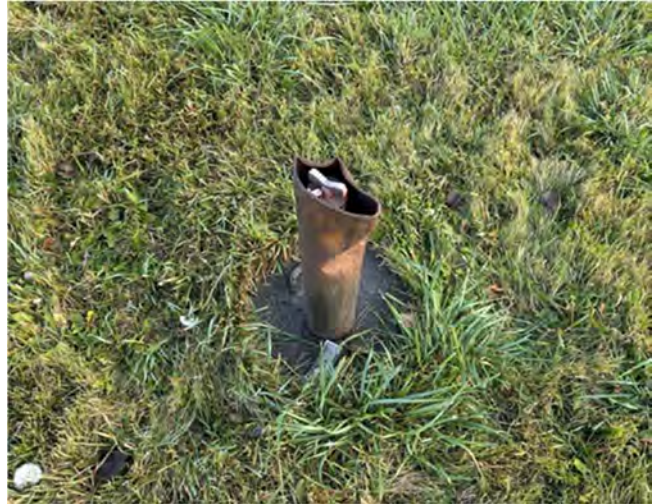
Photo No. 8 OW-1 damaged from lawn mower.
