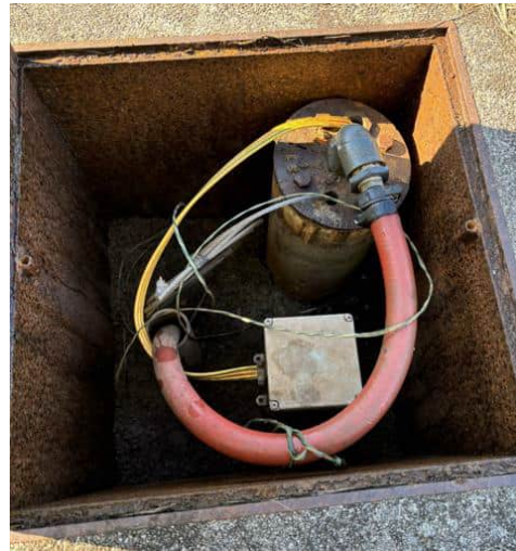
Photo No. 10 interior of injection well pump.
