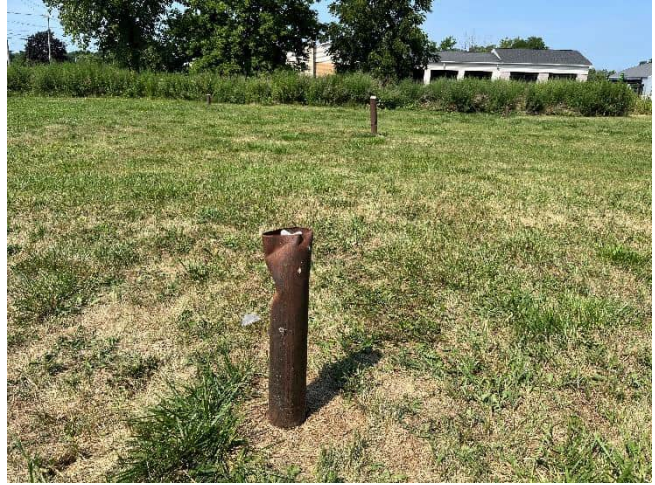
Photo No. 8 OW-1 damaged from lawn mower.
