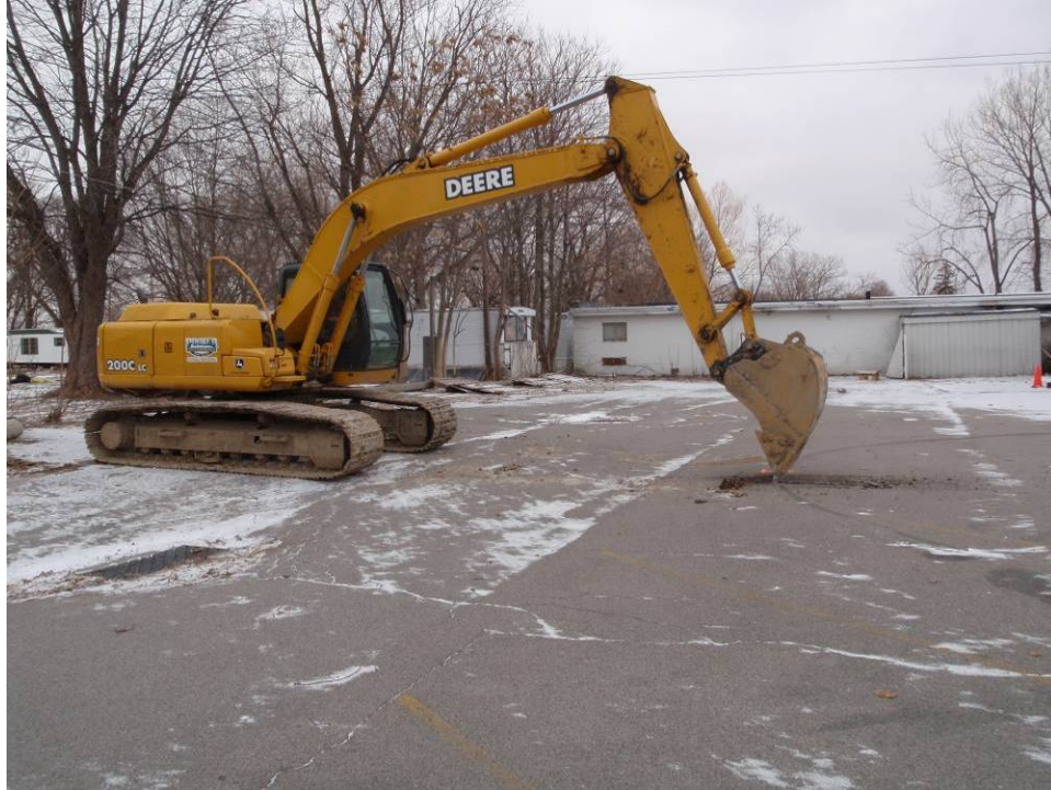
Photograph 1: Typical excavation methodology, facing northeast
