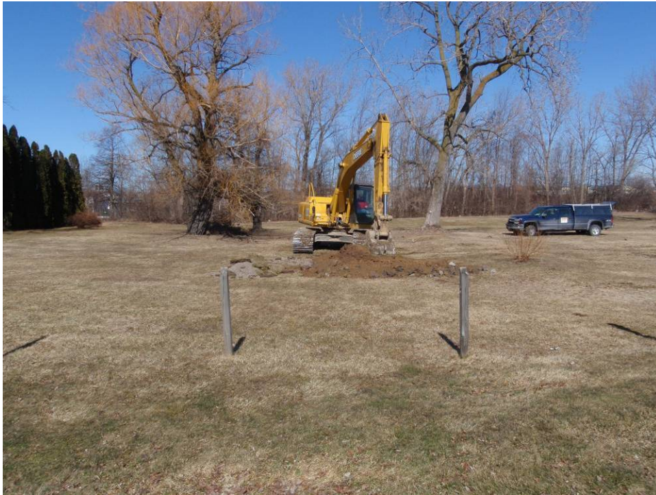
General area of RMSC Can 170, from Lakeshore Drive, facing north
