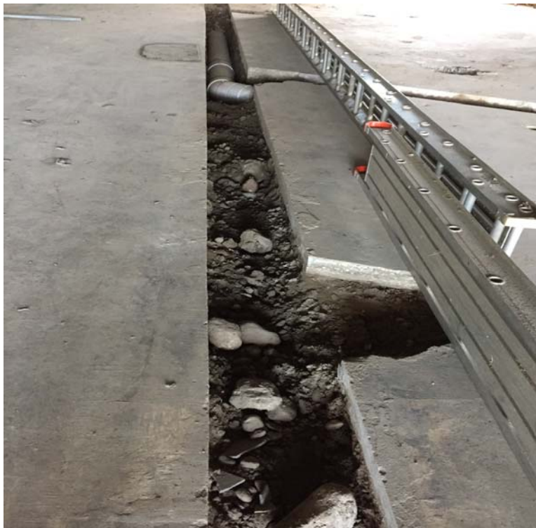
Excavated plumbing utility trench with 10-inch diameter drain pipe installed, looking South.
