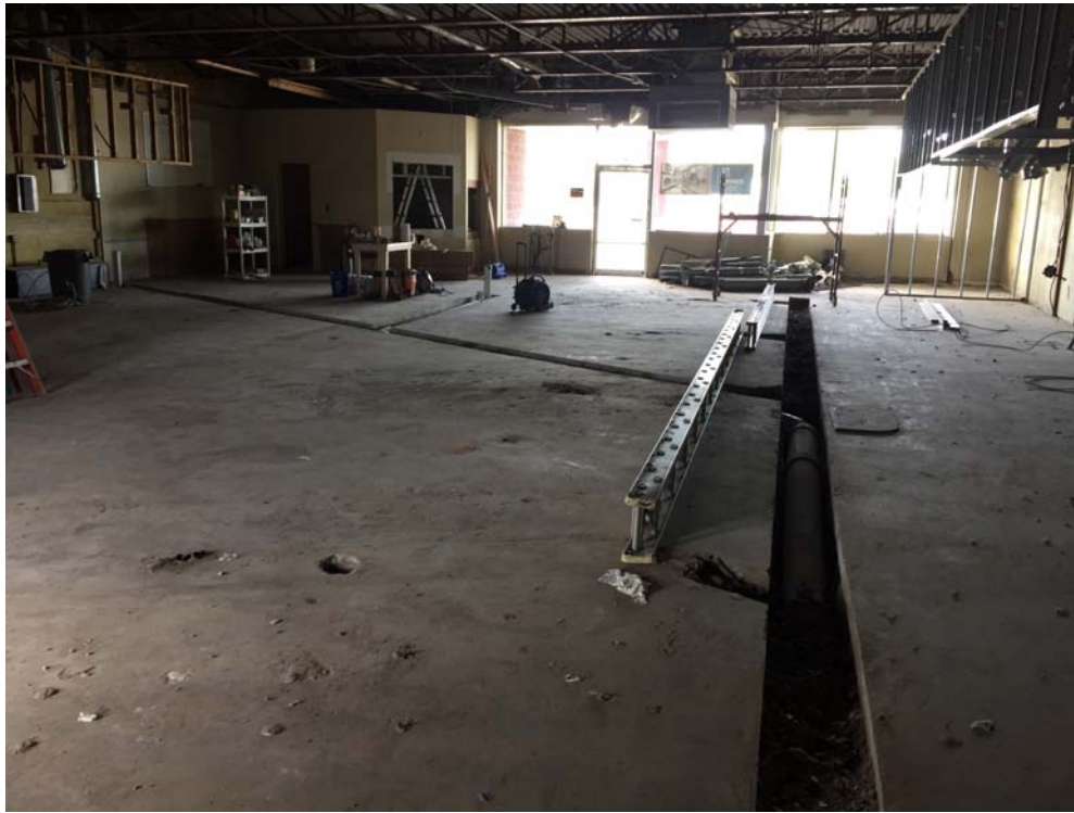
Excavated plumbing utility trench with 10-inch diameter drain pipe installed, looking North.
