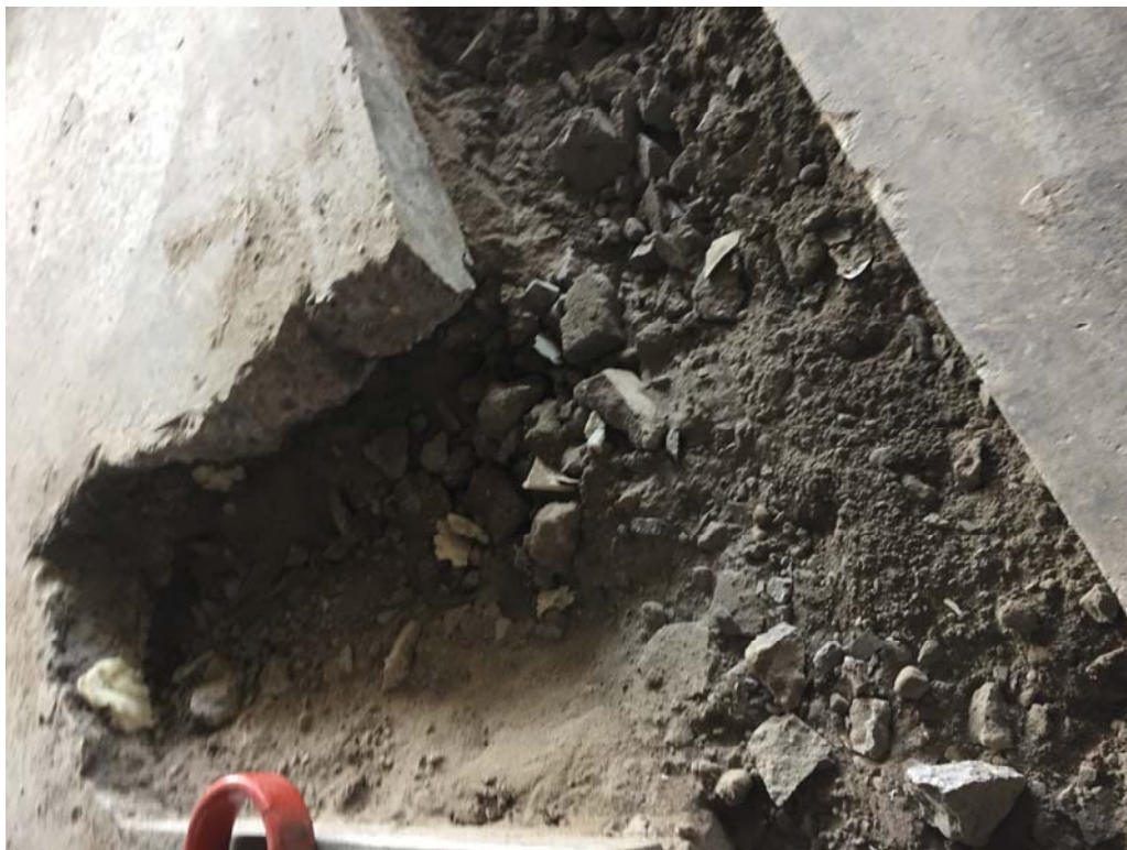
Excavated plumbing utility trench.
