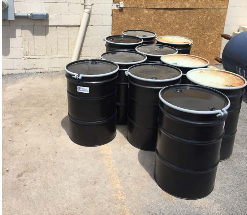
Staged containerized utility trench excavation spoils in NYSDOT-approved 55-gallon steel drums.
