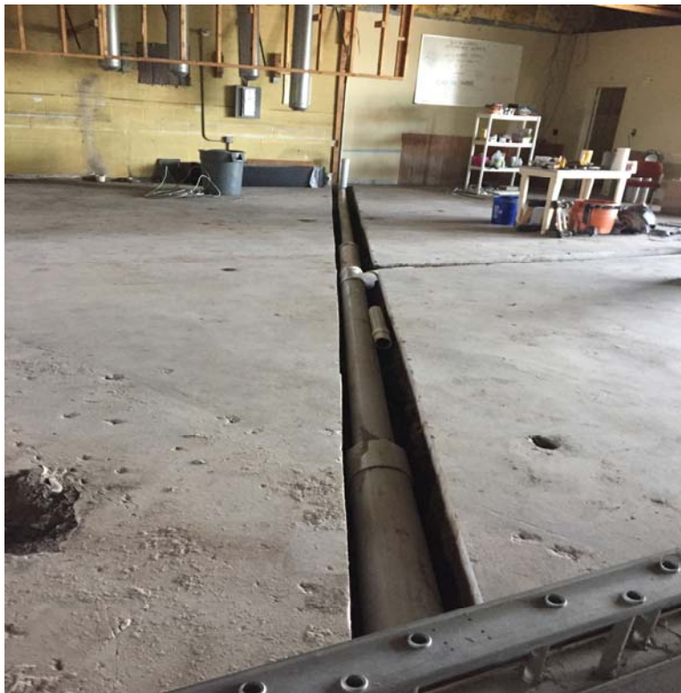
Excavated plumbing utility trench with 10-inch diameter drain pipe installed, looking West.
