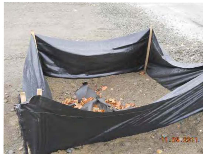
Silt Fence around MH @ G1
