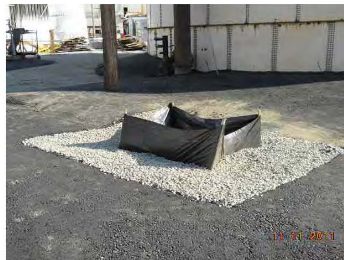
A1/A2 INLET (silt fence w/ gravel perimeter)
