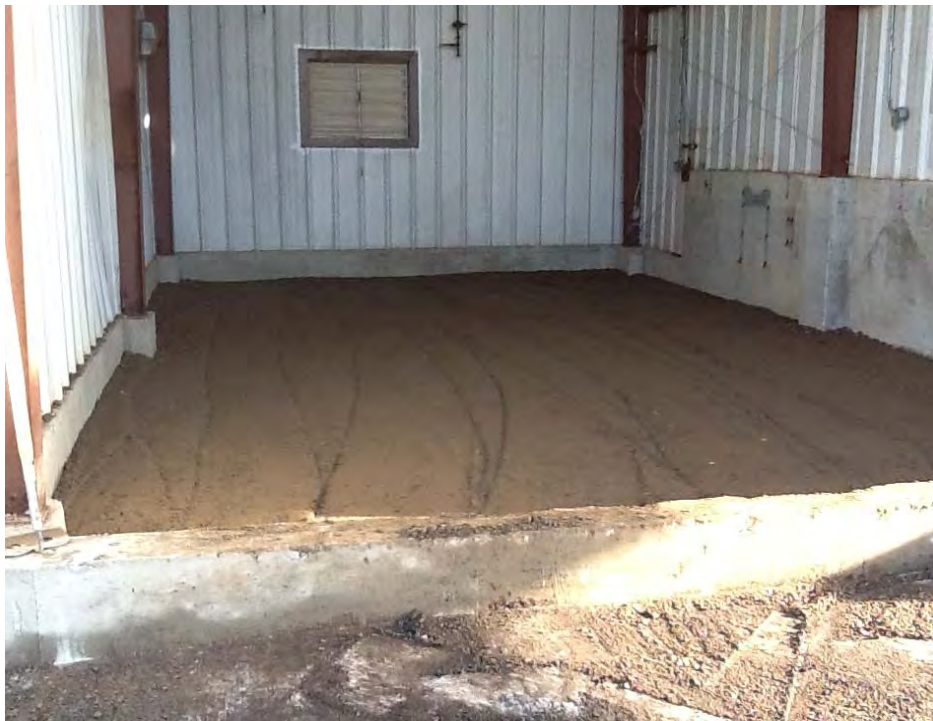
Photograph 23. Metal building demo complete; depressed floor backfilled with item 4.
