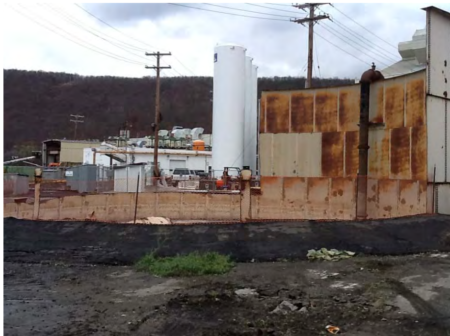
Photograph 19. Demo progress on EQ tank.
