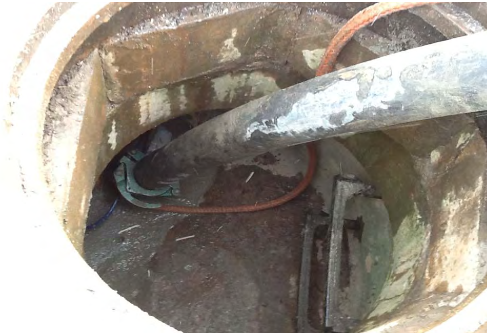
Photograph 7. Filling pipe between RCB-22 and RCB-20.
