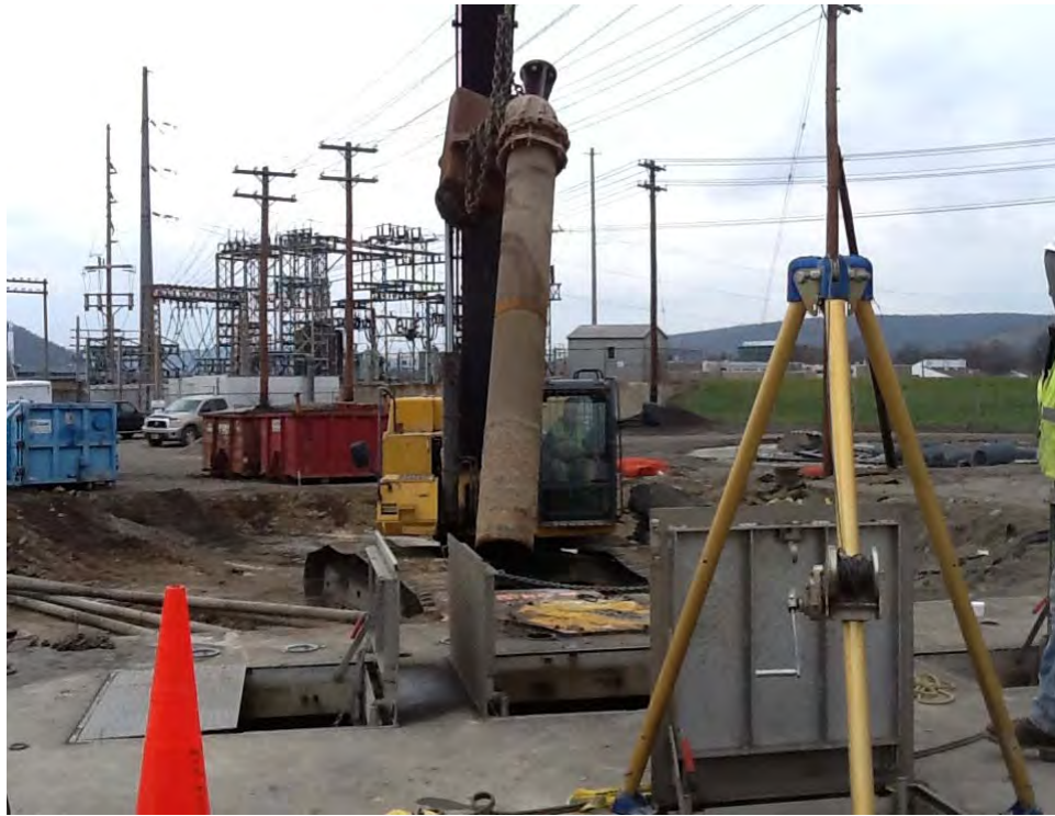
Photograph 11. Removing WWTP piping from wet well structure.
