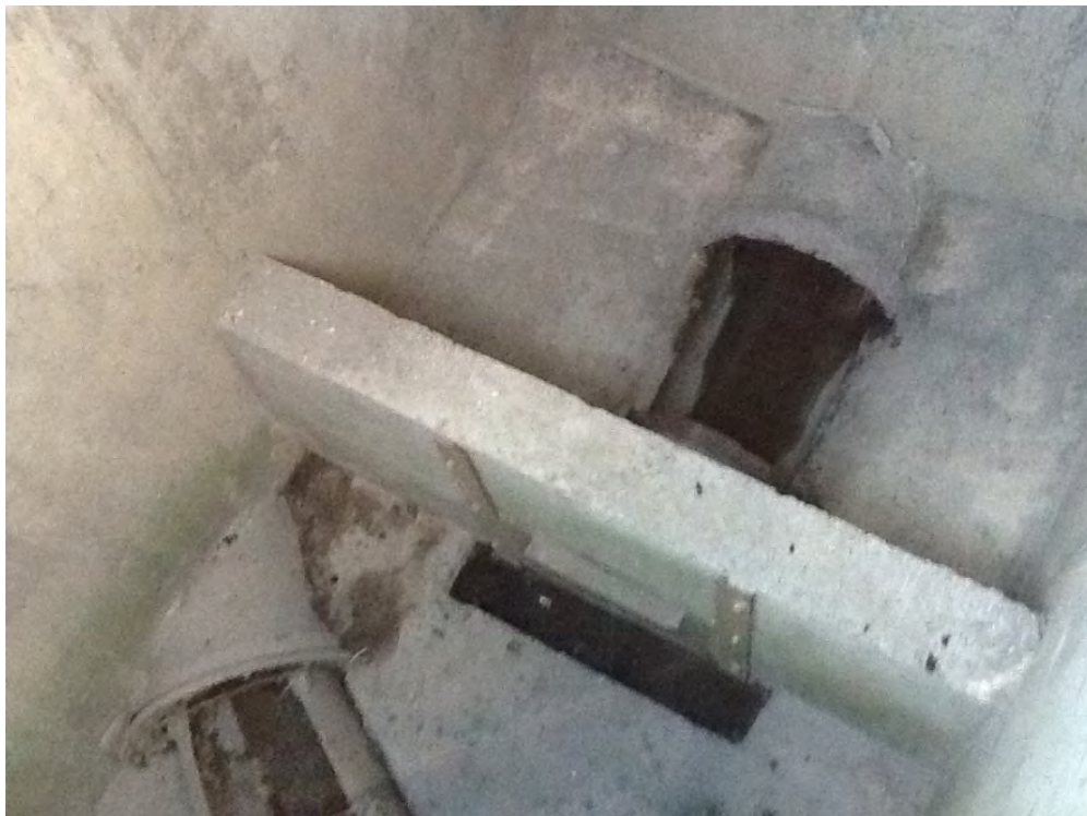
Photograph 14. Interior of diversion structure after cleaning.
