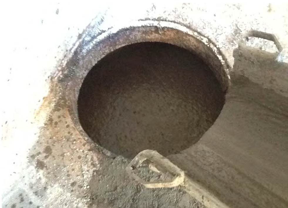
Photograph 2. Topping of manhole with flowable fill from truck.
