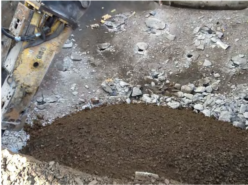
Photograph 33. Backfilling clarifiers with Item 4, note holes punched in floor of unit.
