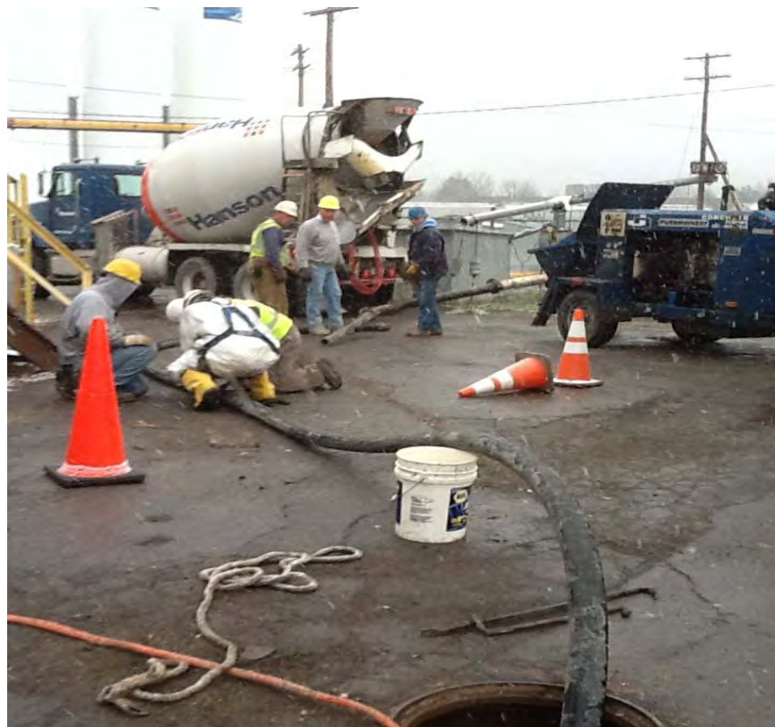
Photograph 6. Concrete pump, truck, lines and crew.
