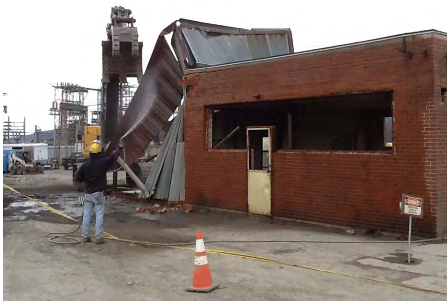
Photograph 20. Demolishing engineering building / pump house.
