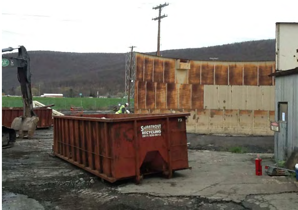
Photograph 18. Beginning EQ tank demo.
