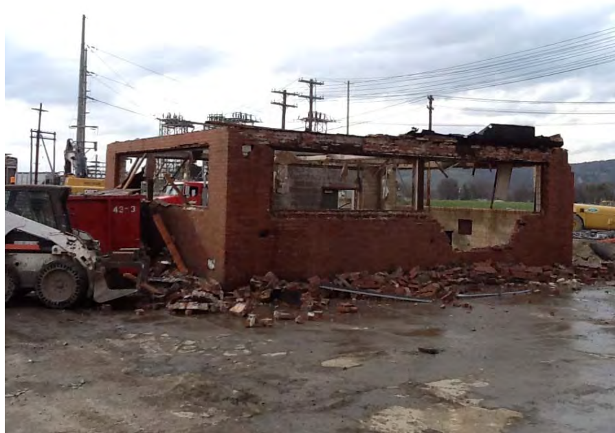
Photograph 21. Engineering building demolition.
