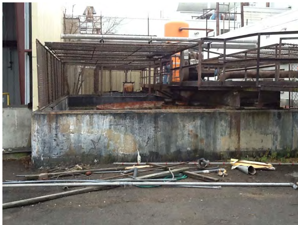
Photograph 32. Removing steel from clarifiers.
