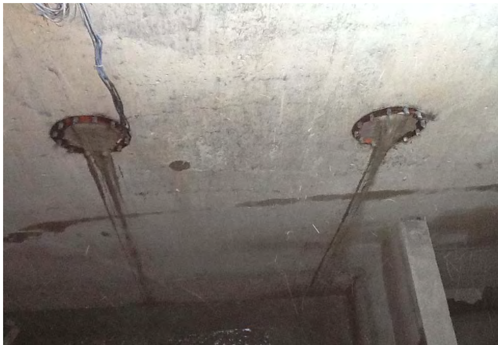
Photograph 4. Flowable fill entering wet well from former standpipe on east side of EQ tank.
