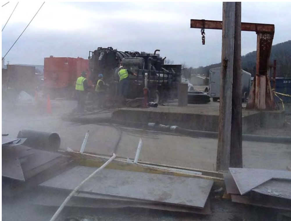
Photograph 9. Jet lines, support truck, and crew.
