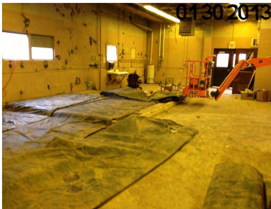
Photograph 24. Equipment removed from Block Building interior.
