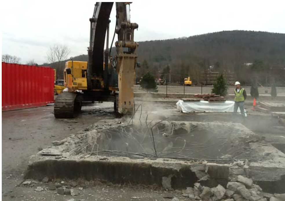
Photograph 12. Removing top of Wet Well.
