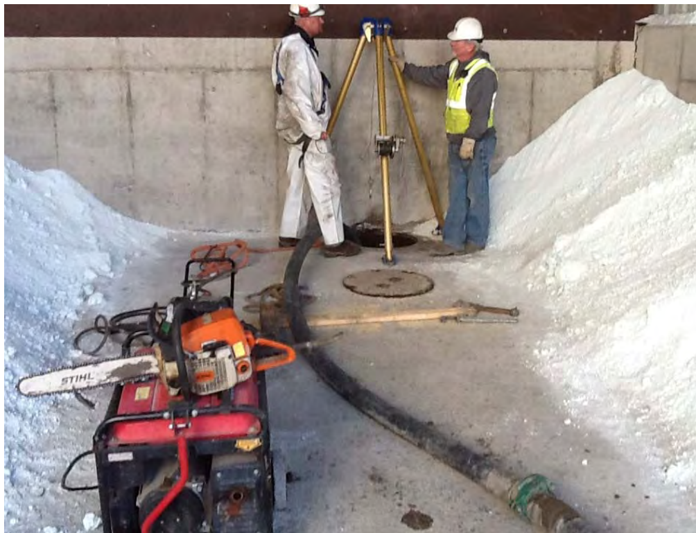
Photograph 8. Filling pipe between covered manhole and RMH-15A.
