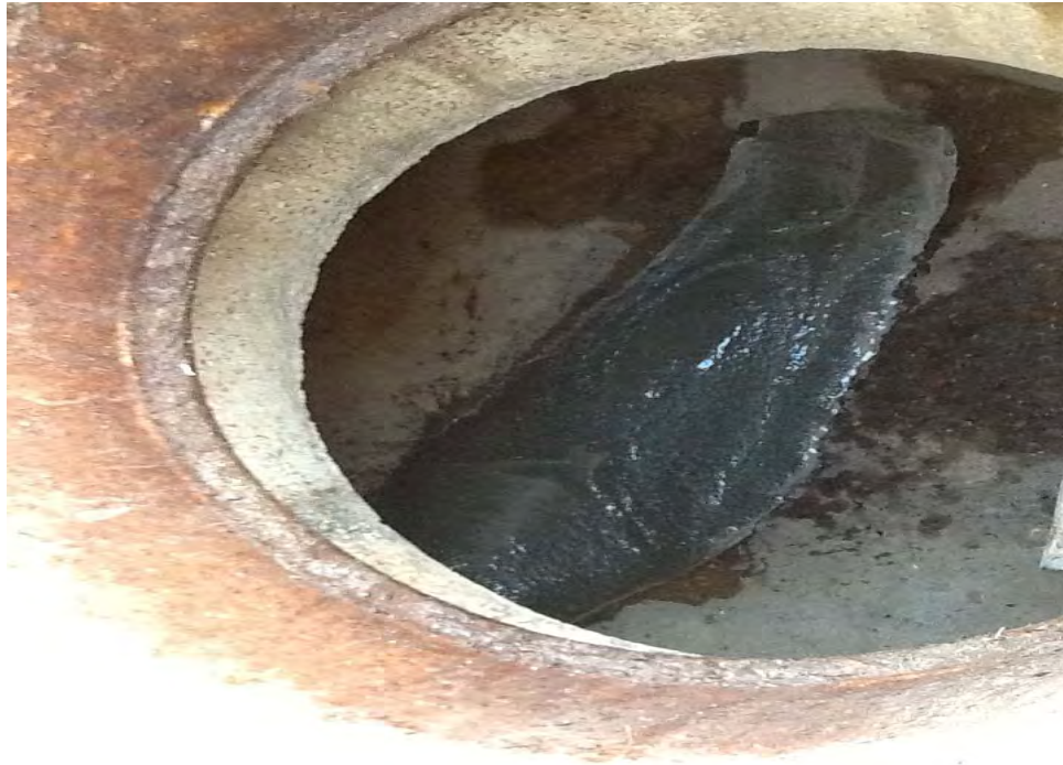
Photograph 3. Flowable fill running into RMH17 from RMH 18A.
