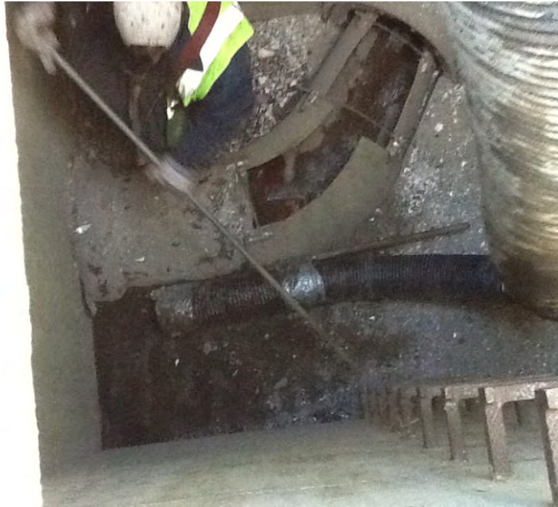
Photograph 13. Cleaning inside of diversion structure.
