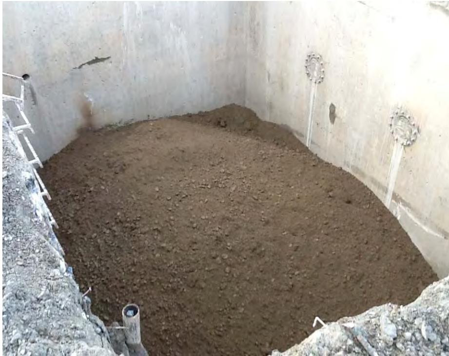
Photograph 17. Backfilling wet well.
