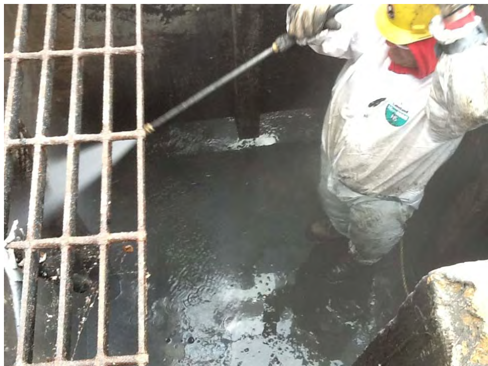
Photograph 30. Cleaning vault of clarifier.
