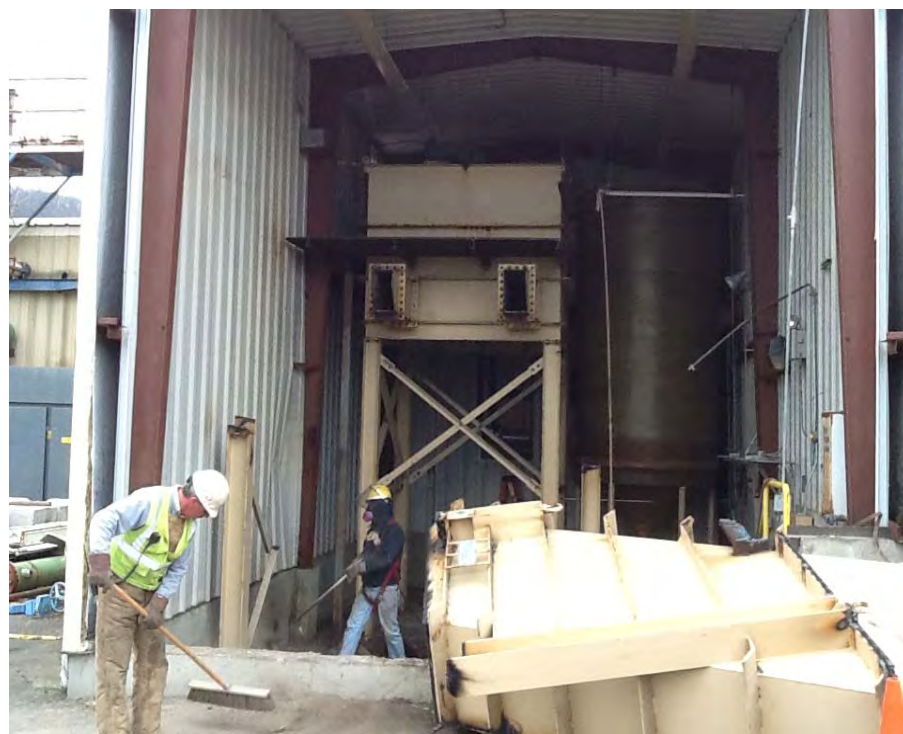
Photograph 22. Lamella cut into pieces, removed for recycling.
