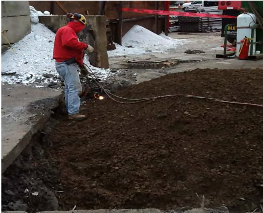
Photograph 15. Diversion structure after demo, backfilled with item 4.
