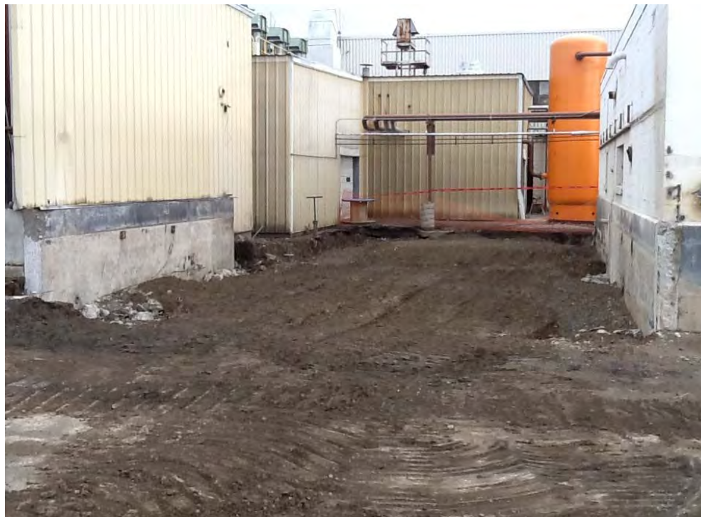
Photograph 34. Closure of clarifiers complete. Asphalt to be placed in 2013.
