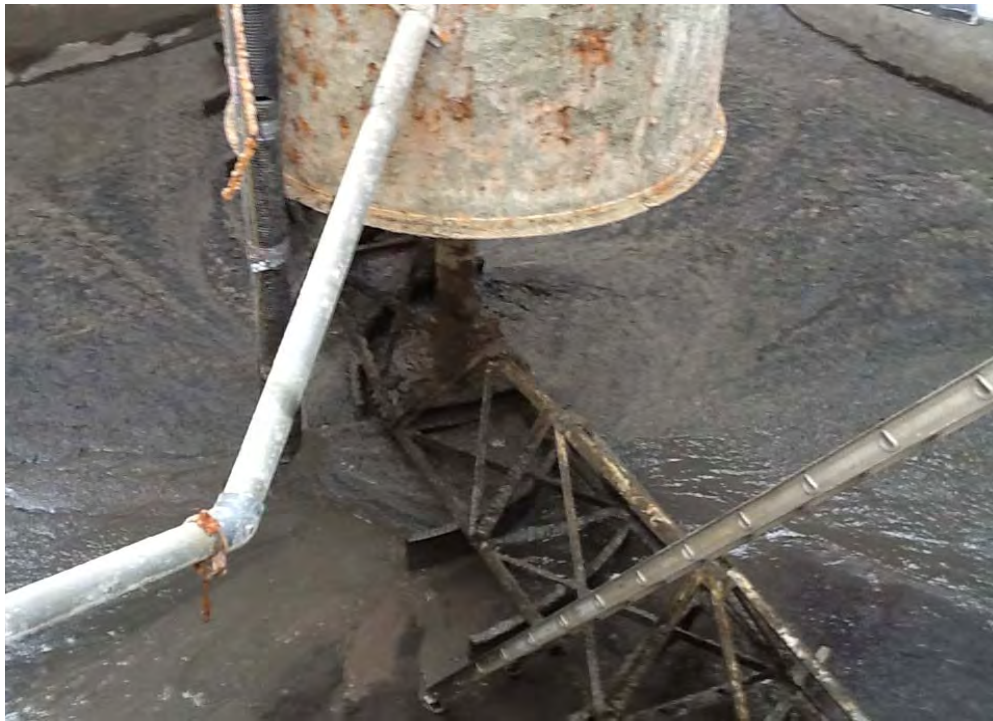
Photograph 27. Pumping sludge out of secondary clarifier.
