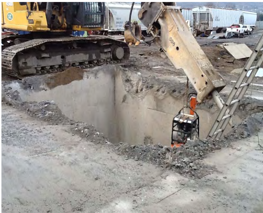
Photograph 16. Lowering plate compactor into wet well.
