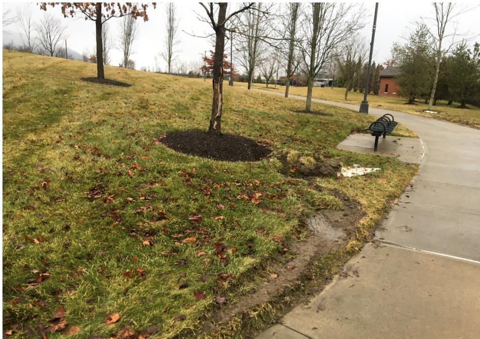
Photo 2: Rutting from snowplows in Soil Cover around park sidewalk.
