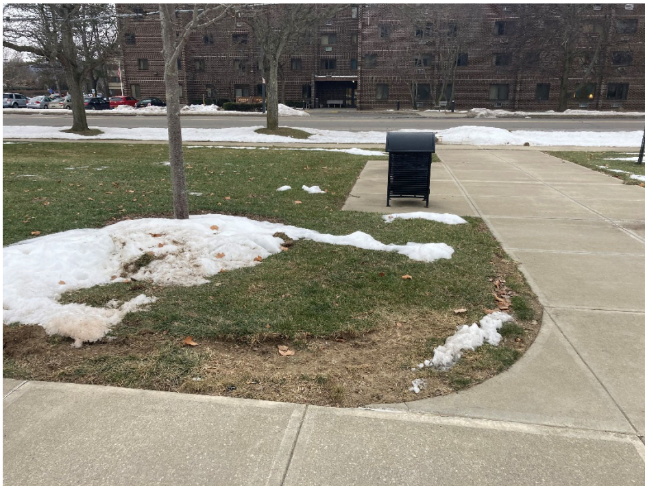
Photo 4: Rutting from snowplows in Soil Cover around park sidewalk.
