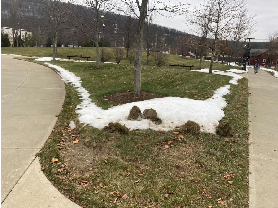
Photo 3: Rutting from snowplows in Soil Cover around park sidewalk.
