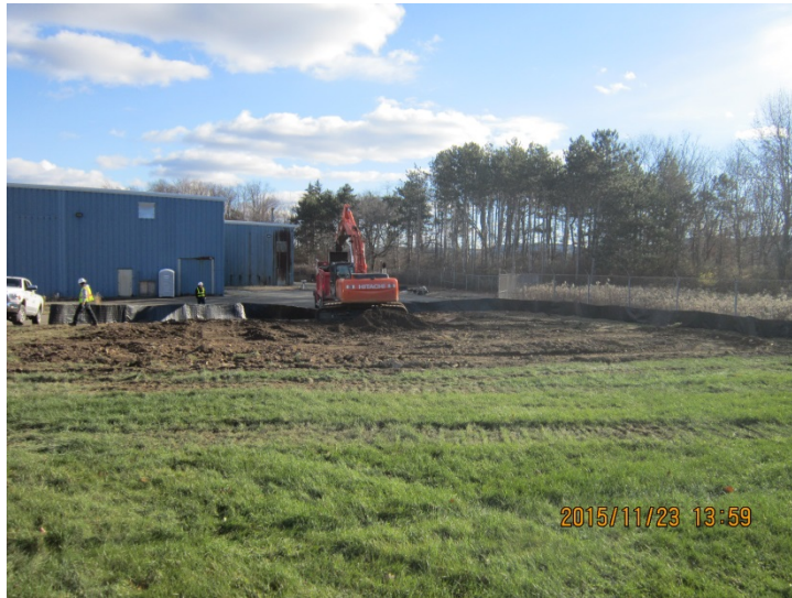
Photograph 4. Loadout for off-site disposal of stockpiled material.
