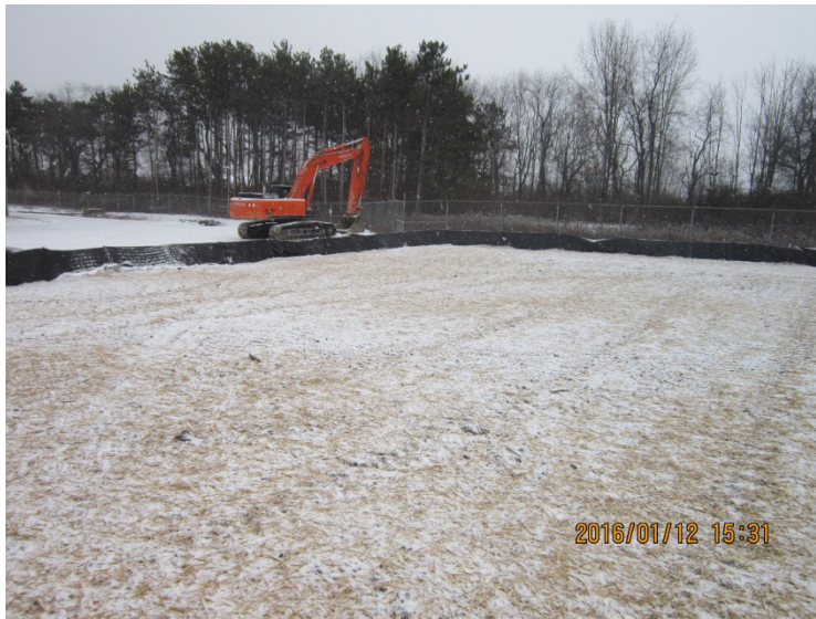
Photograph 7. Seeding and mulching completed.
