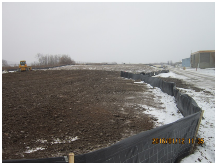
Photograph 6. Grading of topsoil.
