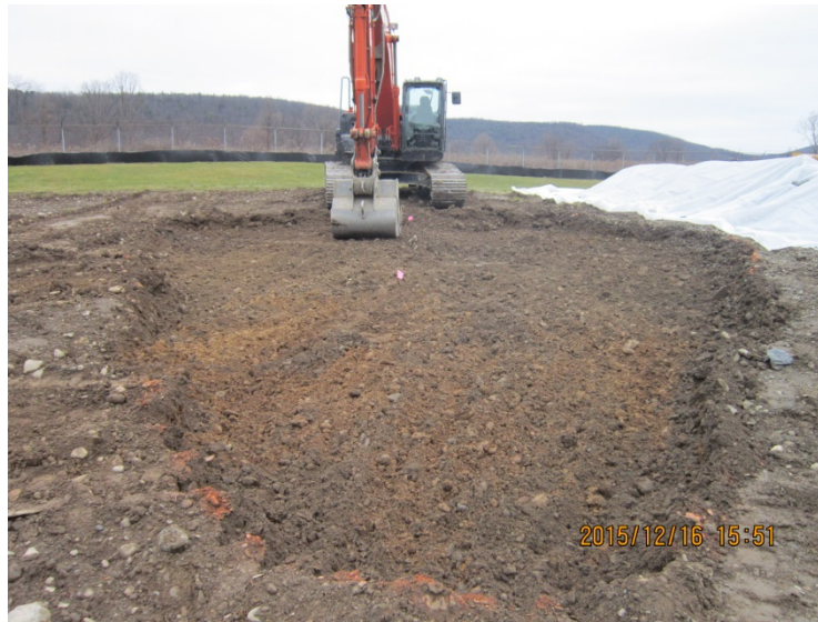
Photograph 5. Excavation of additional soils.
