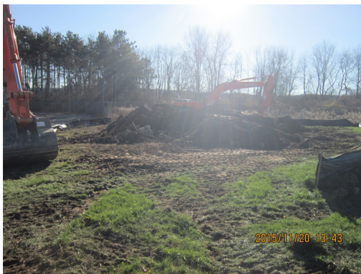
Photograph 2. Sizing concrete and asphalt.
