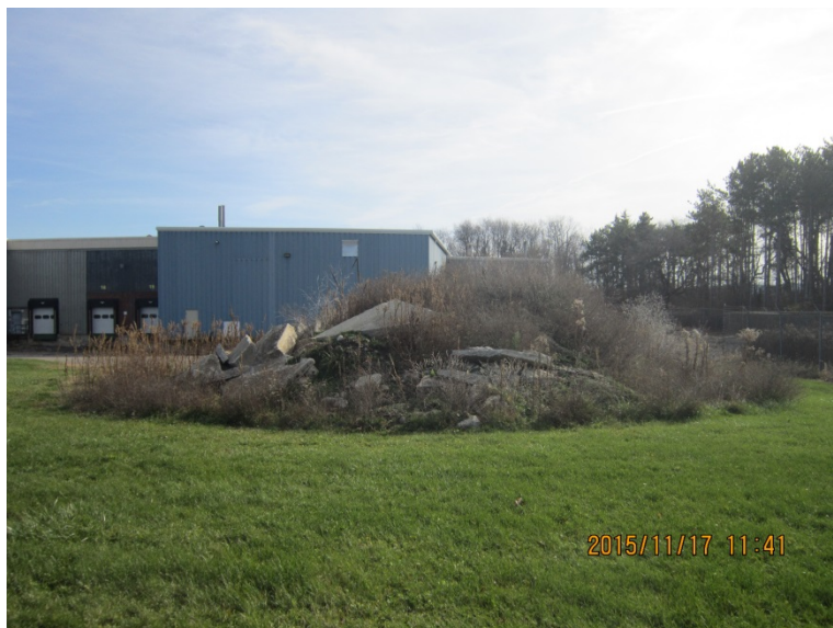
Photograph 1. IRM-6 area prior to construction activities.
