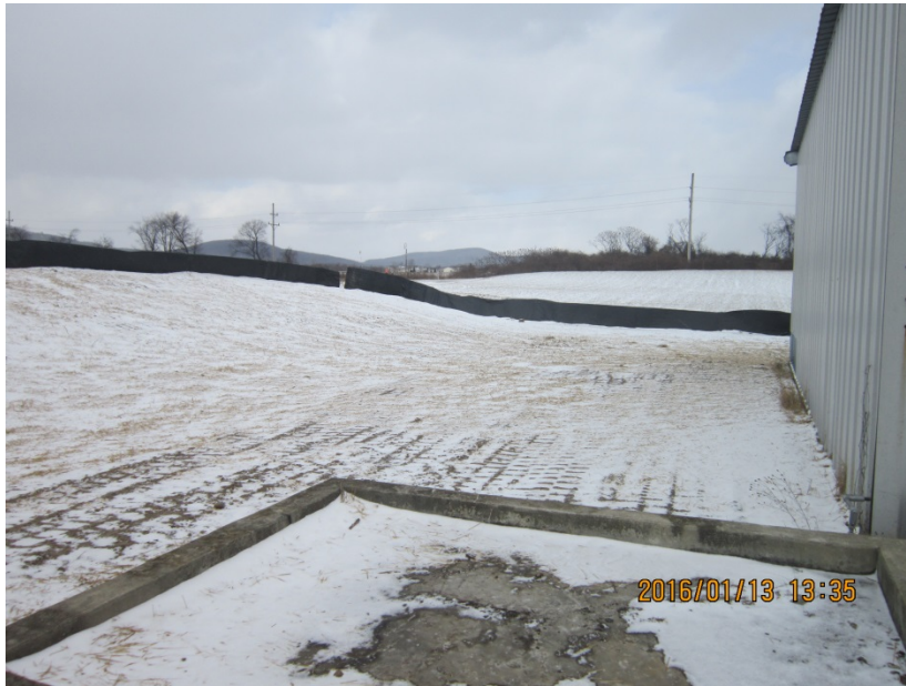
Photograph 5. Seeding and mulching completed at IRM-3.
