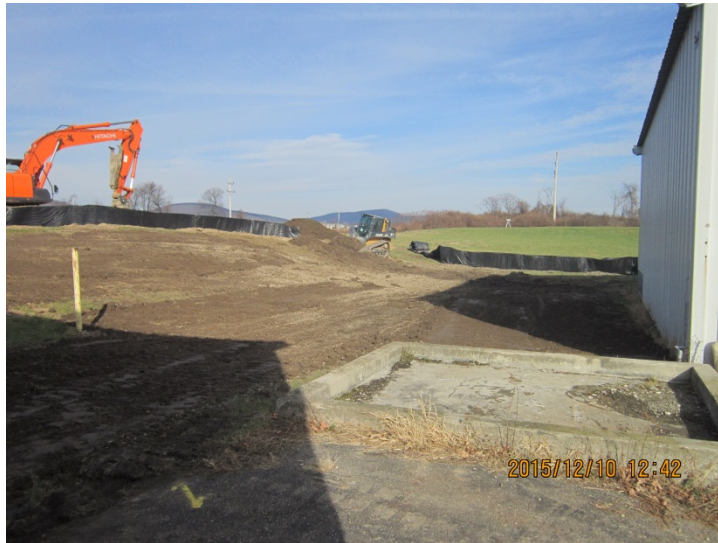
Photograph 4. Placement of reuse material and demonstrated clean imported materials to ground surface.
