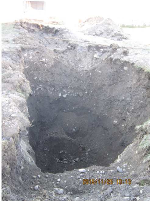
Photograph 3. Vent/fill lines removed and excavation advanced to 12.5 feet BGS.
