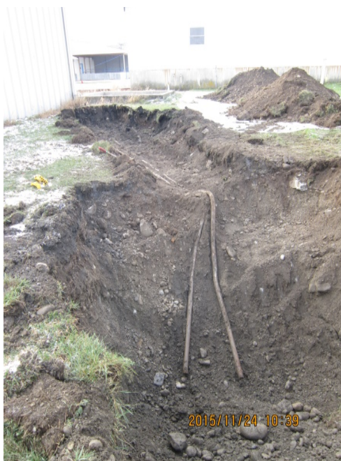
Photograph 2. Excavation following vent/fill lines. At photo bottom: vent/fill lines terminated.
