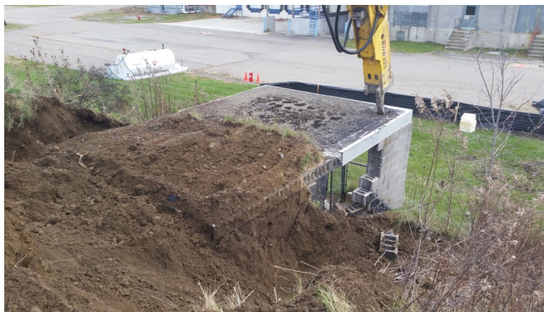
Photograph 2. Unearthing of bunker walls and roof.
