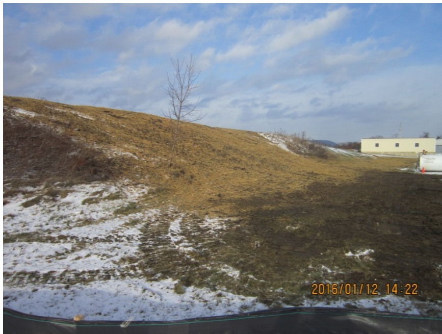
Photograph 8. Seeding and mulching completed at IRM-4.
