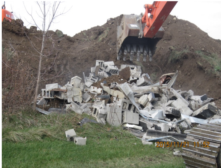
Photograph 3. Stockpile of demolished bunker material.
