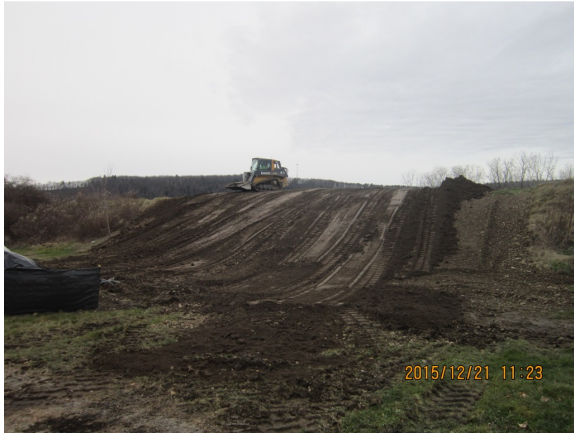
Photograph 7. Placement of import topsoil after regrading of IRM-4 area.
