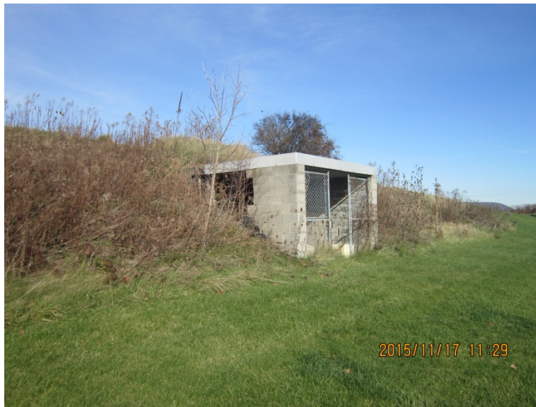
Photograph 1. IRM-4 area prior to construction activities.
