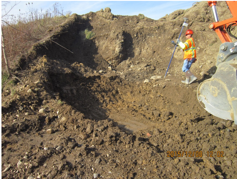
Photograph 5. First targeted excavation at sample location SB-IRM4-102.
