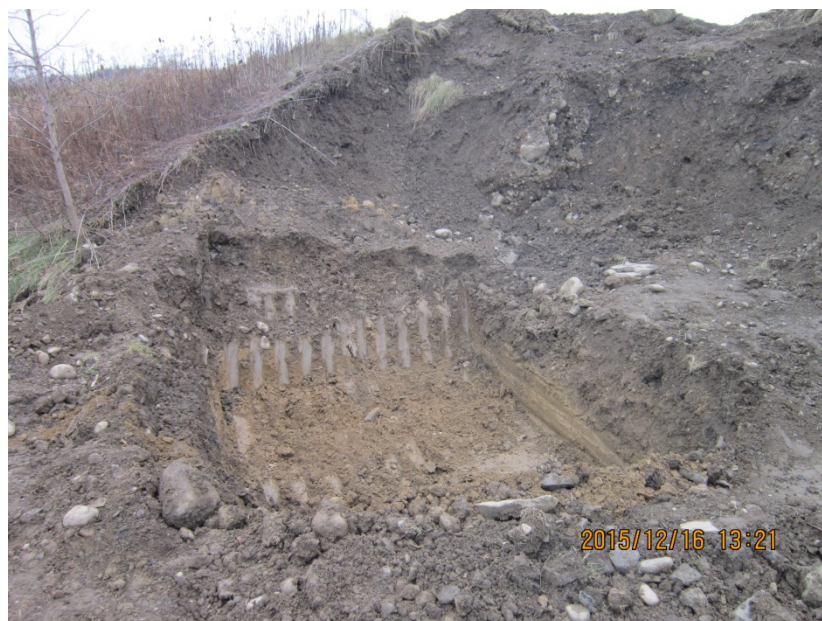
Photograph 6. First targeted excavation at sample location SB-IRM4-102.
