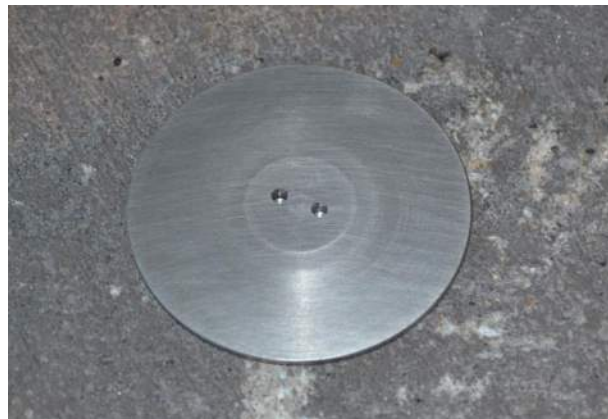
Figure 4. Secure Cover Installed
