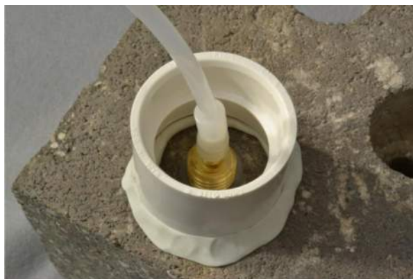
Figure 6. Water dam used for leak detection
