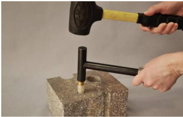
Figure 2. Installing the VAPOR PIN®
