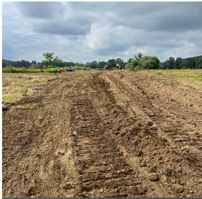
Photo 18: View facing south - completed backfilling of excavated trench
