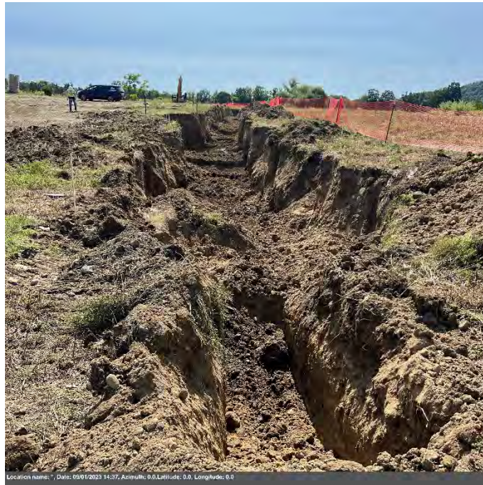
Photo 13: View facing south – excavation of trench completed
