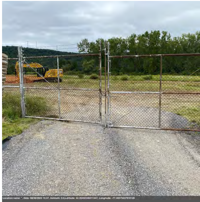
Photo 5: fencing for control access to excavation area
