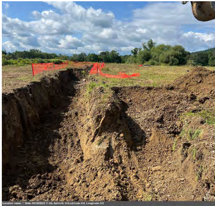
Photo 10: View facing south – excavated trench at south end
