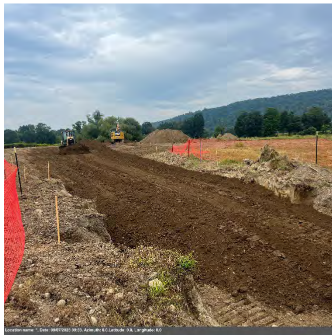
Photo 14: Backfilling of excavated trench from south end point
