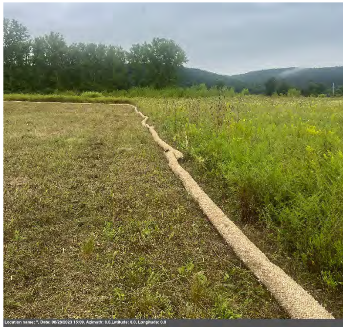
Photo 4: Straw waddles placed along perimeter of project site
