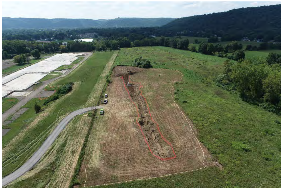
Photo 16: View facing south – overview of IRM-7 excavation
