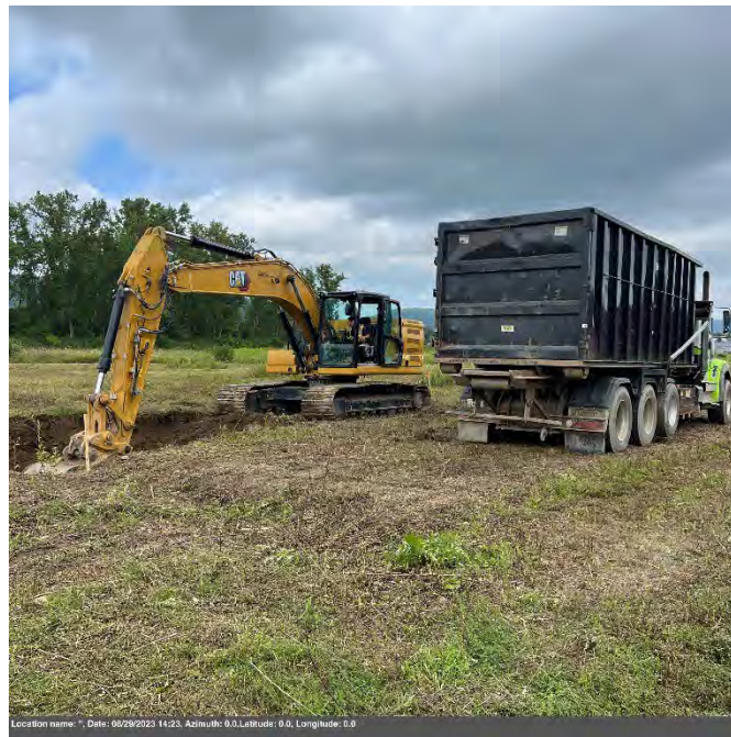
Photo 8: Direct loading of waste for off-site disposal
