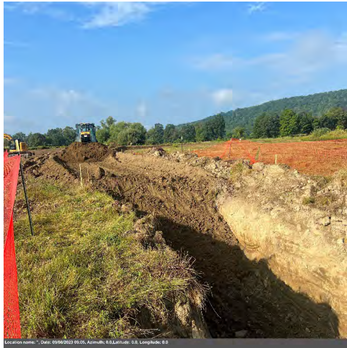
Photo 15: View facing south – backfilling of excavation at north end point
