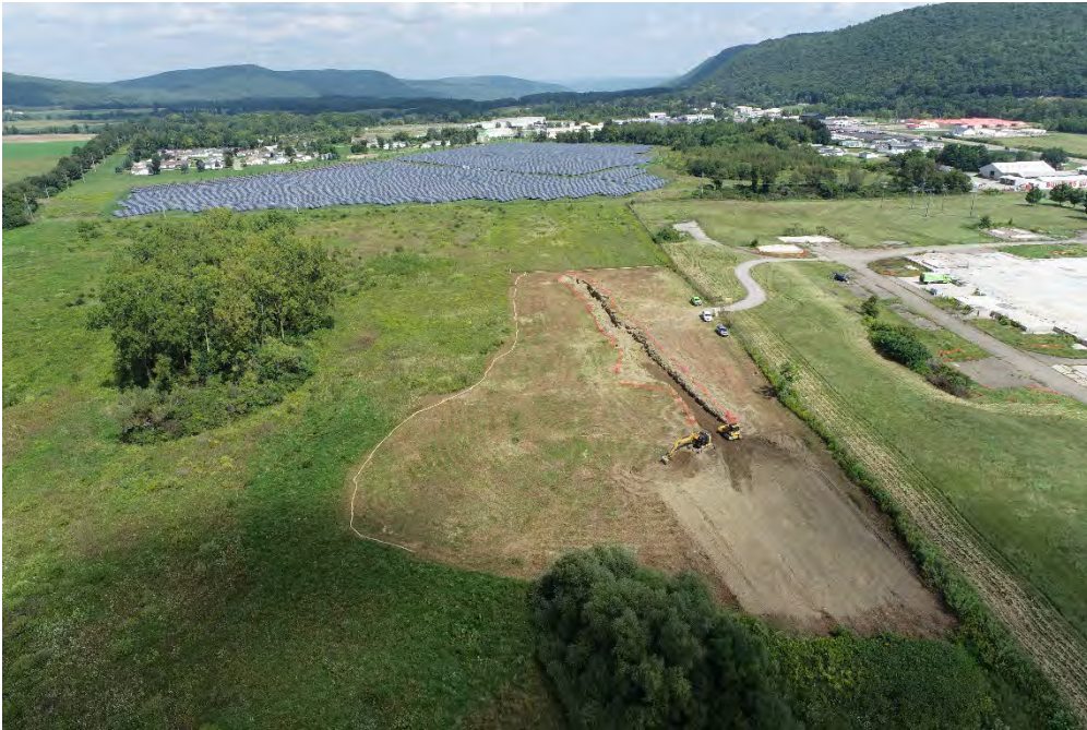
Photo 17: View facing north - overview of IRM-7 excavation
