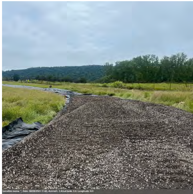
Photo 6: Construction of temporary crushed gravel roadway
