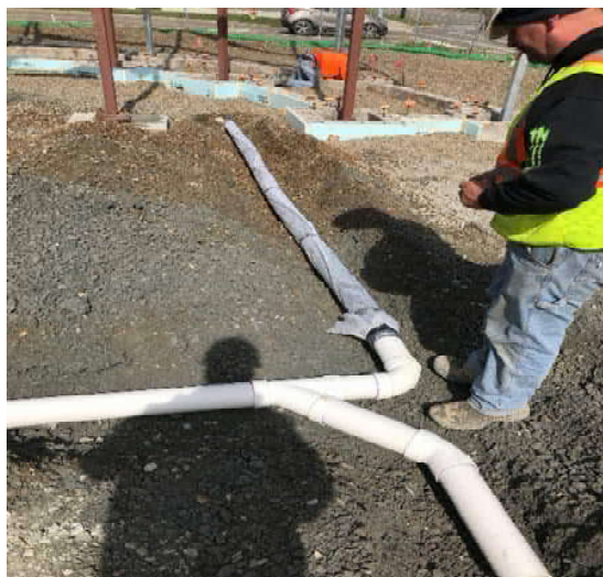
Header piping connected to perforated Building 1 4/29/19
