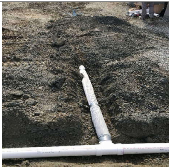
SSDS piping installed Building 1 4/29/19
