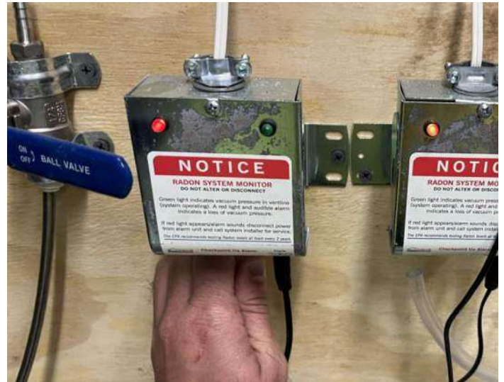
Building 2 alarms (testing alarms) 10/9/23
