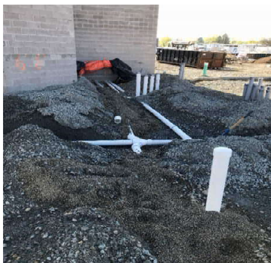
PVC header pipes being installed Building 1 4/29/2019
