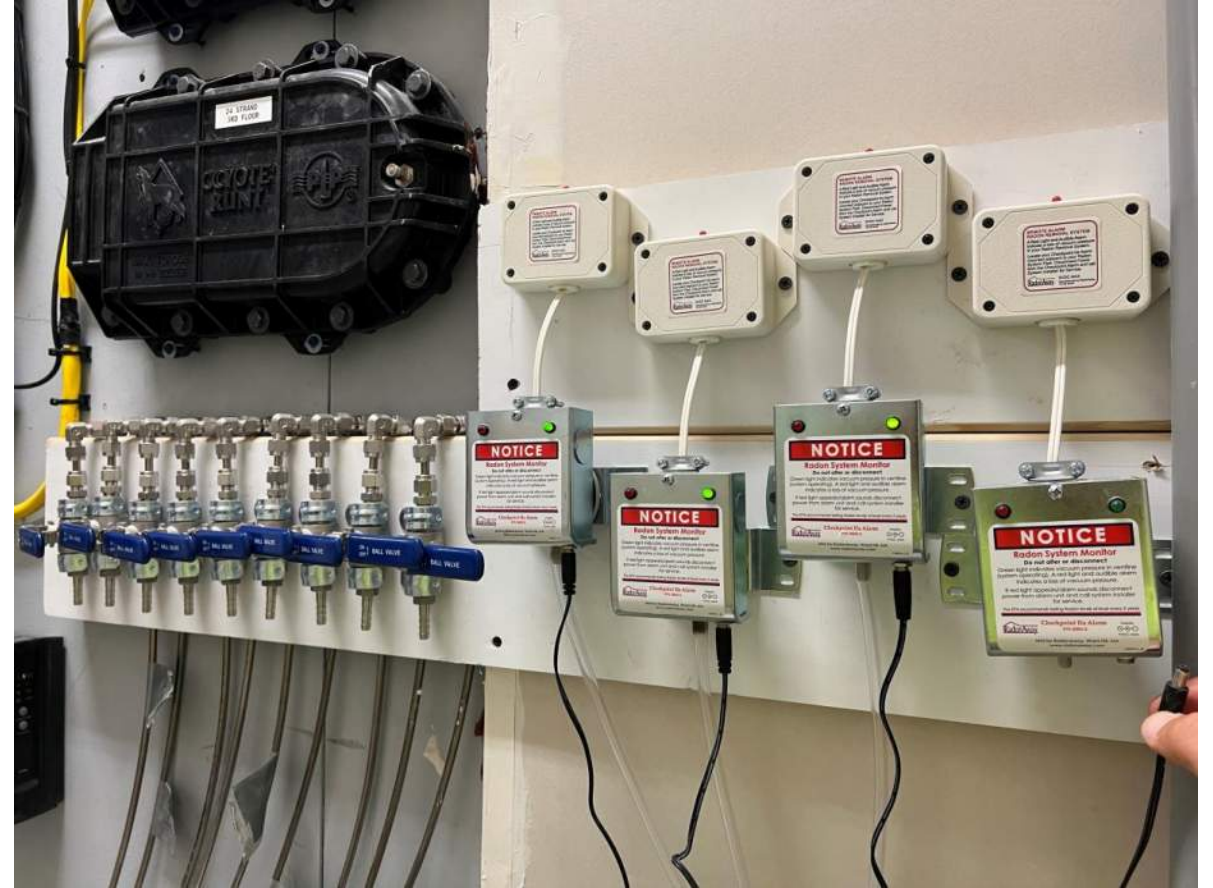
10/18/24 – Building 1 Alarms and PFE Monitoring Points
