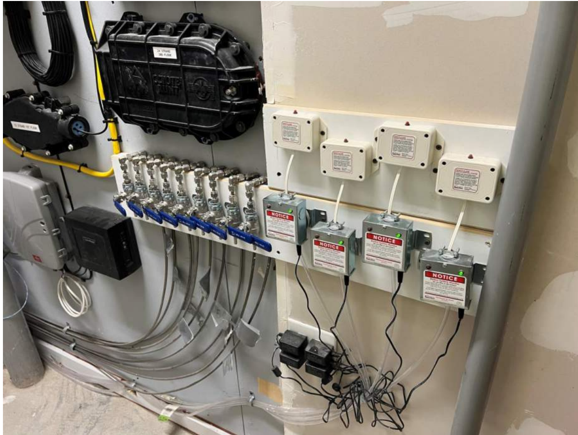
10/18/24 – Building 1 Alarms and PFE Monitoring Points
