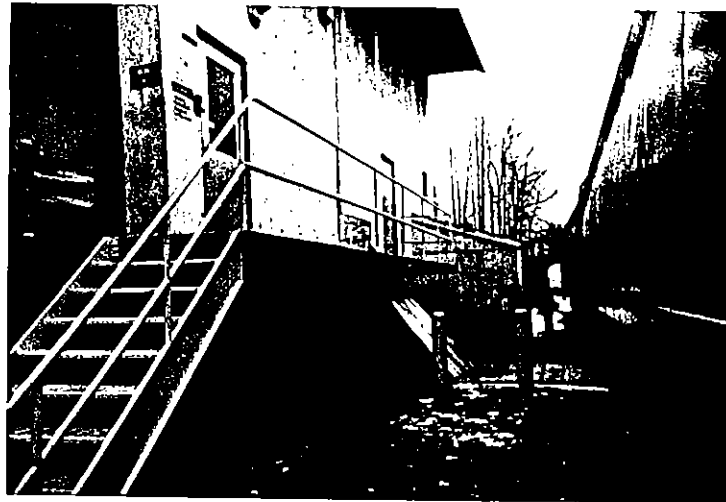
Photo 3-4. Resin Offloading Facility
