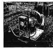
Buildings 11A-A, 11A-B, and 20 Roof Mounted Fan and Disconnect Switch
