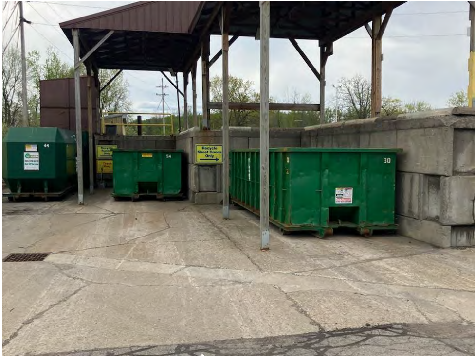
Photo 3 Representative photograph documenting various refuse and debris removed from around the trash compactor area by Garlock personnel after the PRR reporting period.
