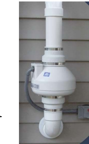
Typical exterior wall mounted RadonAway® Blower
