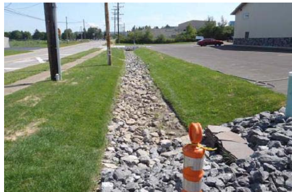
After remediation: Finished stormwater ditch along Franklin Street
