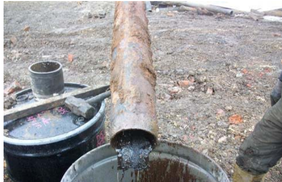
During remediation: 1,489 gallons of water/oil/tar mixture removed from the site
