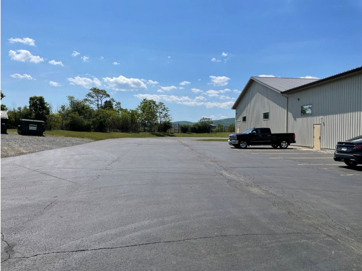
Asphalt cover conditions facing south.
