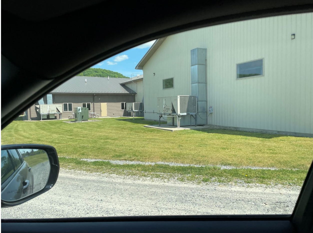
Cover/site conditions, west side of building.
