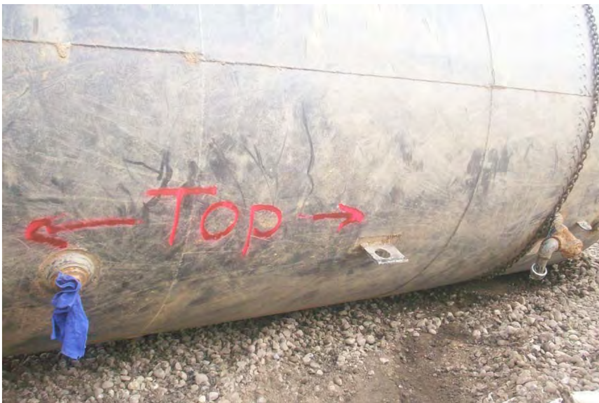
Photograph 4. Top of the tank
