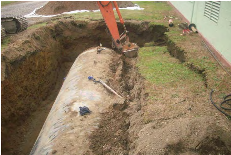
Photograph 1. Orientation of tank inside excavation area
