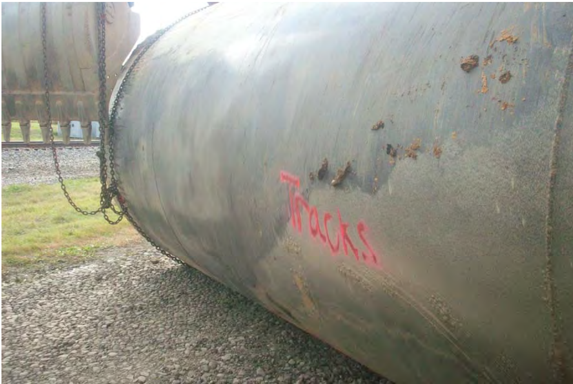
Photograph 9. Side of the tank facing the railroad tracks
