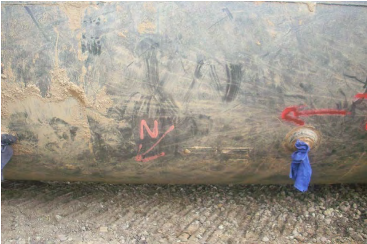
Photograph 5. North end (top) of the tank
