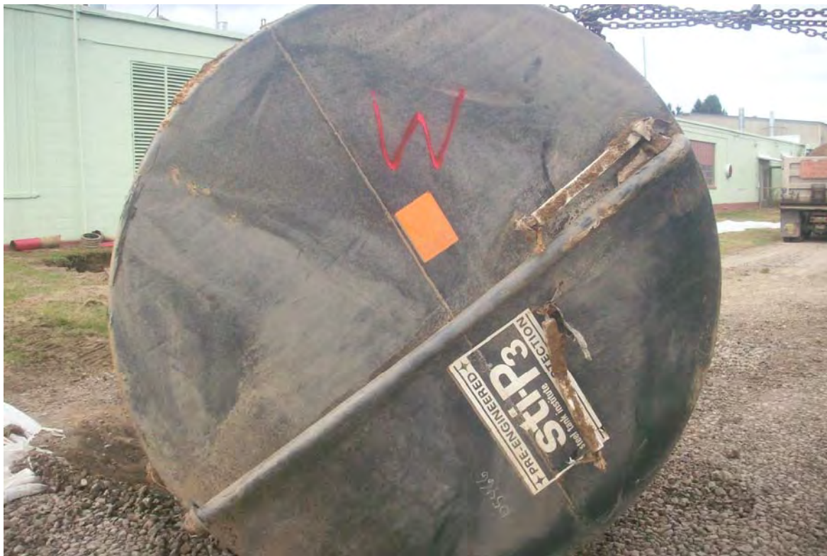
Photograph 3. West end of tank
