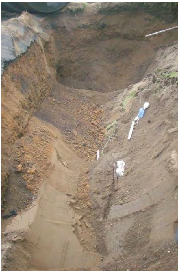
Photograph 2. Excavation area after tank removal
