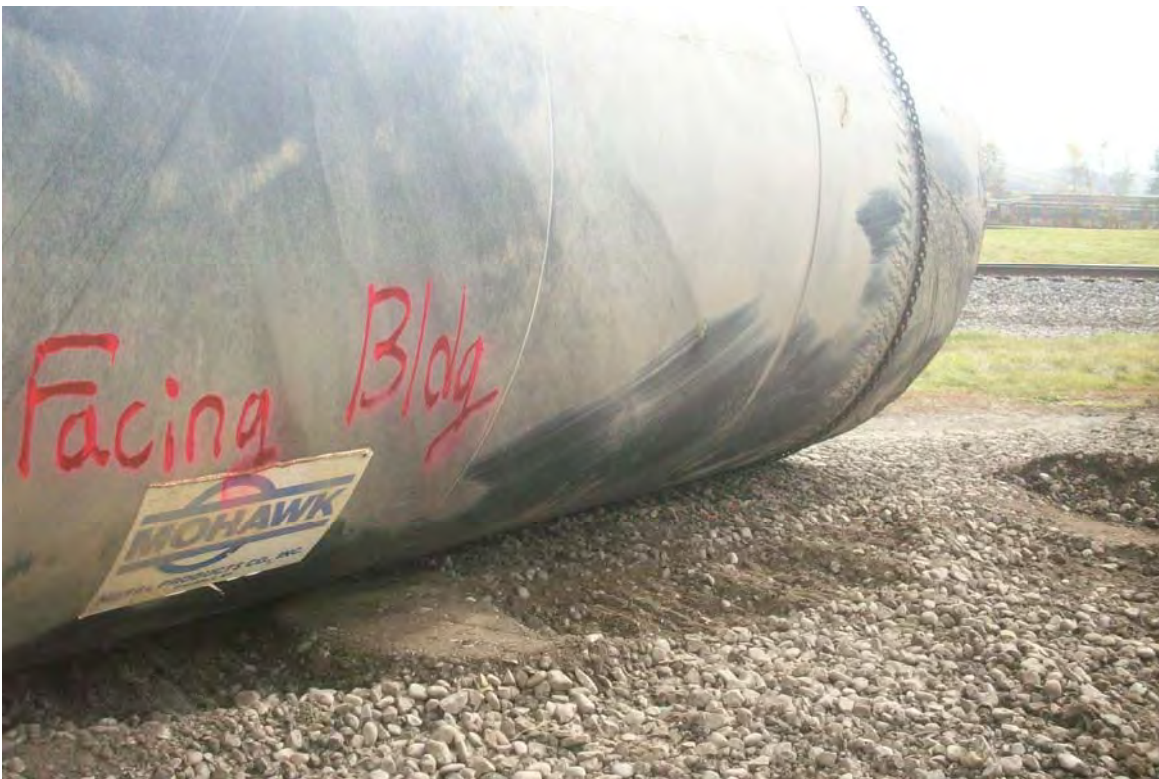
Photograph 8. Side of the tank facing the building
