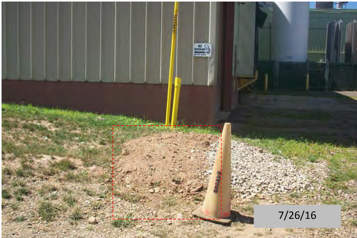
View of area at the southeast corner of the Site where erosion had degraded cover soil and was subsequently repaired with the addition of supplemental cover soil (and gravel on off-site portion)
