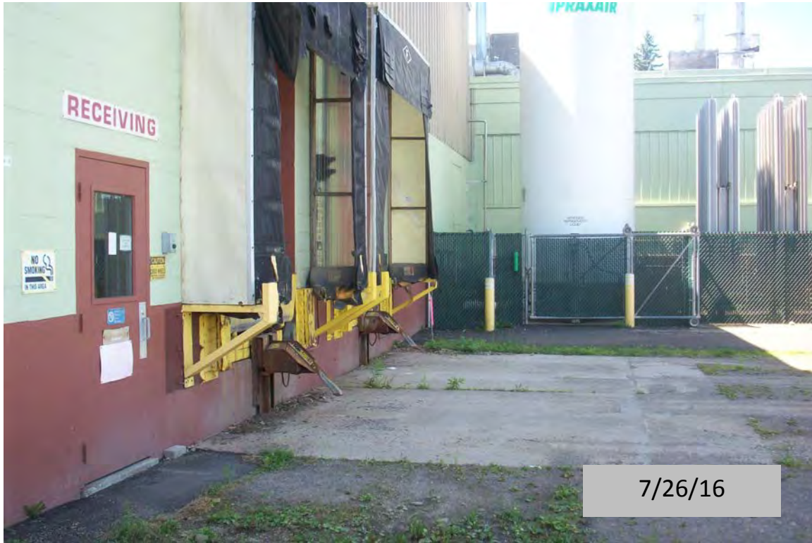
View, facing north, of the concrete/asphalt pavement cover over the receiving lot on the southeast portion of the Site
