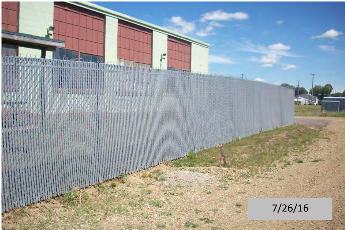
View, facing southeast, of the soil cover over the southwest portion of the Site
