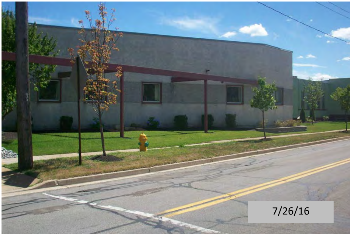
View, facing southwest, of the soil cover over the northern edge of the Site
