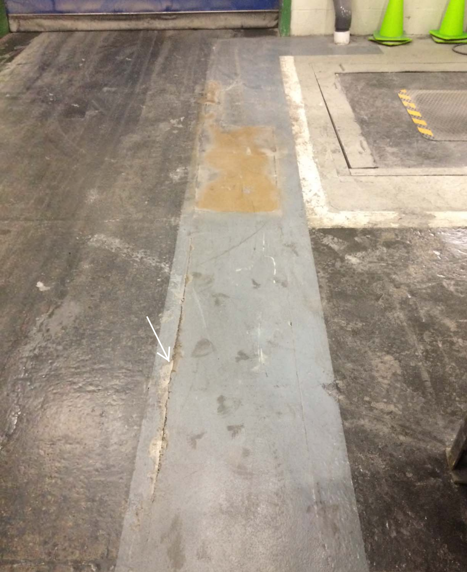
Typical view of minor cracking/settlement at edge of concrete patch over SSDS, located in the Packaging Department of the facility building, facing south.
