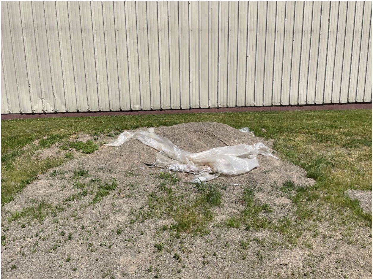
Stockpile of pea gravel for driveway repairs.
