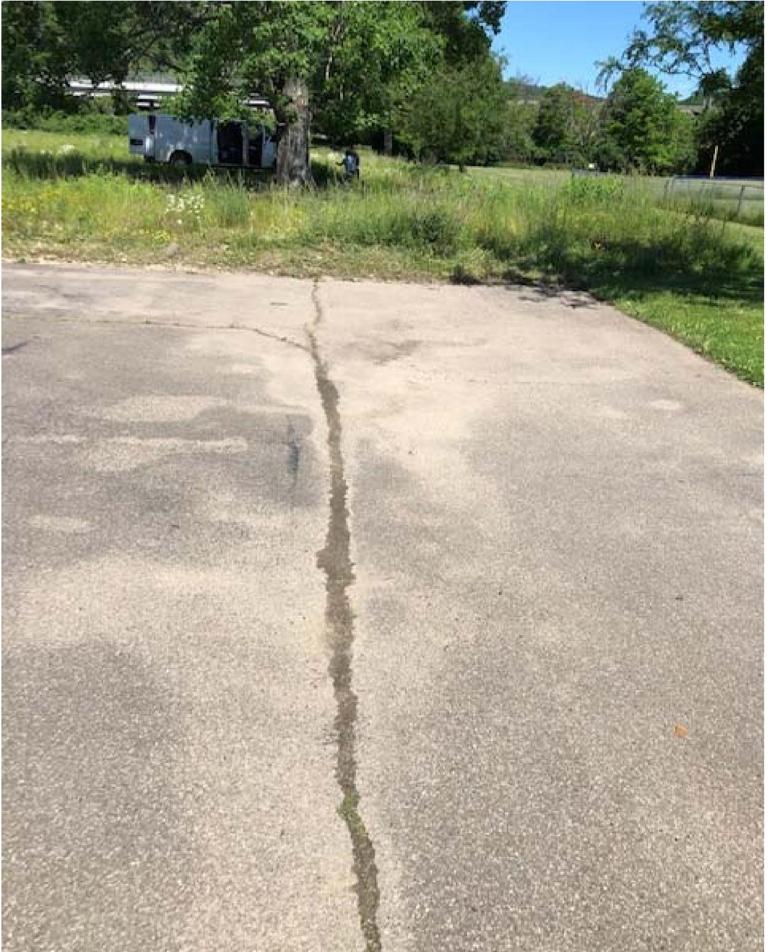
View of repaired asphalt cover located on the eastern portion of the Employee Parking Lot, facing northwest. View of groundwater monitoring event at monitoring well MW-E, amid the soil/vegetative cover and mulch cover (below visible tree) at top of photo.
