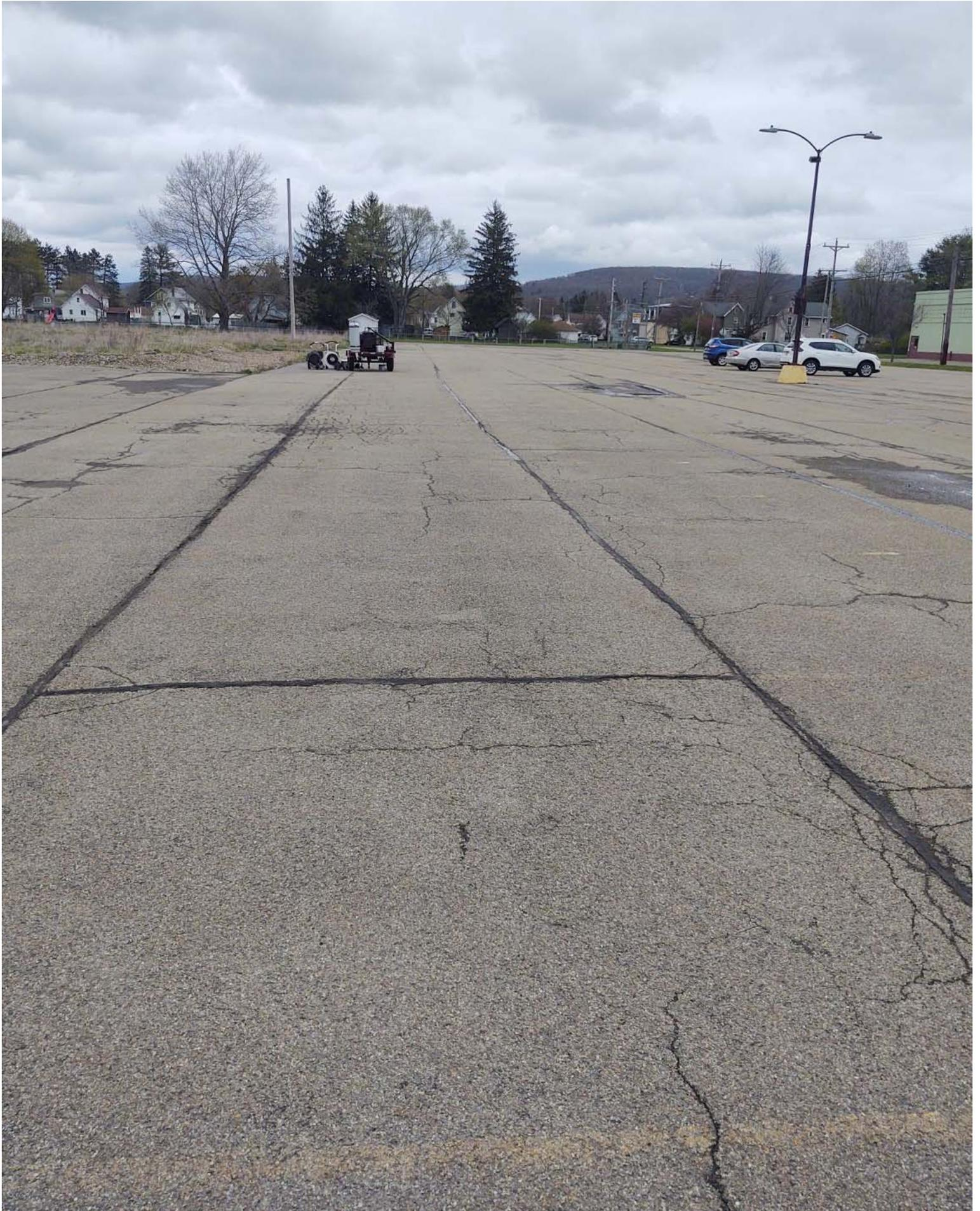
Partial view of the Employee Parking Lot at 202 Franklin St., taken on May 2, 2022, depicting repairs made to the cracks in the asphalt pavement, and Carter Blacktop's equipment that was used to make the repairs, facing east.
