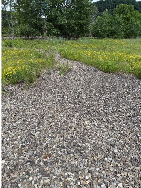
Partial view of the drainage channel stone cover (foreground) and vegetated soil cover (background) located in the central-western portion of the Site, facing northwest.
