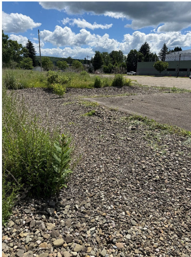
Partial view of the drainage channel stone cover (foreground) and asphalt pavement cover (background) located in the central portion of the Site, facing southeast.
