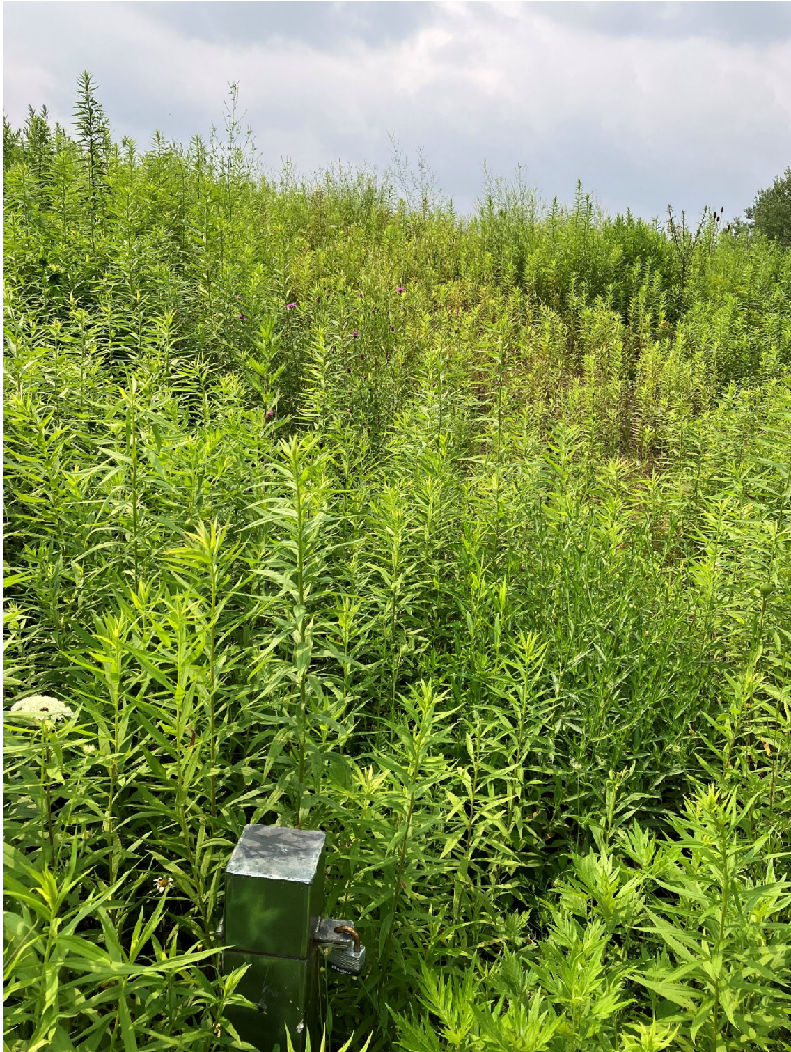
Representative view of a monitoring well protective casing, equipped with padlock (MW-C - foreground) with vegetative cover over a soil mound (background), facing southwest.
