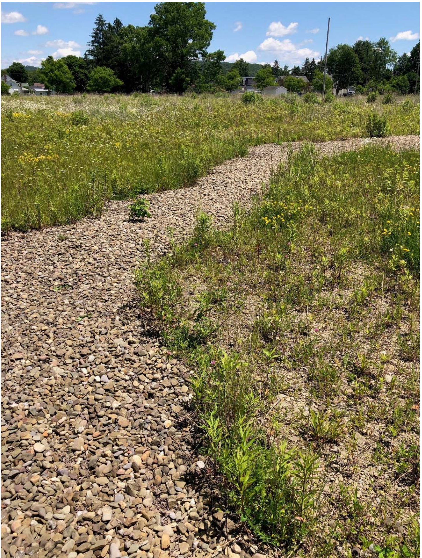
View of a portion of the drainage swale and adjoining soil cover, located on the northwestern portion of the Site, facing east.
