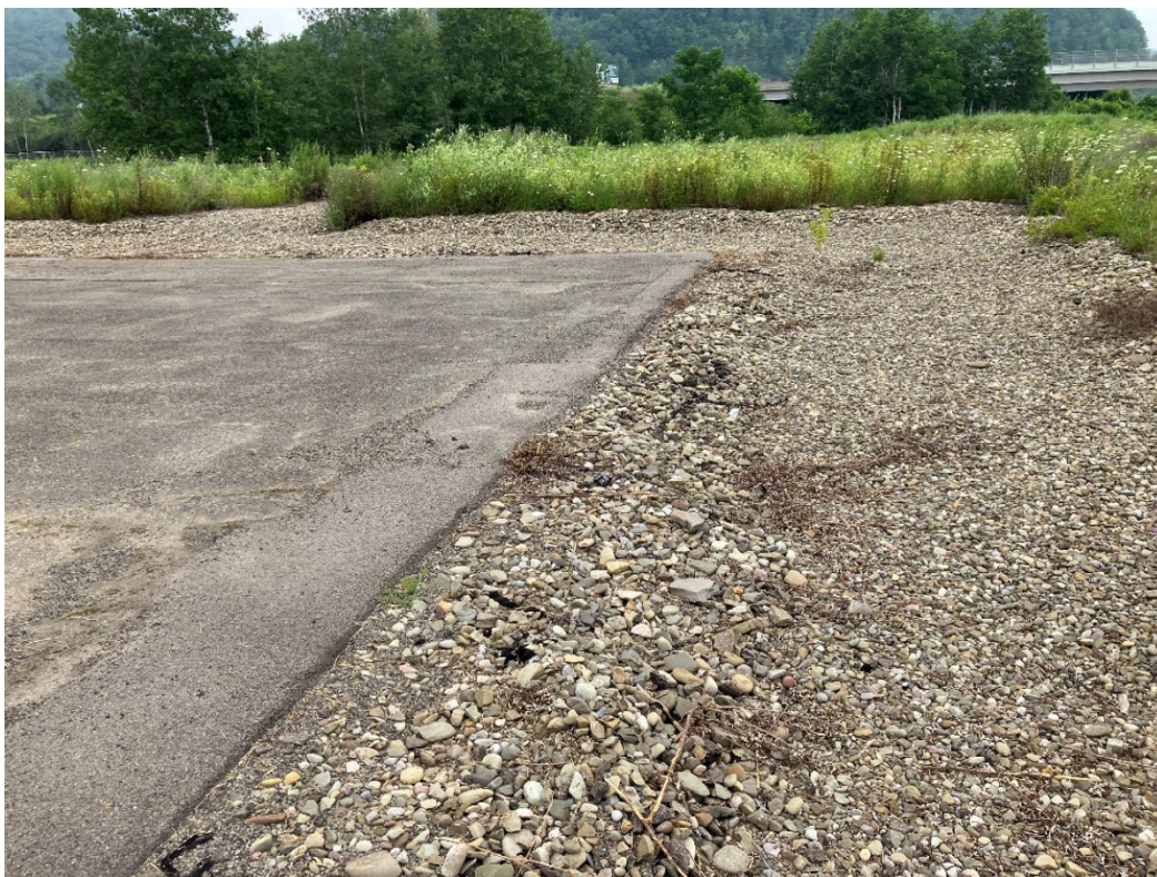
View of a portion of the drainage channel stone cover located along the northern edge of the parking lot, facing north.
