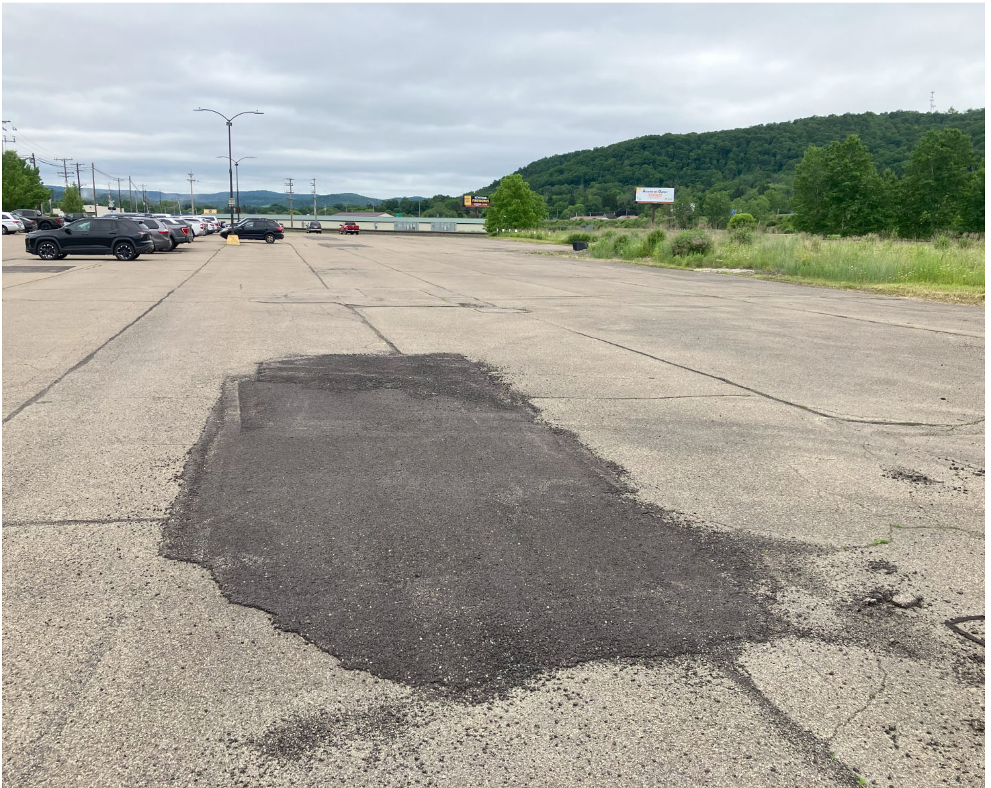
View of an area of repaired asphalt cover (completed October 2024), located on the eastern portion of the asphalt-paved parking lot, facing west.
