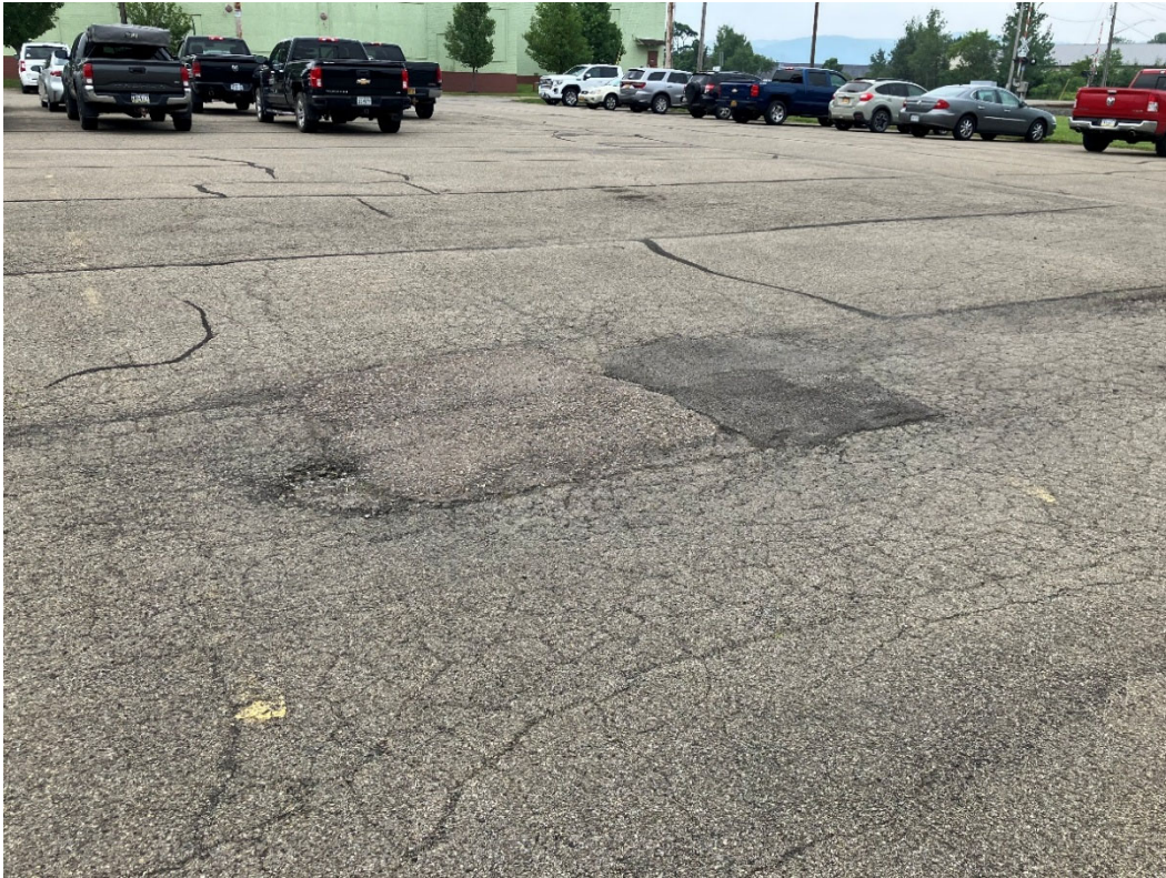
View of the western-central portion of the asphalt pavement cover, with older repairs (i.e., sealant along cracks and asphalt patches) visible, facing southwest.
