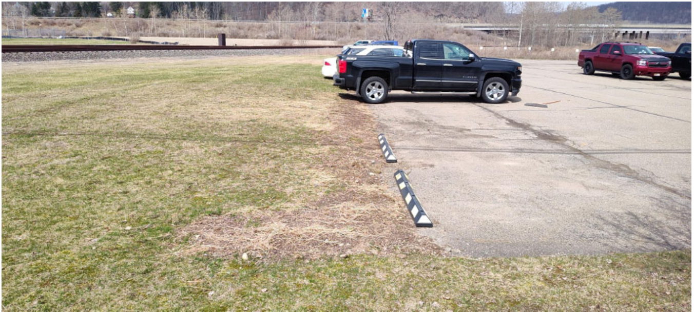
View of the repaired area of soil cover located near the southwestern edge of the Employee Parking Lot, facing north.
