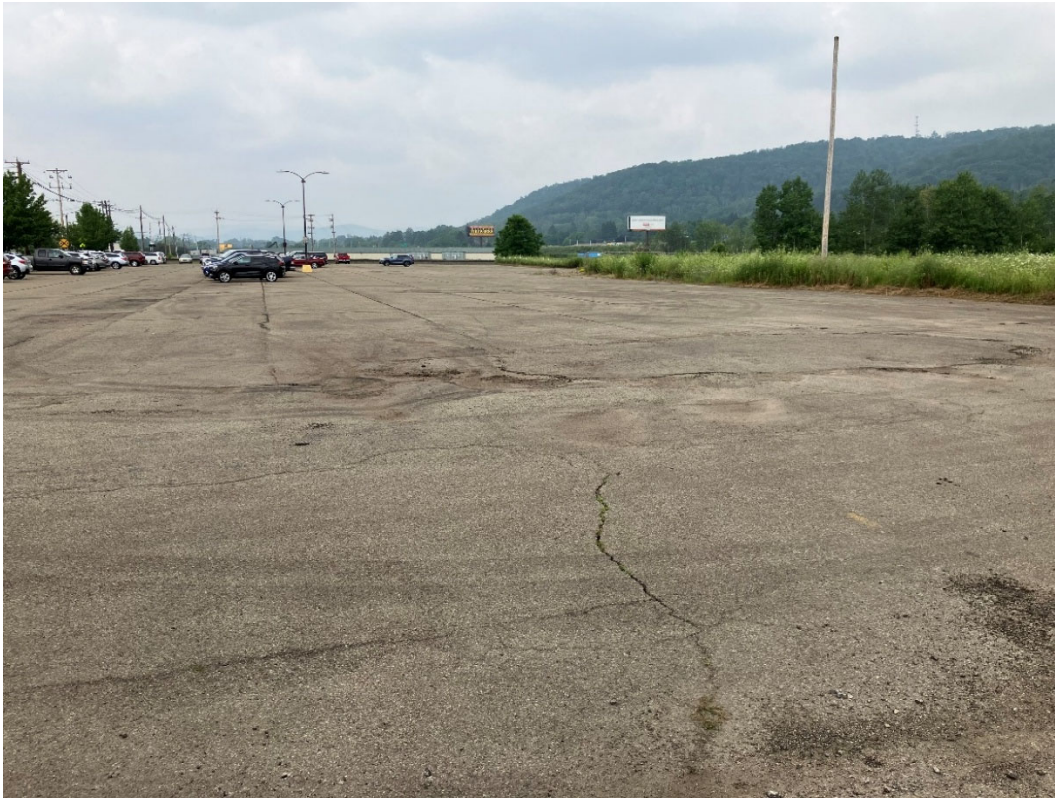
View of the eastern-central portion of the asphalt pavement cover, facing west.
