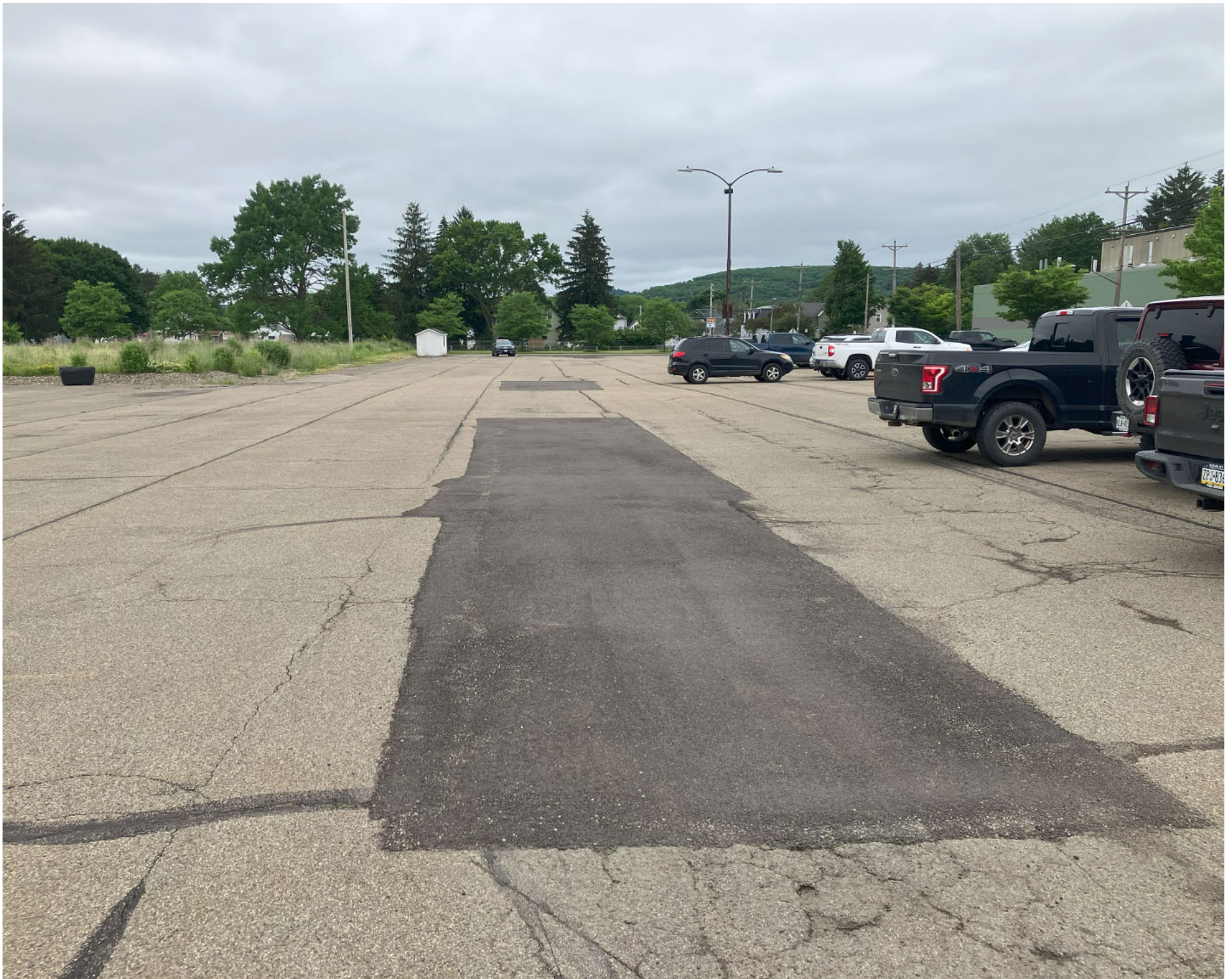
View of an area of repaired asphalt cover (completed October 2024), located on the central portion of the asphalt-paved parking lot, facing east.
