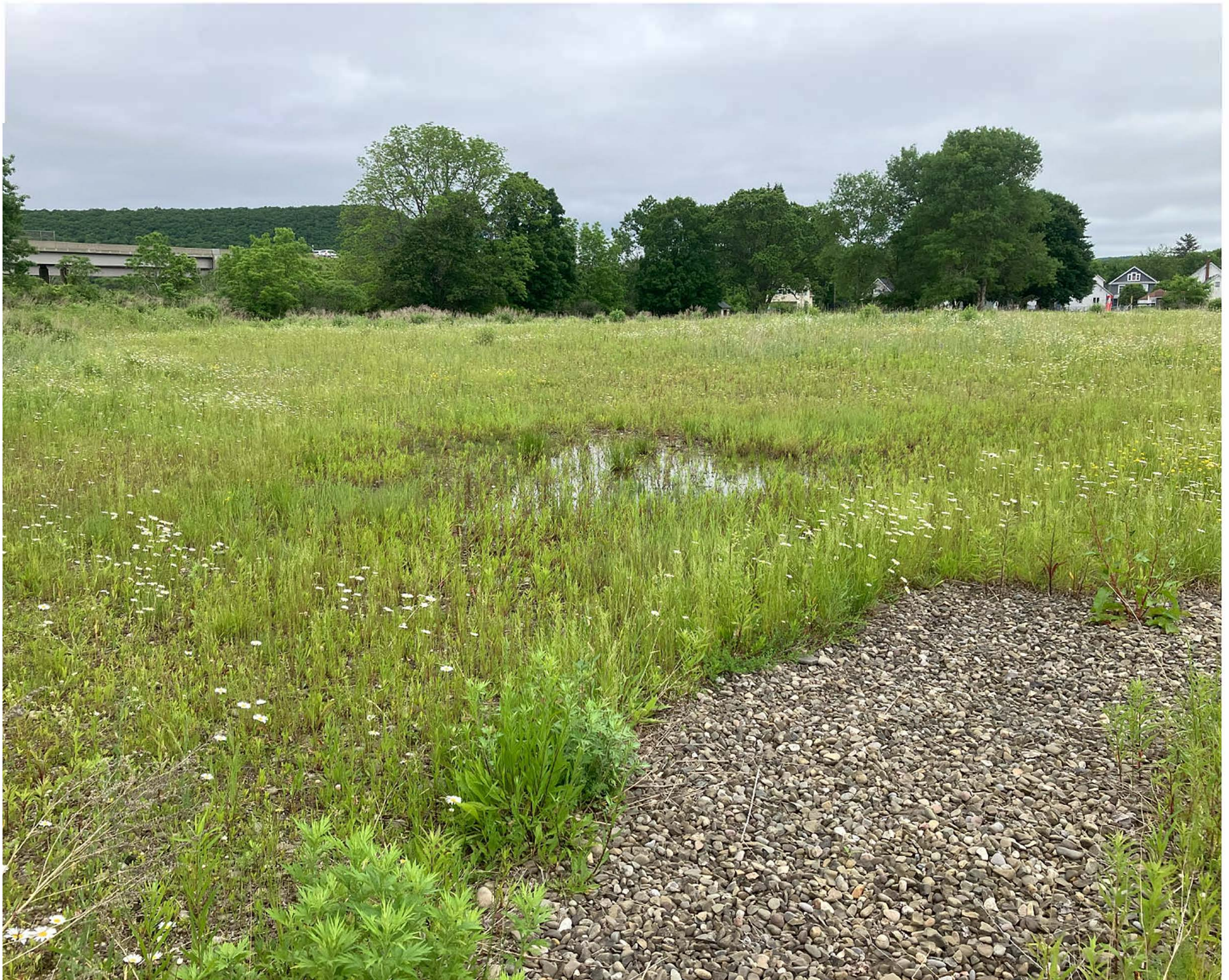
View of a portion of the drainage channel stone cover (foreground and right) with the area of standing water behind, facing north.
