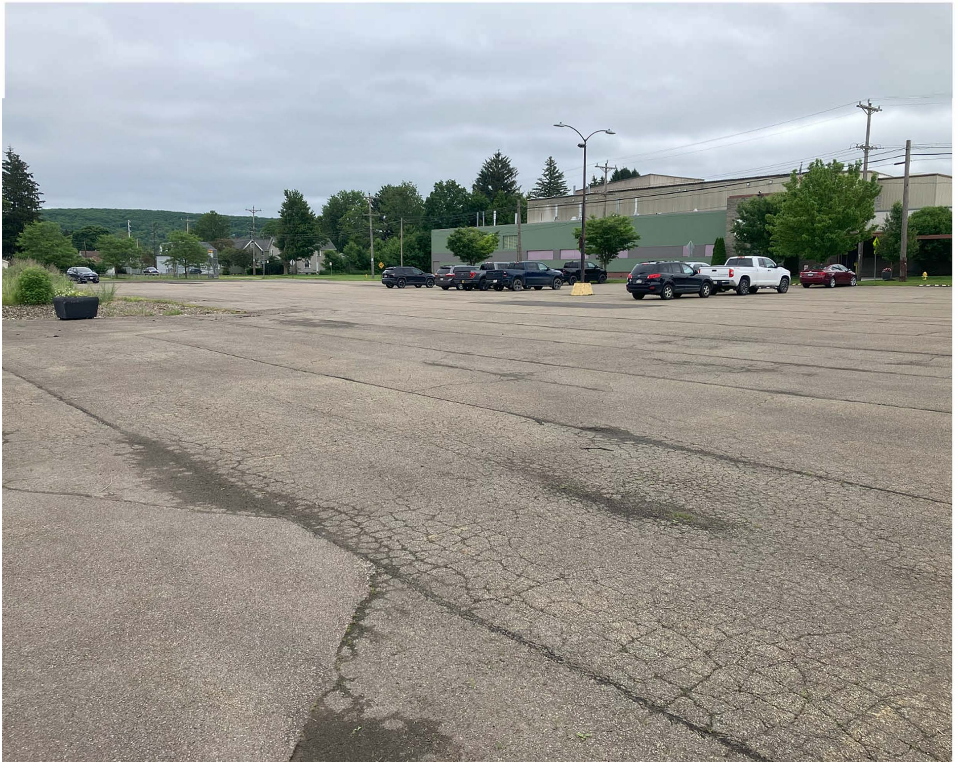
View of the central portion of the asphalt pavement cover facing south.
