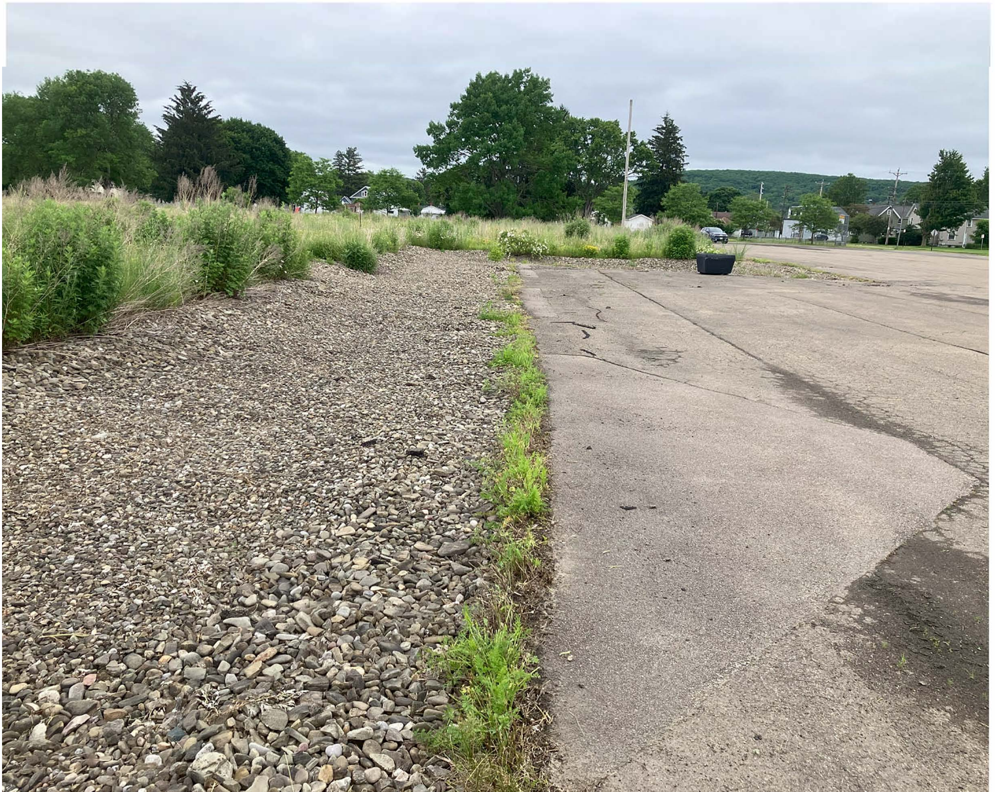
View of a portion of the drainage channel stone cover located along the northern edge of the parking lot, facing east.
