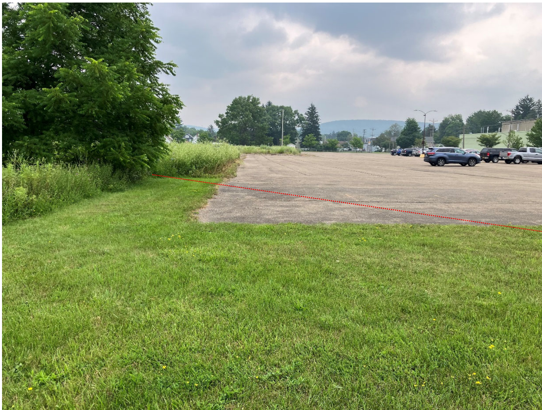
View of the western portion of the asphalt pavement cover (right) and soil cover (left), facing east. The approximate Site boundary is depicted by a dash line.
