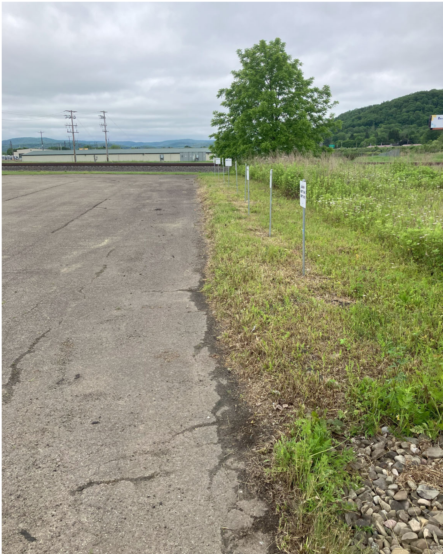
View of soil cover (right) and asphalt cover (left) along the northwestern edge of the parking lot, facing northwest.
