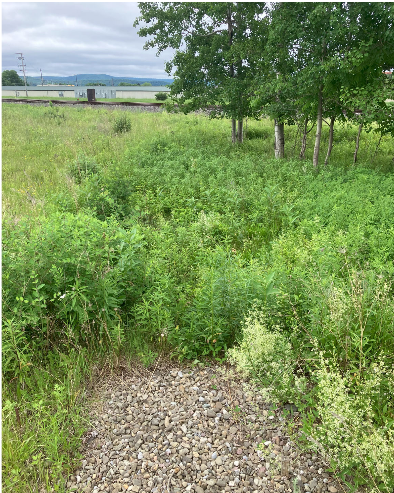
View of the northern terminus of the drainage channel stone cover (foreground), with soil cover beyond, facing northwest.
