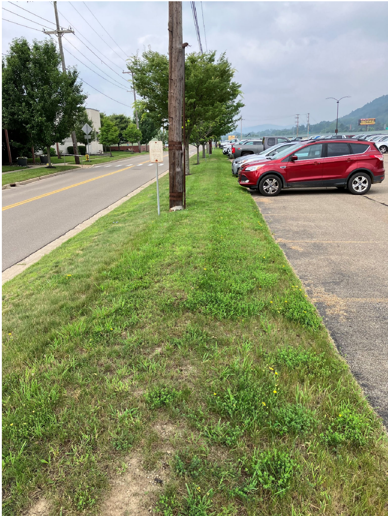
View of asphalt cover (right) and soil cover (left) along the southern edge of the eastern portion of the parking lot, facing west.
