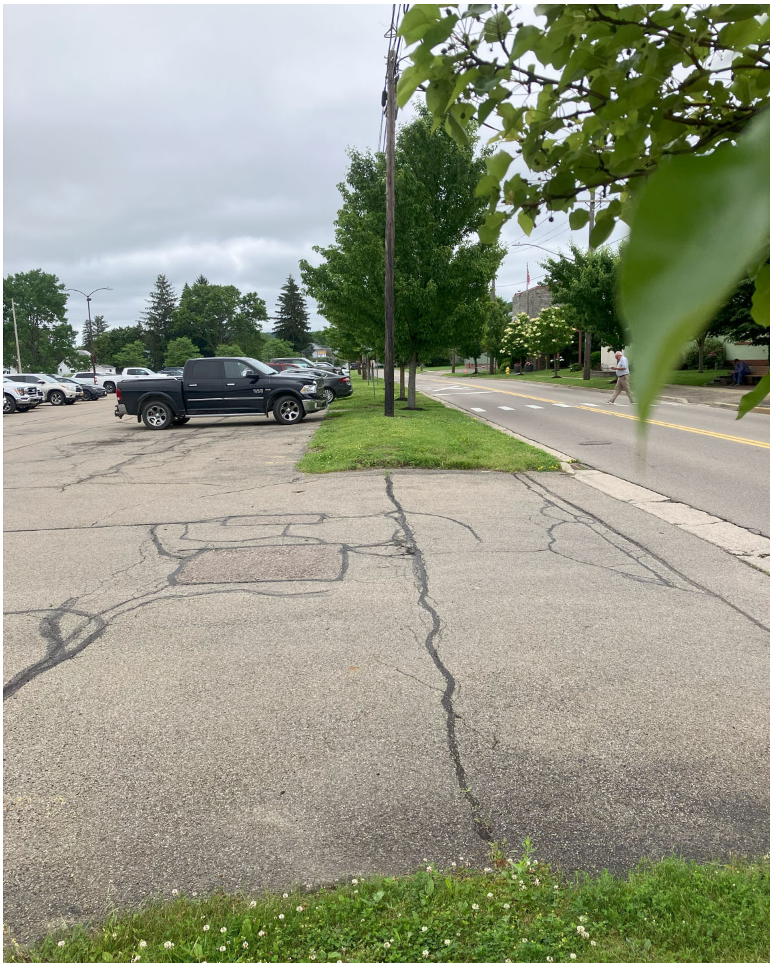
View of asphalt cover (foreground and left) and soil cover (background -center) along the southern edge of the western portion of the parking lot, facing east.
