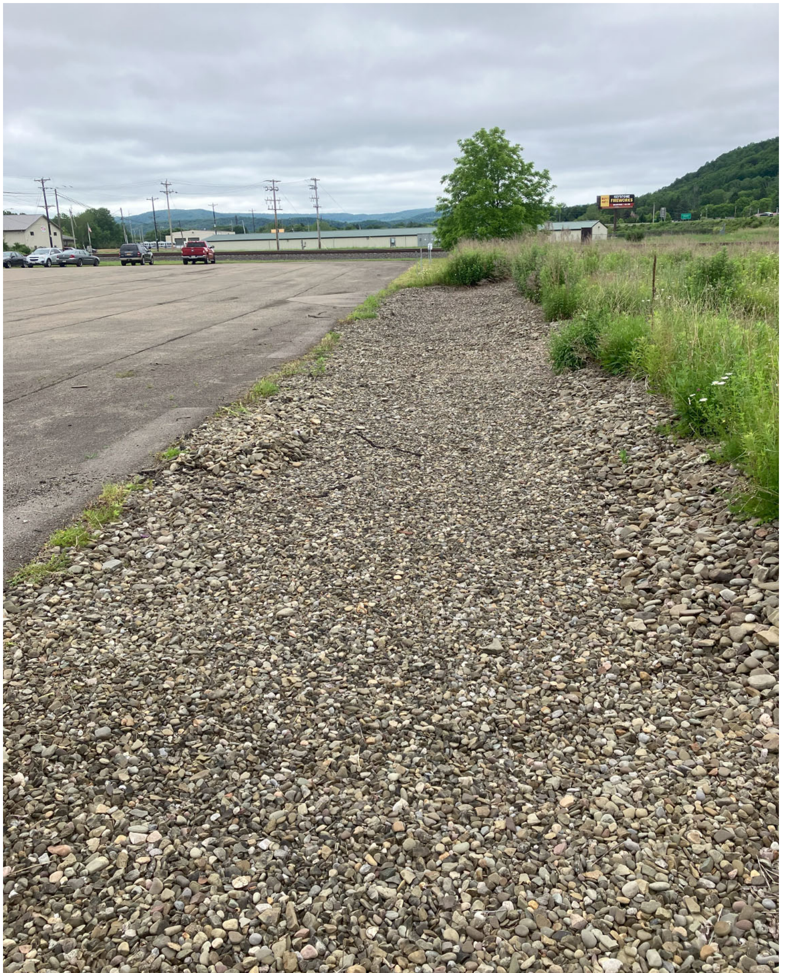
View of a portion of the drainage channel stone cover located along the northern edge of the parking lot, facing west.
