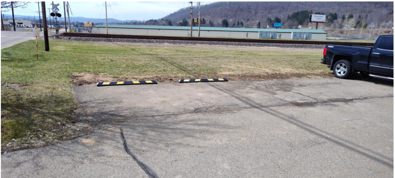
View of the repaired area of soil cover located near the southwestern edge of the Employee Parking Lot, facing west.
