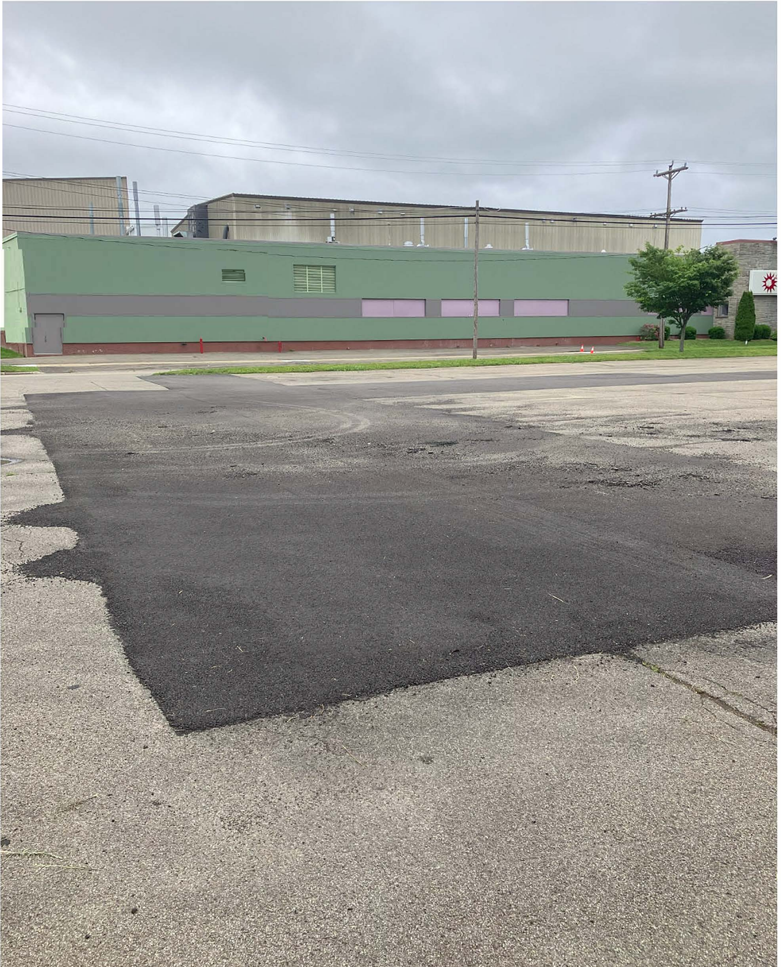
View of an area of repaired asphalt cover (completed October 2024), located on the eastern portion of the asphalt-paved parking lot, facing south.
