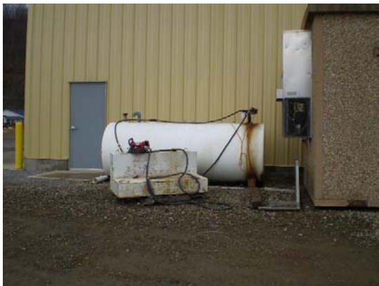
AST located along southwestern wall of Site building
