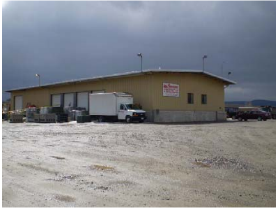
Site looking south
