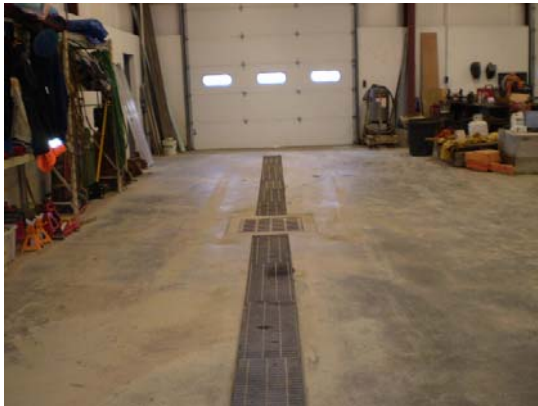
Wash bay within the warehouse/storage area of the Site building
