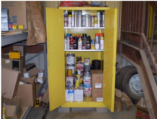
Flammable storage cabinet within the warehouse/storage area of the Site building
