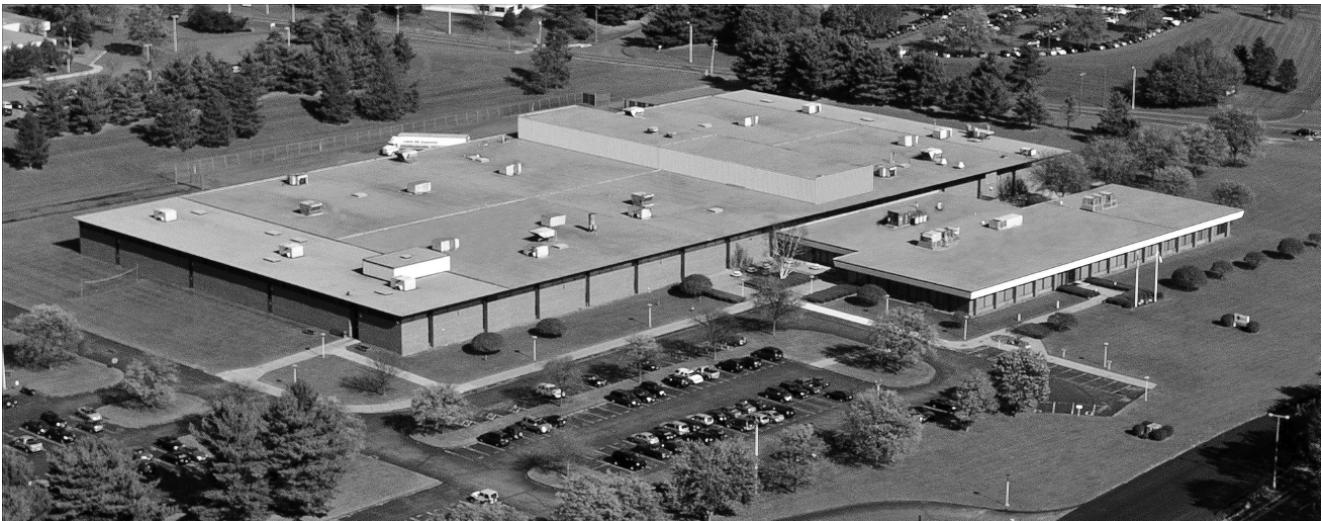
Spencer Corporate Headquarters and Manufacturing Plant, Windsor, CT USA
