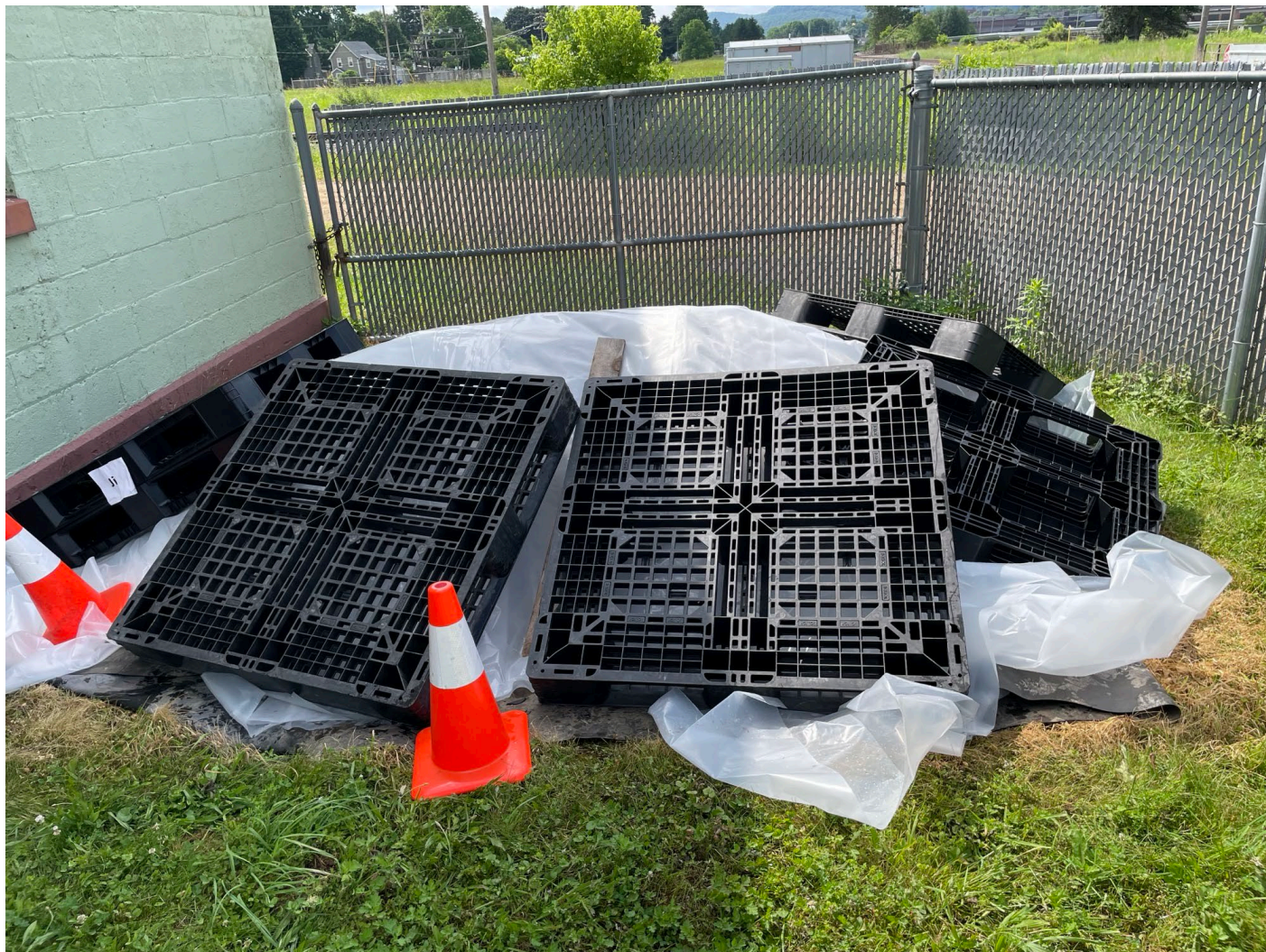
Covered spoils stockpile. Disposal pending completion of trenching work.
