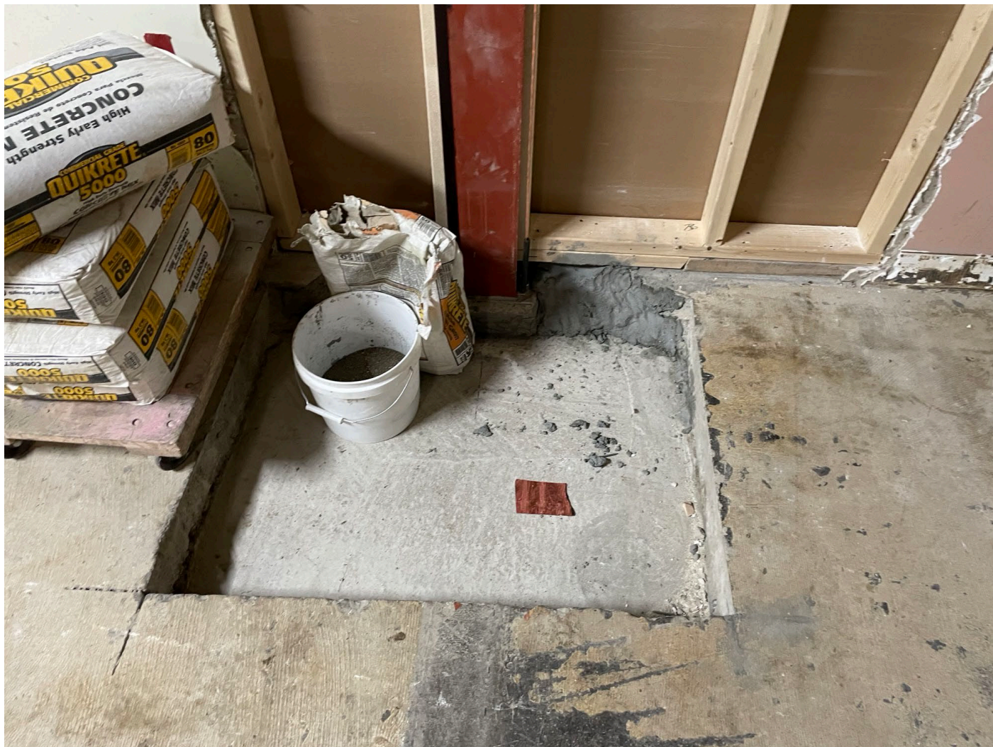
Conference room excavation that will eventually be filled with concrete to grade. Slab may or may not be penetrated to install additional electrical conduit.
