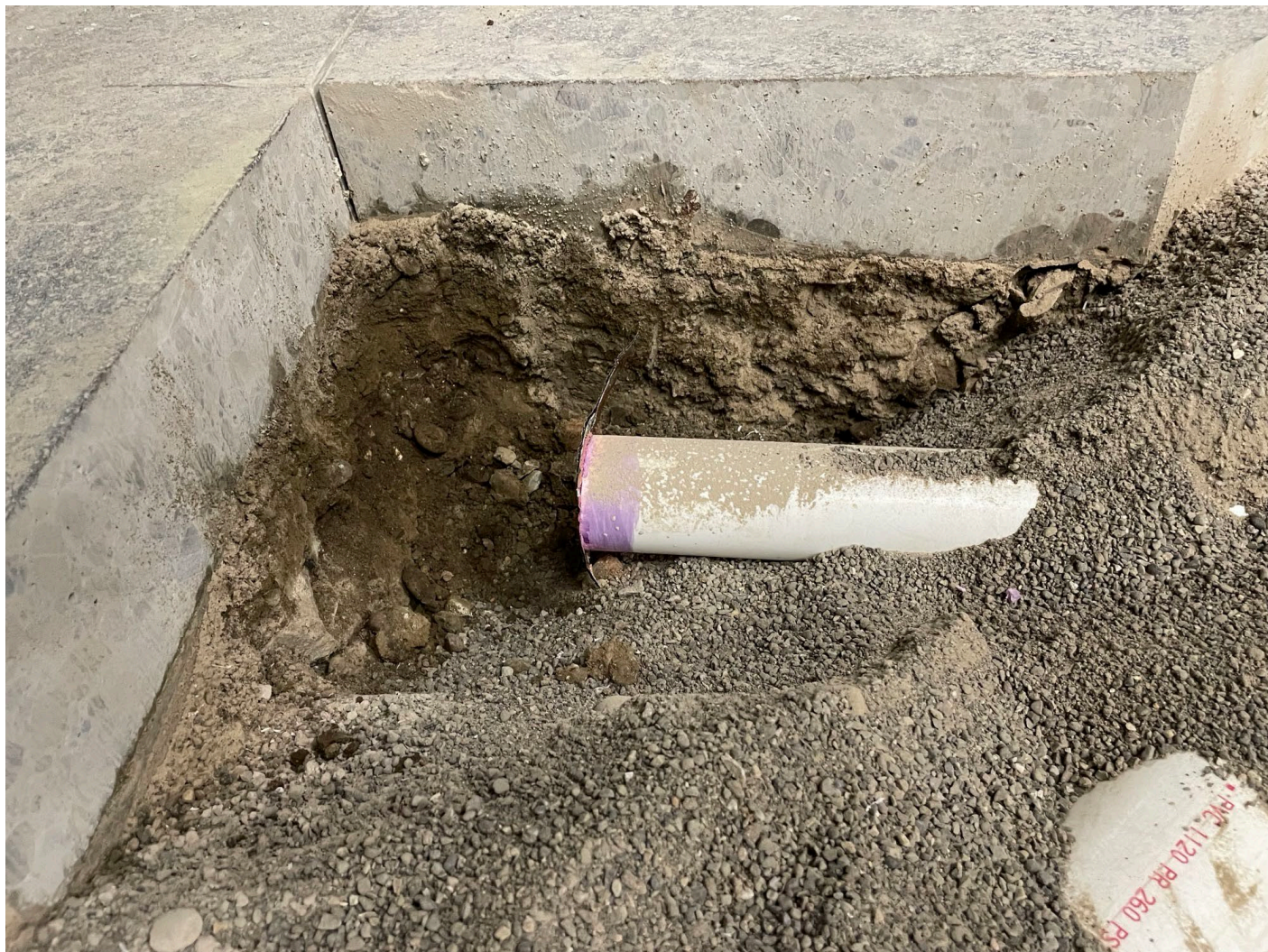
Trench/utility line with imported sand/gravel and native soil.
