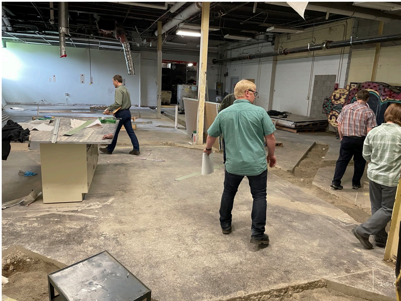
Locker room trench conditions backfilled with approved imported sand.
