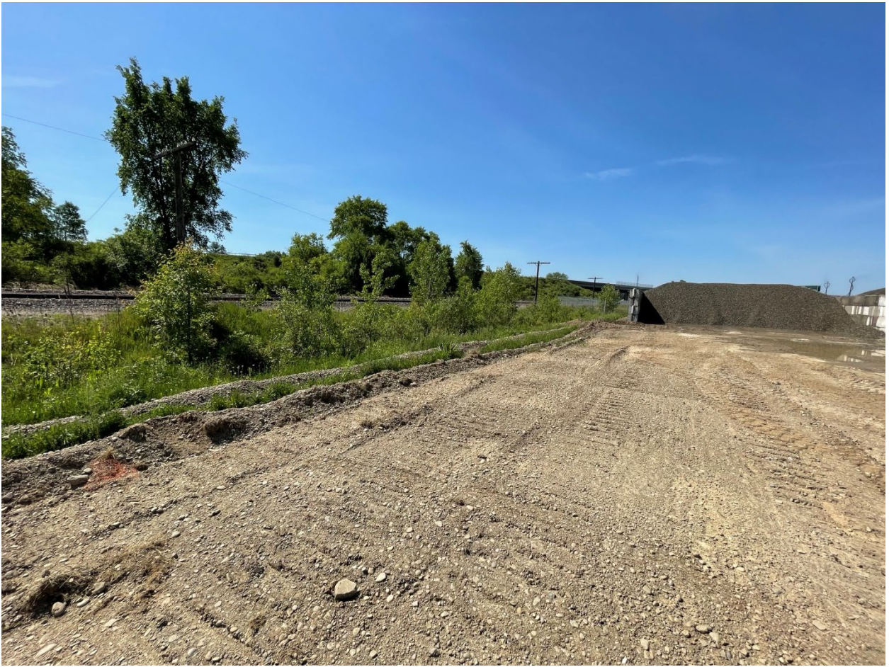
Silt berm/southeastern site conditions.
