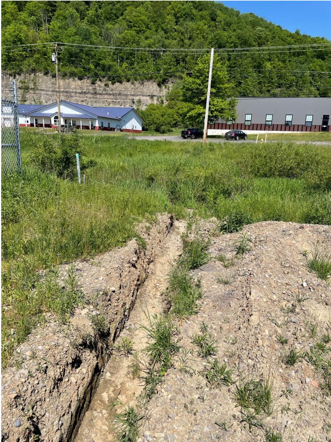
Onsite trench view is facing WNW.
