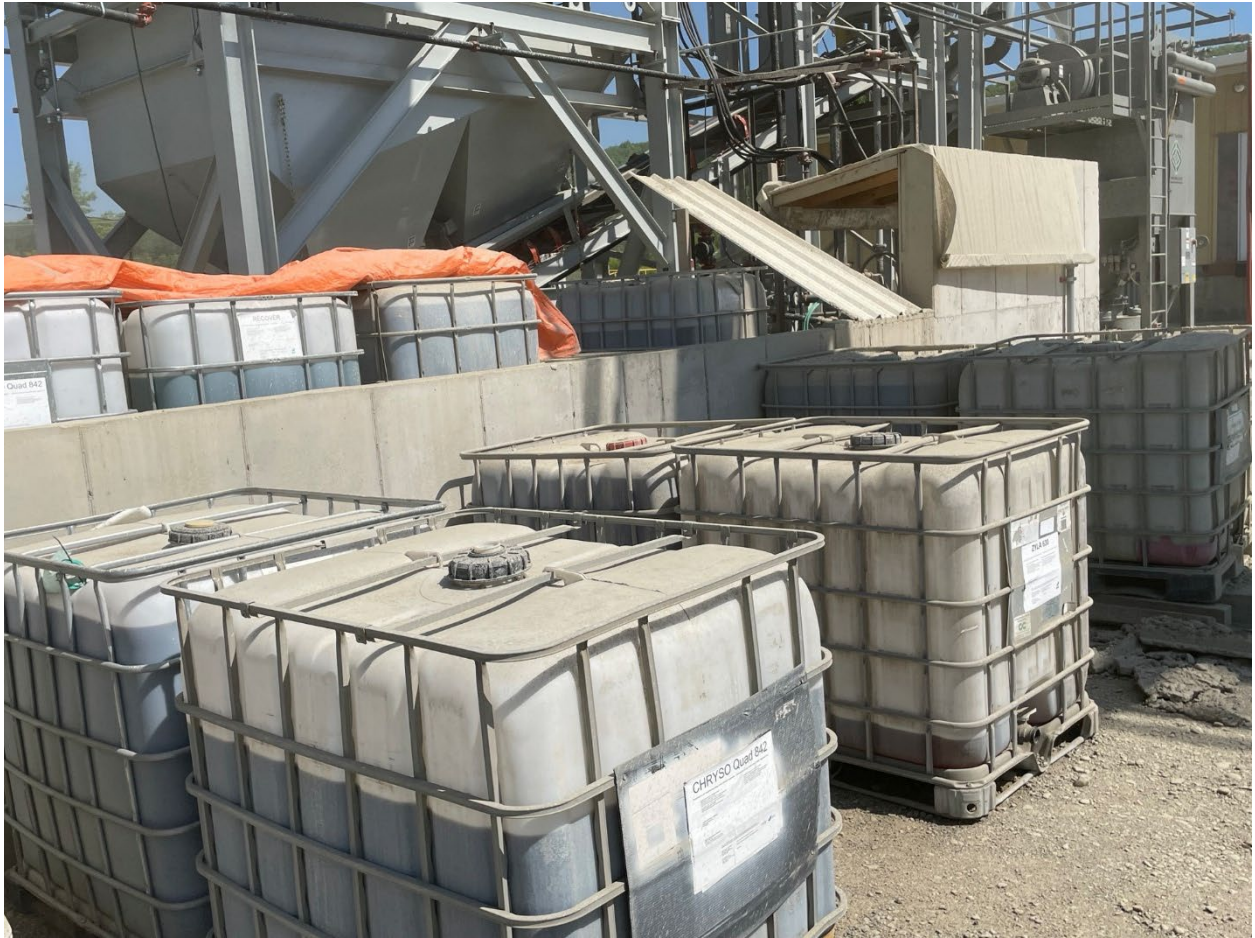
Onsite chemical storage.
