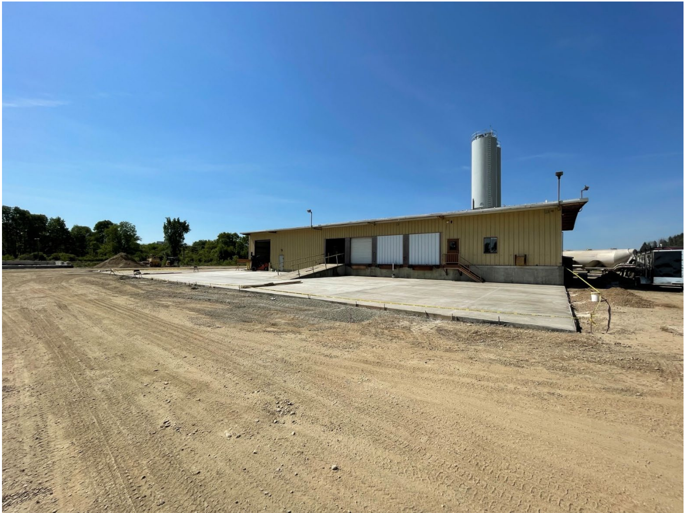
Concrete pad/northeastern site conditions.
