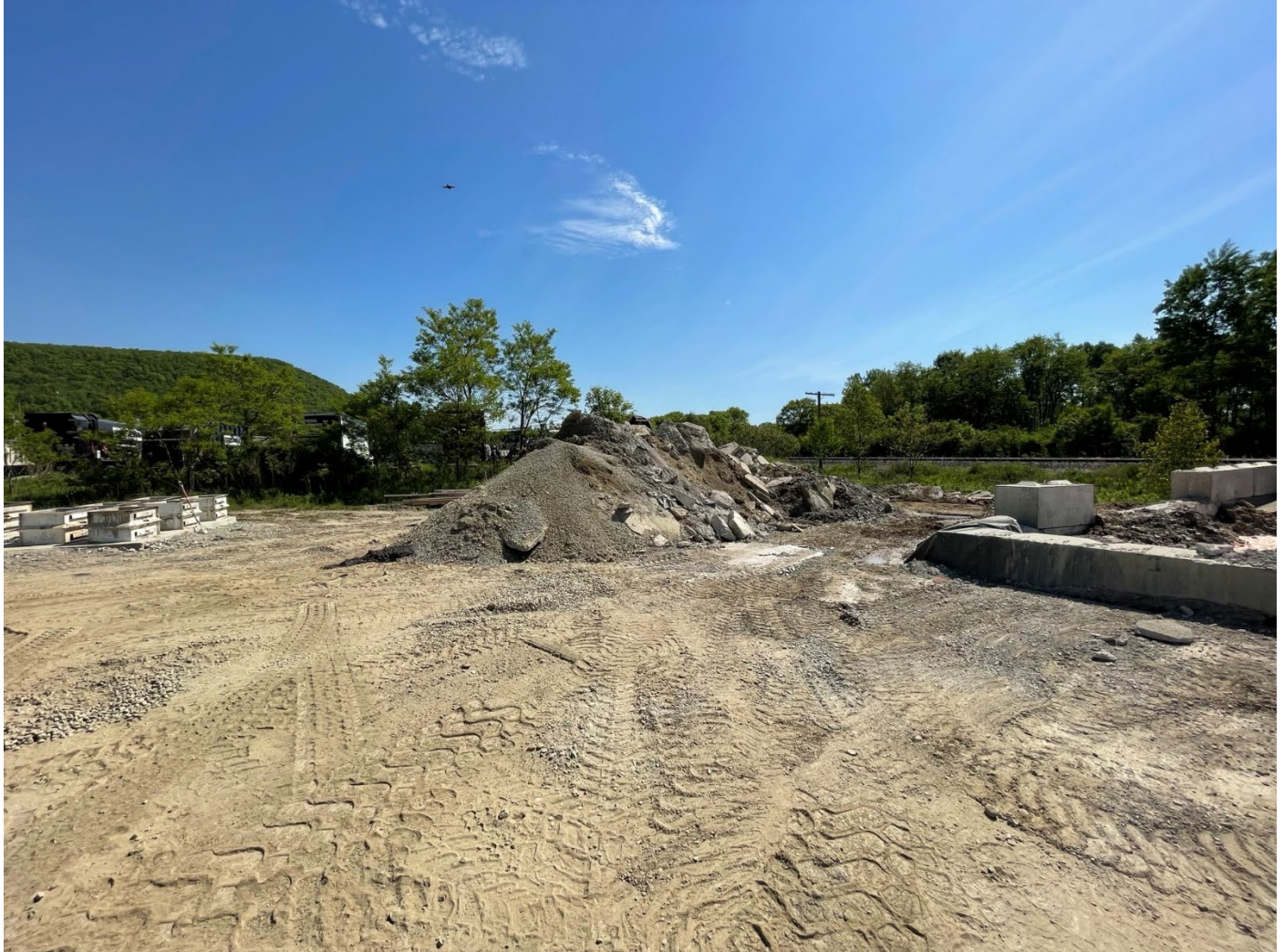
Uncovered soil pile, presumably from concrete pad excavation.
