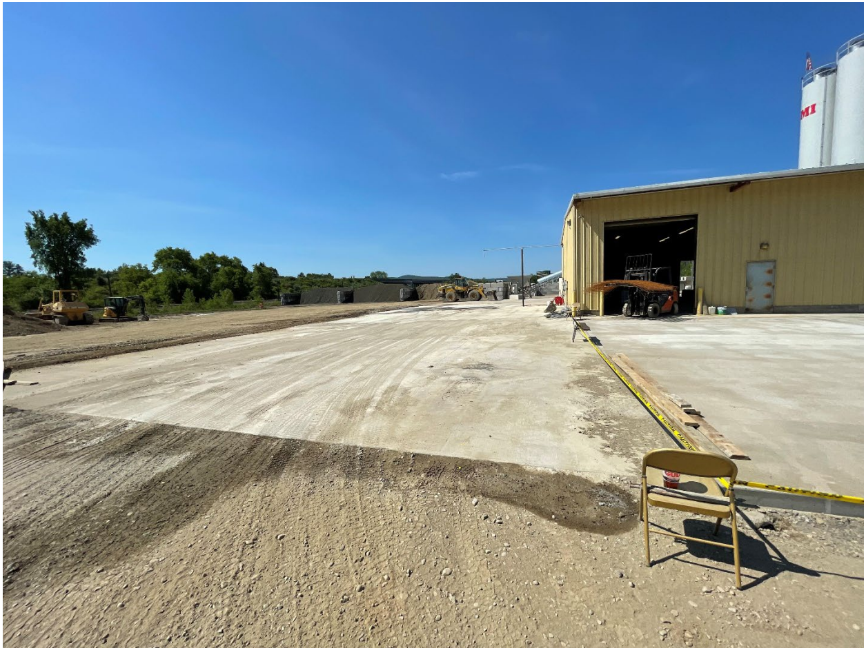
Extended concrete pad/site conditions facing SSW.
