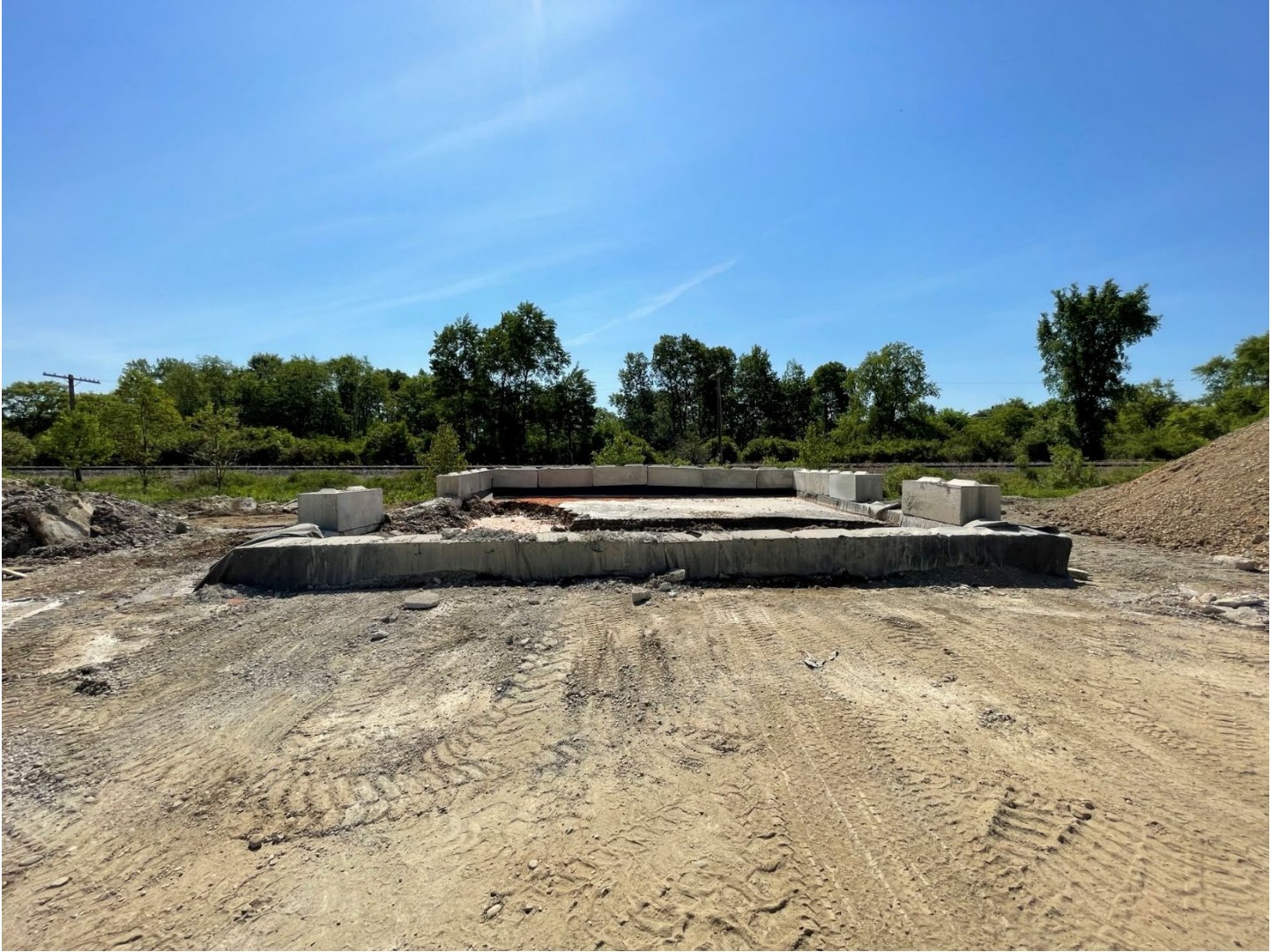
Material storage pad, eastern corner of site.
