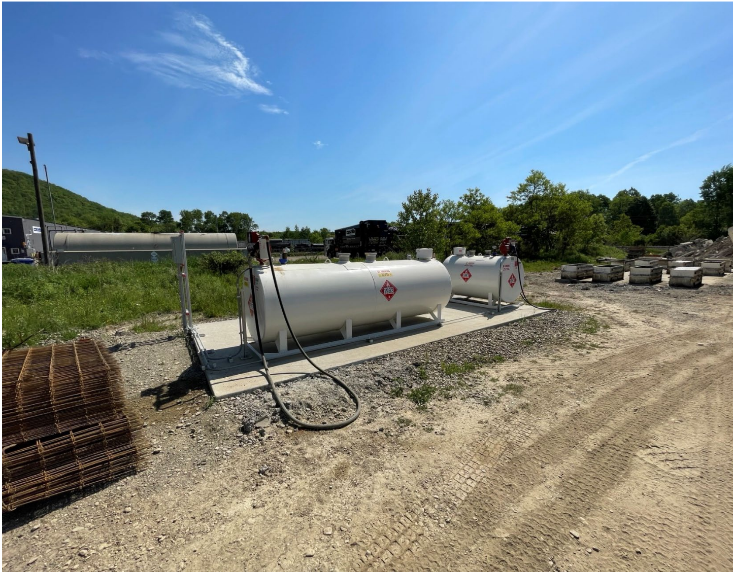
Additional concrete pad/fuel storage island.
