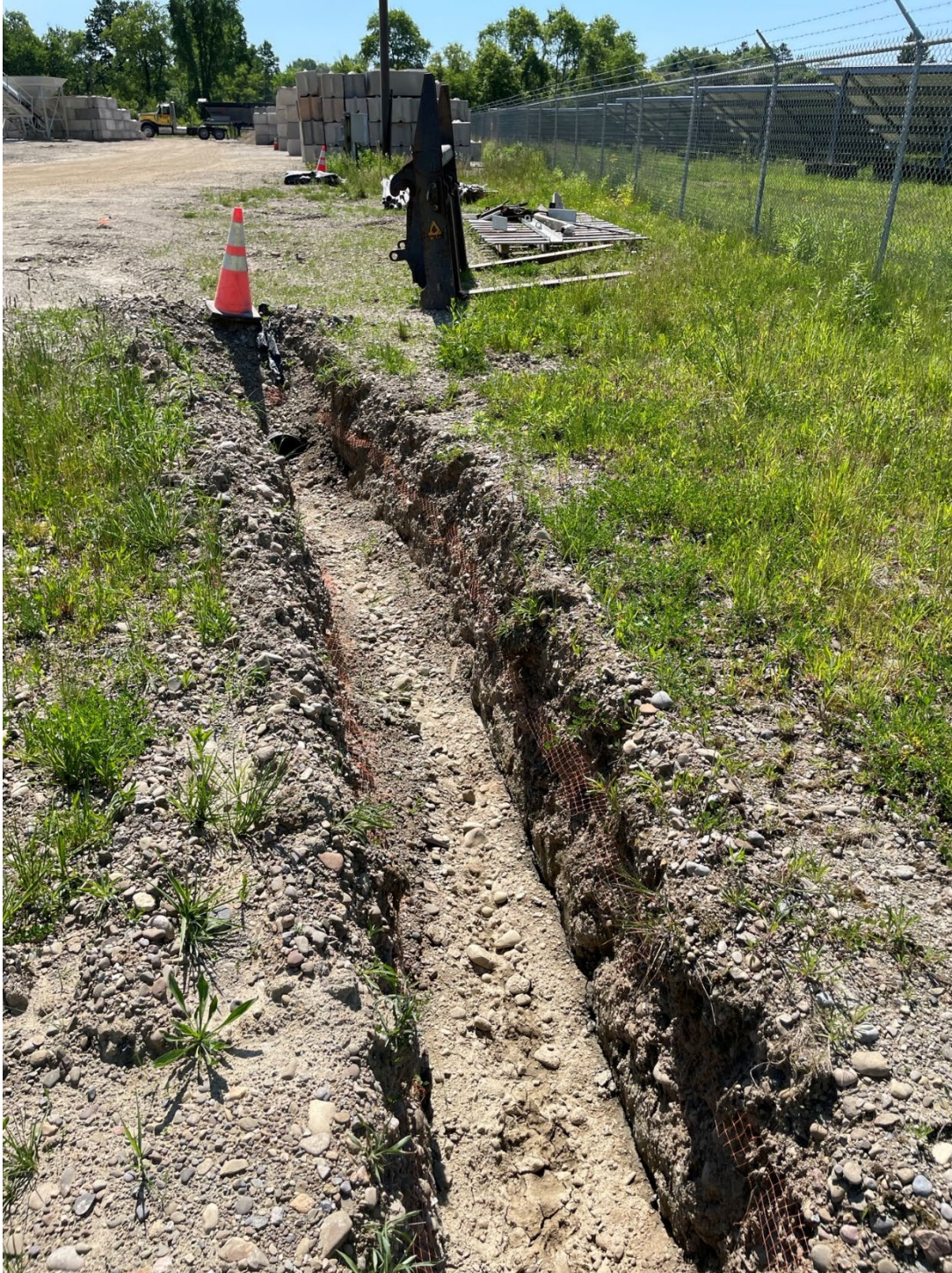
Onsite trench, view is facing southeast.
