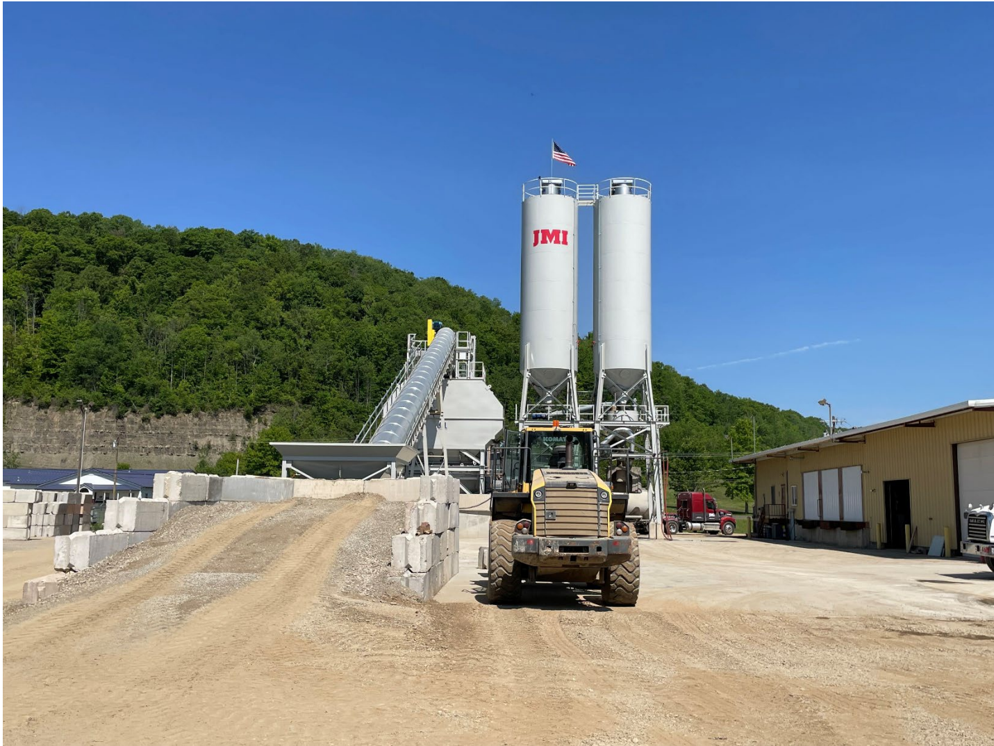
New facilities/southern end of building with possibly extended concrete pad.
