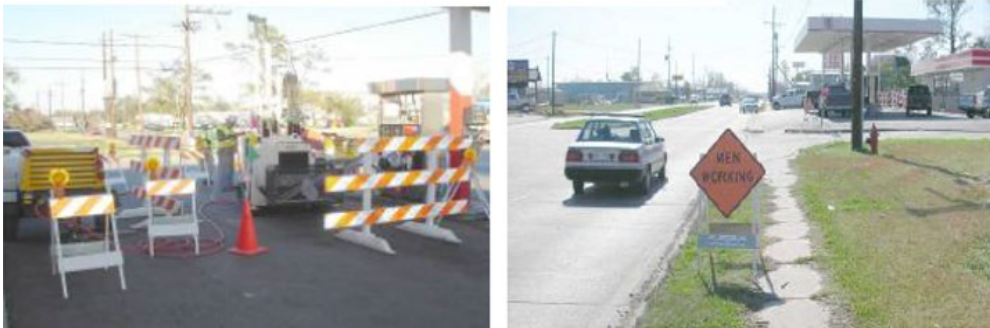
Examples of Level 2 Traffic Control
