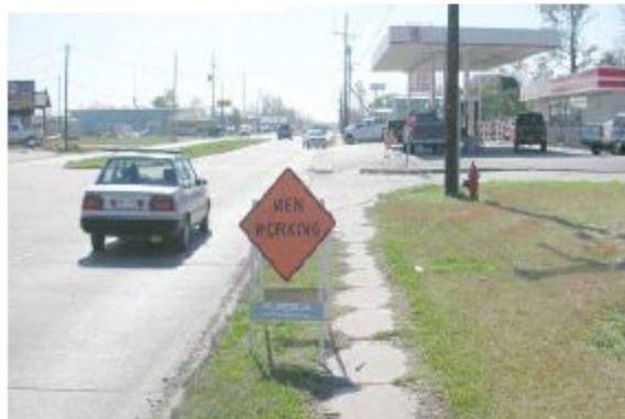
Example of Level 2 Traffic Control
