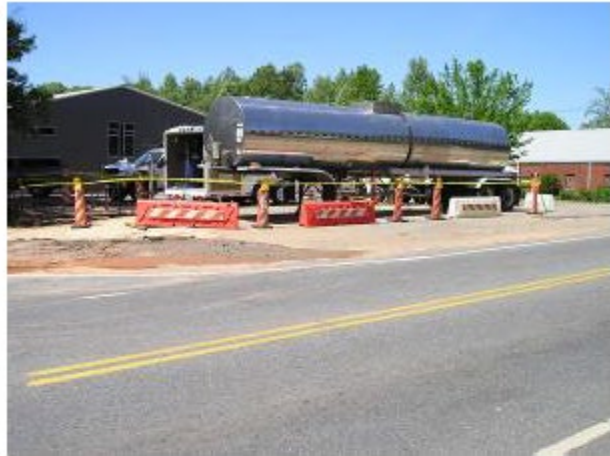
Example of Level 2 Traffic Control
