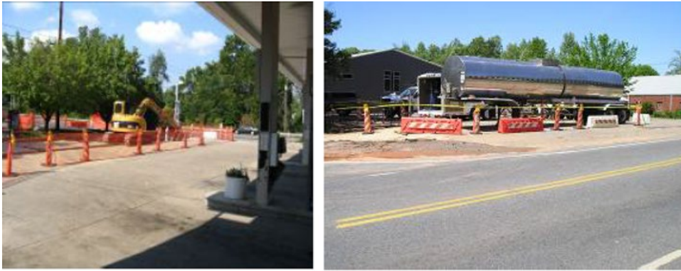
Examples of Level 2 Traffic Control
