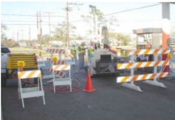
Example of Level 2 Traffic Control
