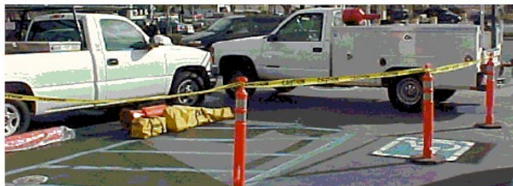
Example of Level 1 Traffic Control
