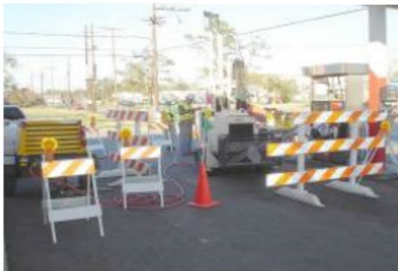
Example of Level 2 Traffic Control
