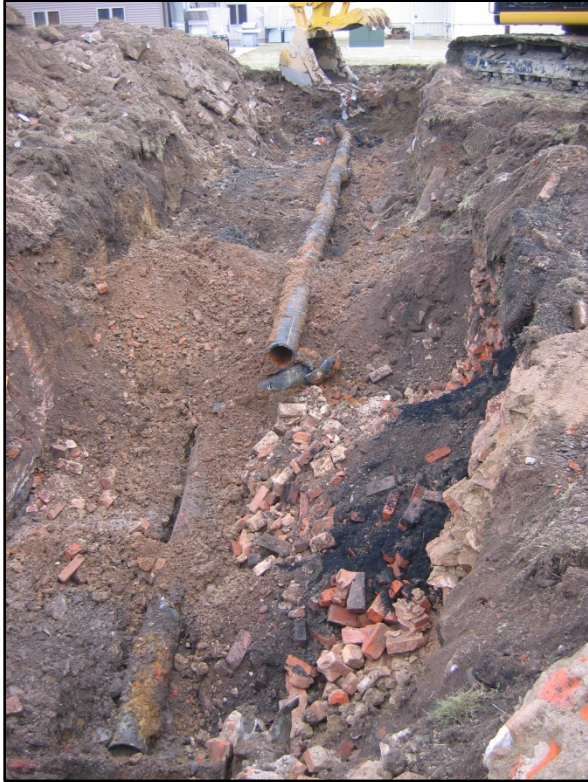
Photograph 3: SRS-Area-2 Pipe (looking east)
