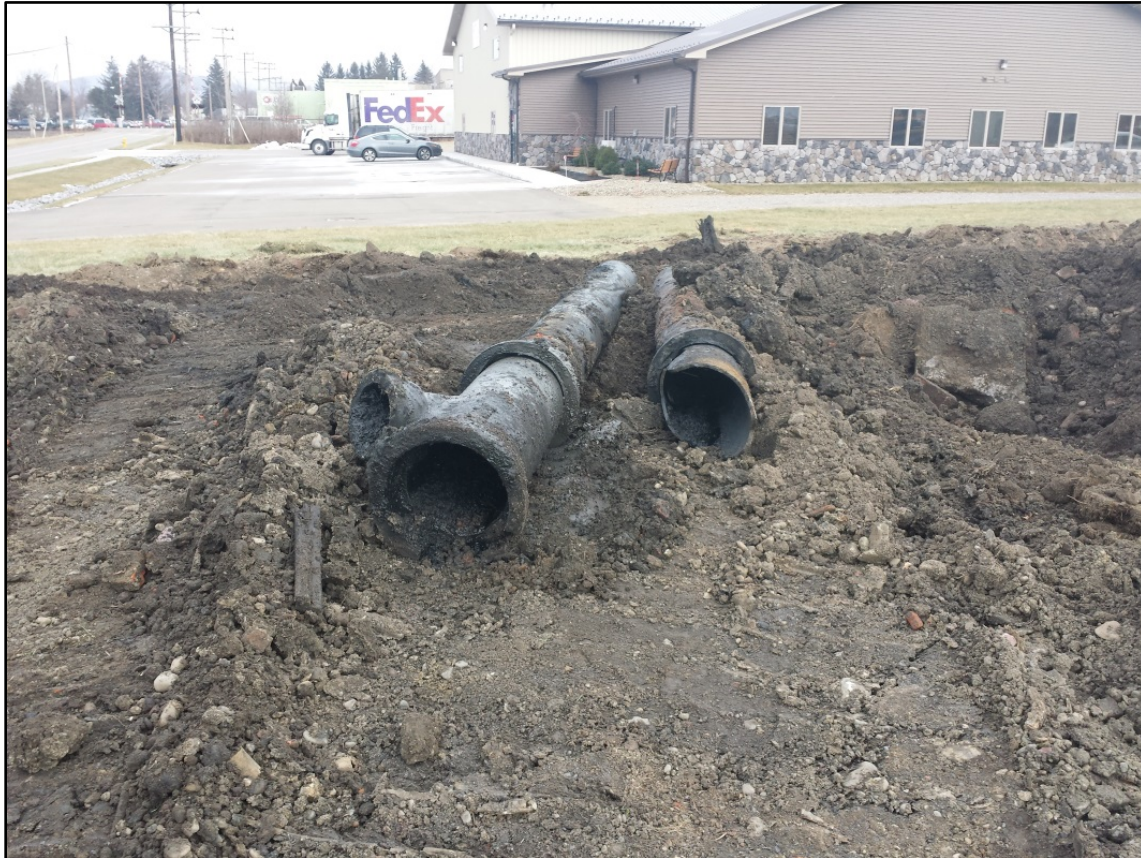
Photograph 2: SRS-Area-1 (deepest pipe – 12” pipe)
