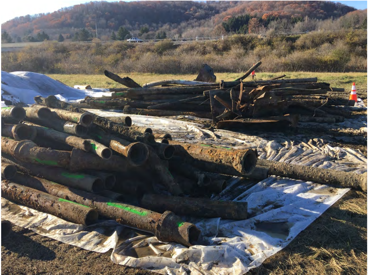
Photo 7: Excavated piping from 350 Franklin Street ready for off-Site disposal.
