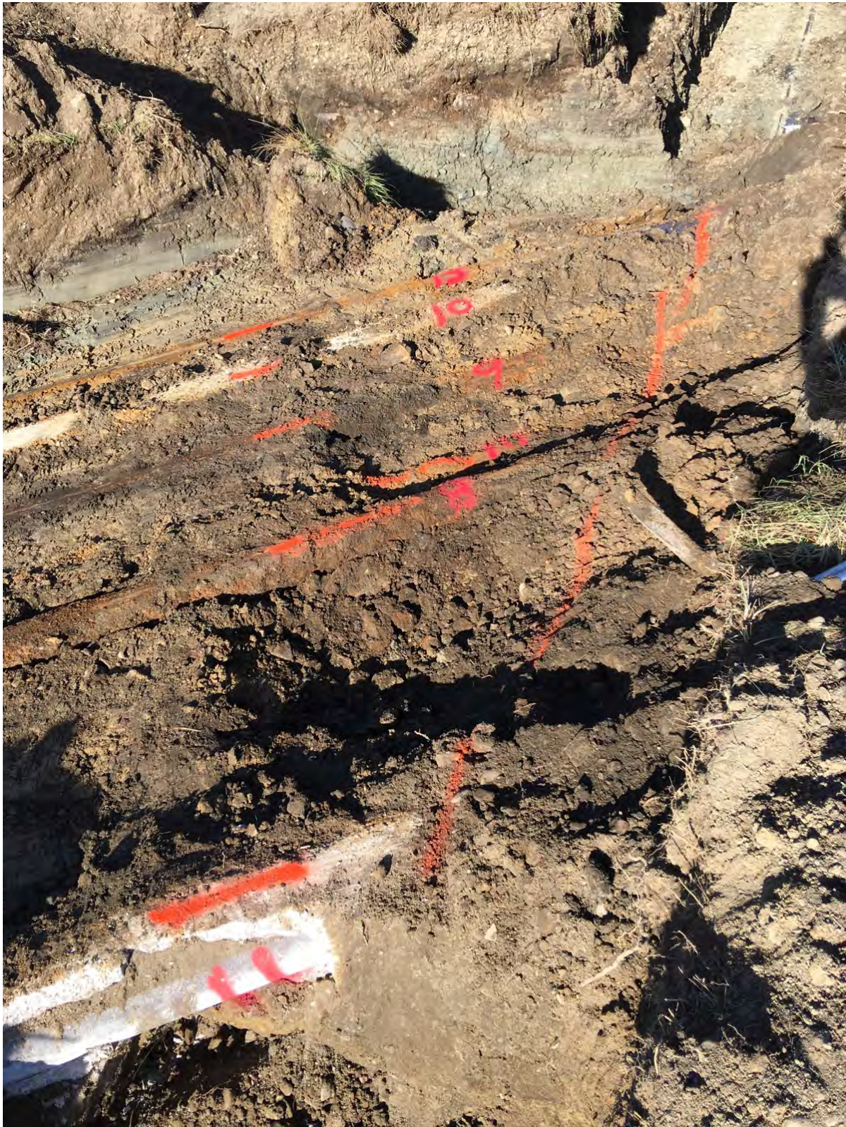
Photo 6: Excavation Zone 3 – 6 pipe cluster encountered at approximately 5 ft bgs (looking North).
