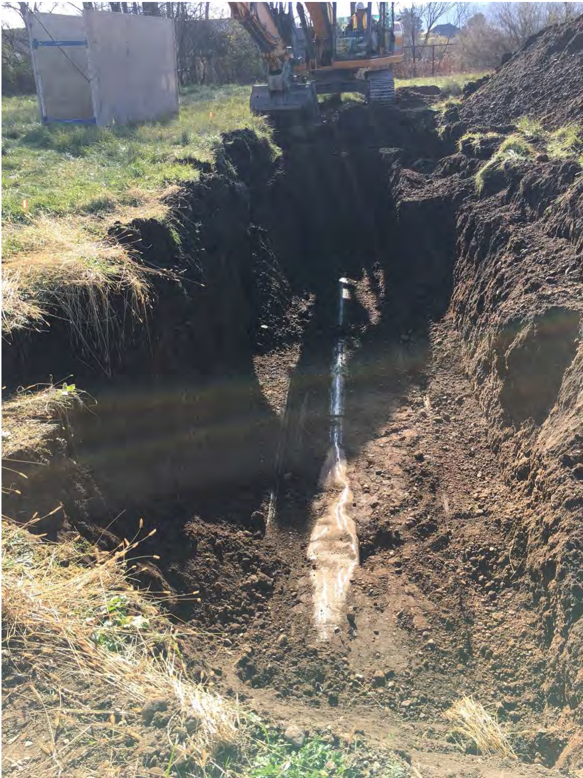
Photo 3: Excavation Zone 5 - 20" pipe encountered approximately 6 ft bgs (looking South).
