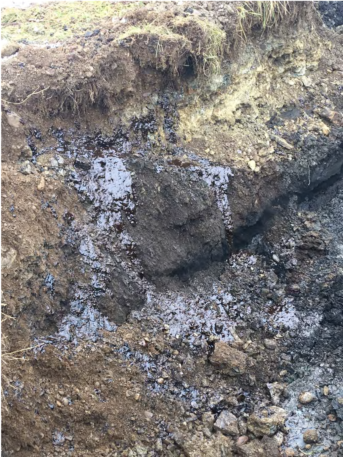
Photo 8: Excavation Zone 1 – Suspected GCM on sidewall encountered at approximately 5 ft bgs.
