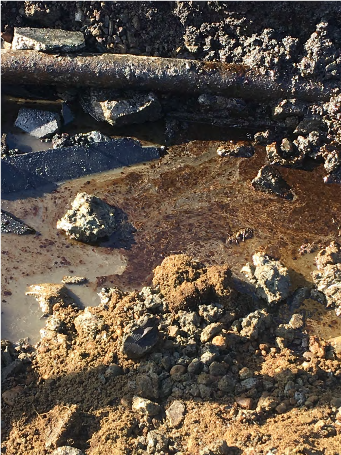
Photo 9: Excavation Zone 1 – Suspected GCM encountered approximately 5 ft bgs near....
