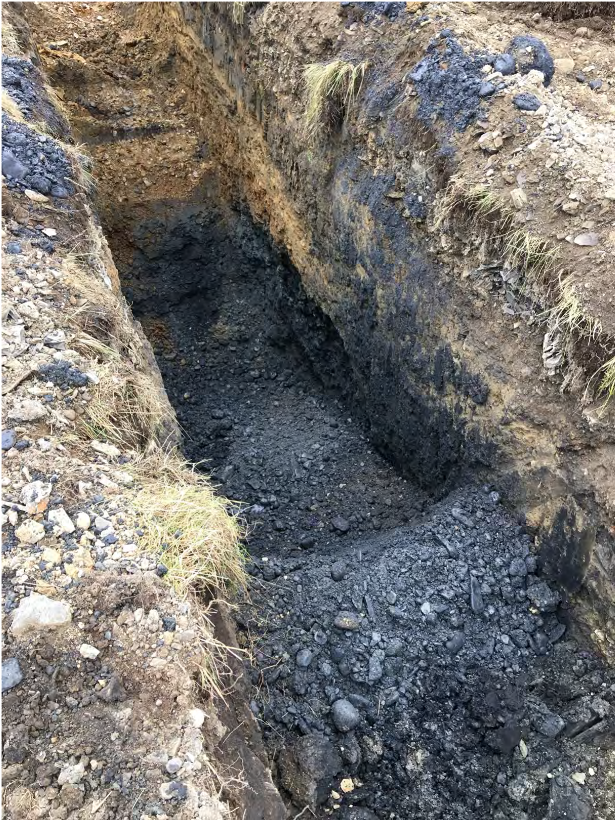
Photo 2: Excavation Zone 1 – suspected GCM encountered from 6-12 ft bgs.
