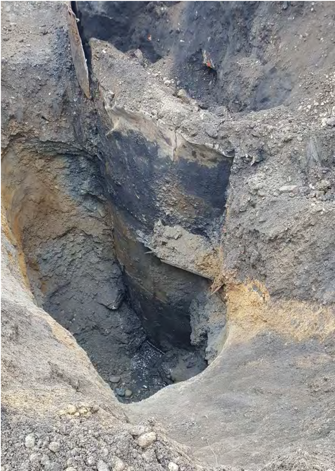
Photo 4: Excavation during investigation of Structure 2; bottom of structure and clay confining layer encountered at approximately 22 ft bgs.
