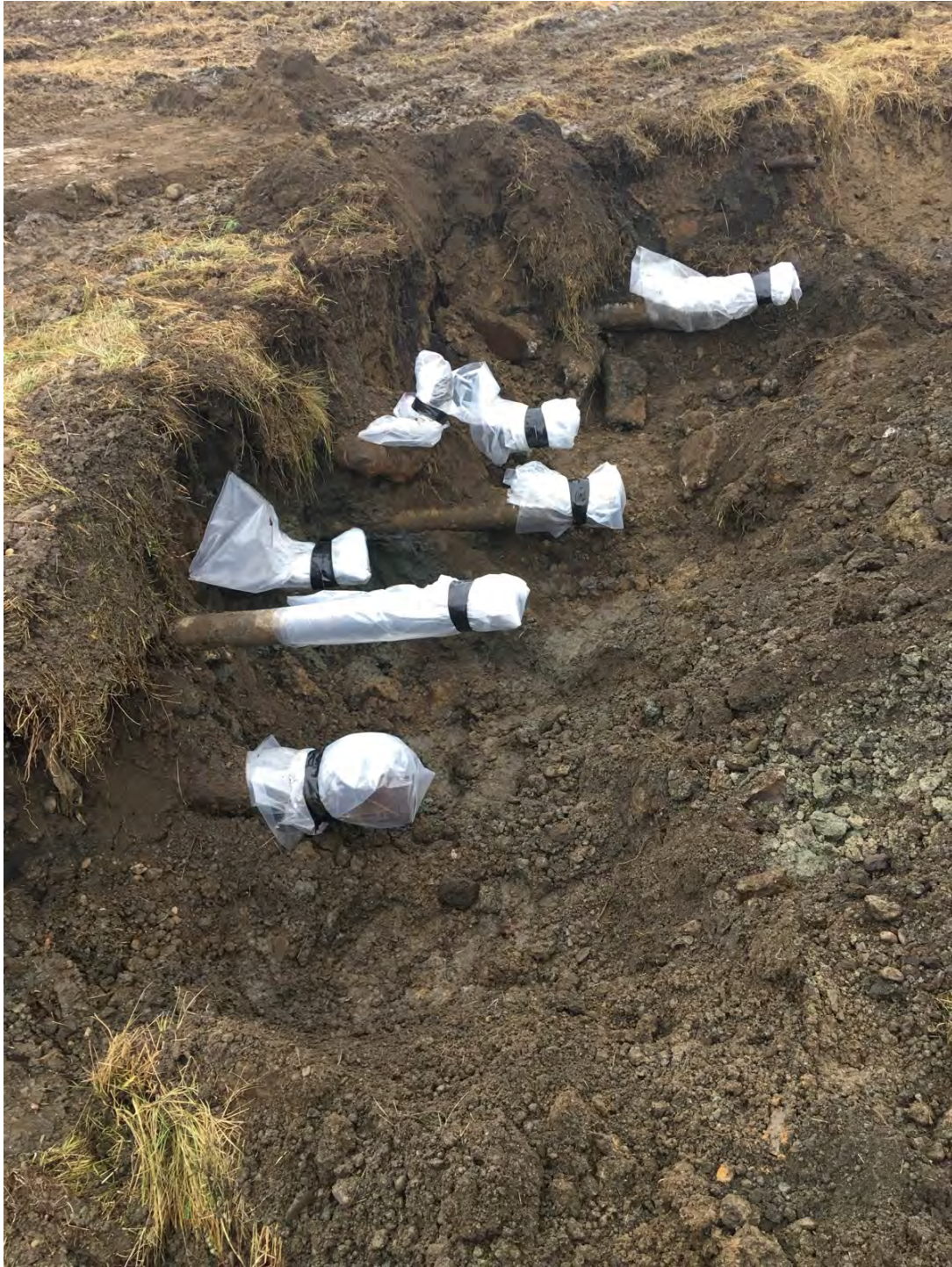
Photo 10: Excavation Zone 3 – Pipe capping activities.
